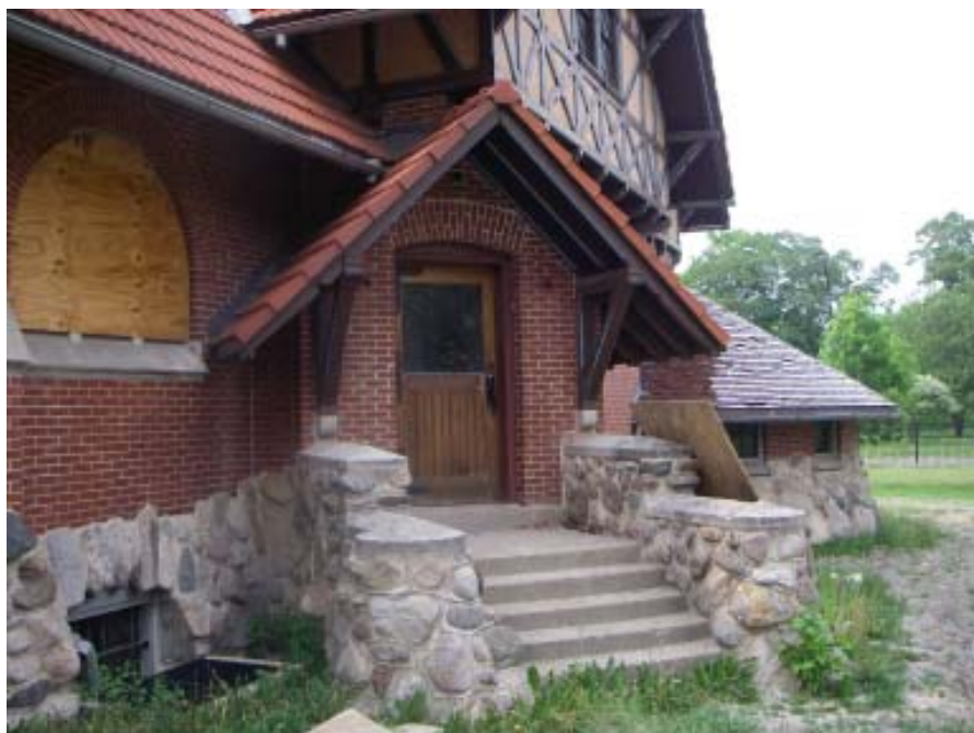
Bottom: The entrance to the northeast pavilion has an oversized roof-covered porch with rusticated field stone banisters.
