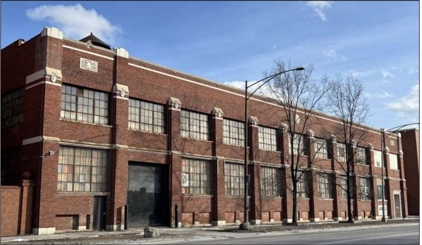
Western Boulevard Industrial Corridor, 4425 S. Western Boulevard, Grinnell Co., 1916, Argyle E. Robinson. Photo credit: Debbie Mercer
