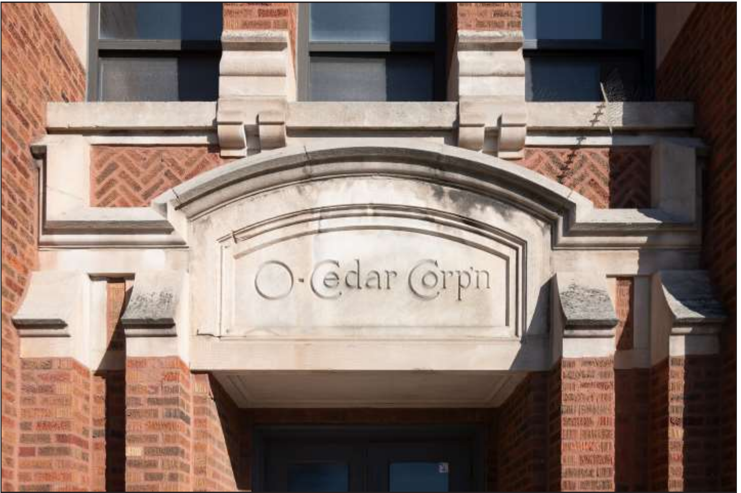
Entry details, Western Boulevard Industrial Corridor, 4501 S. Western Boulevard, 555 International / O-Cedar Corporation, 1920, Davidson & Weiss. Photo credit: Serhii Chucky / Esto
