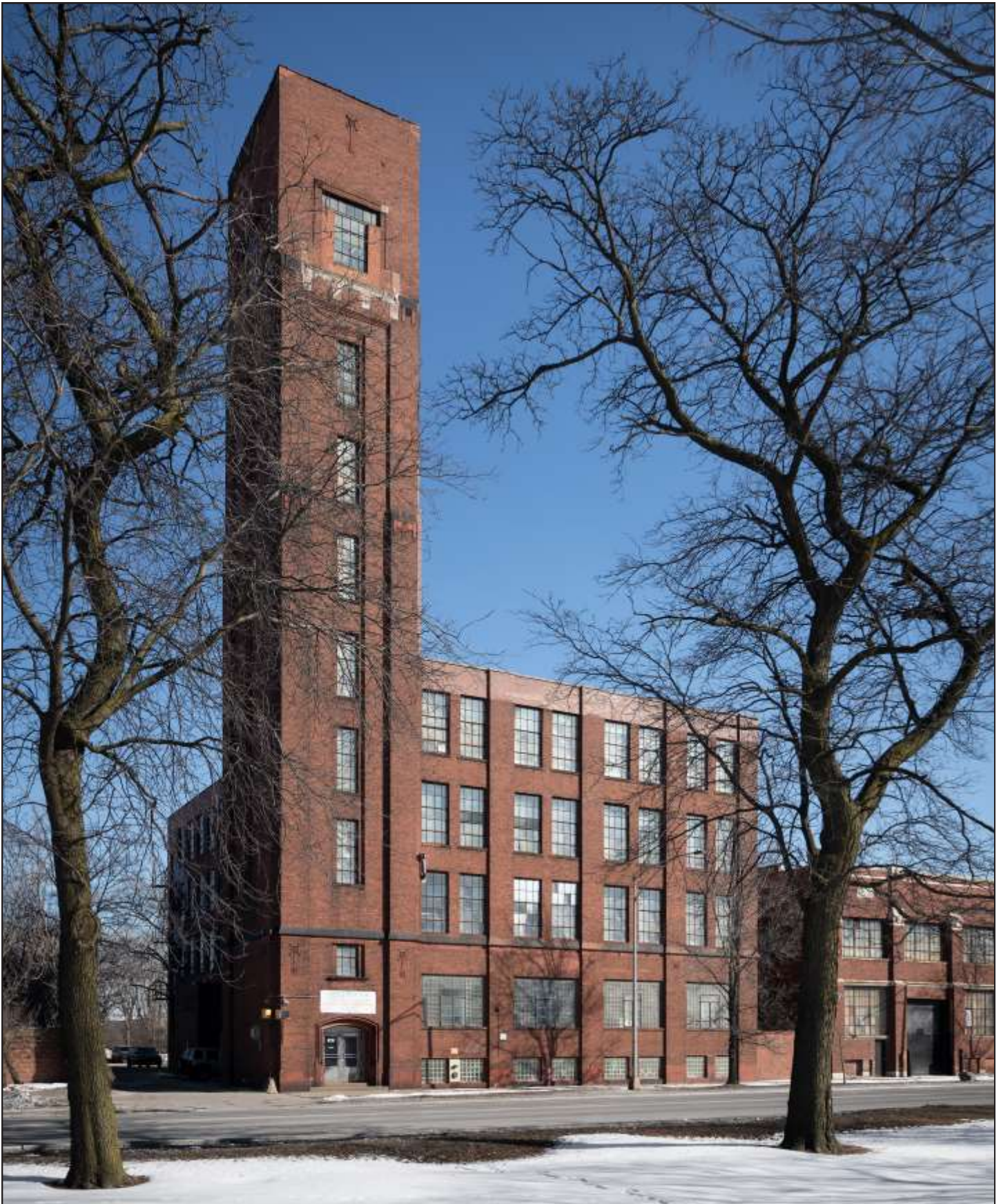
Western Boulevard Industrial Corridor, 4401 S. Western Boulevard, Wheatland Tube / Cold Parts, 1914, Samuel Scott Joy. Photo credit: Serhii Chucky / Esto
