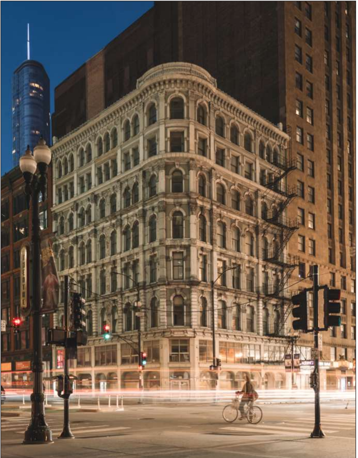
Evening view of the Delaware Building, 1872-1874, Wheelock & Thomas, with 1889 addition by Julius Huber, 36 W. Randolph Street. Photo credit: Lily Ma, Numi Studio
