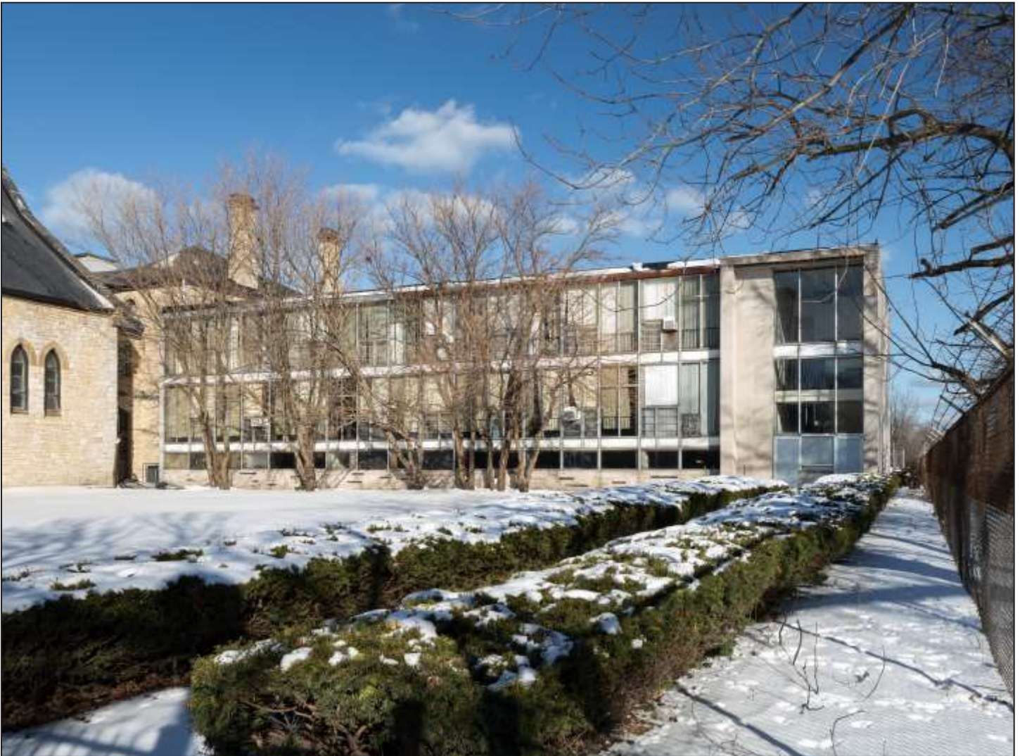
Olivet Baptist Church School, 1962, McKissack & McKissack, 3125 S. King Drive. Photo credit: Serhii Chrukky / Esto
