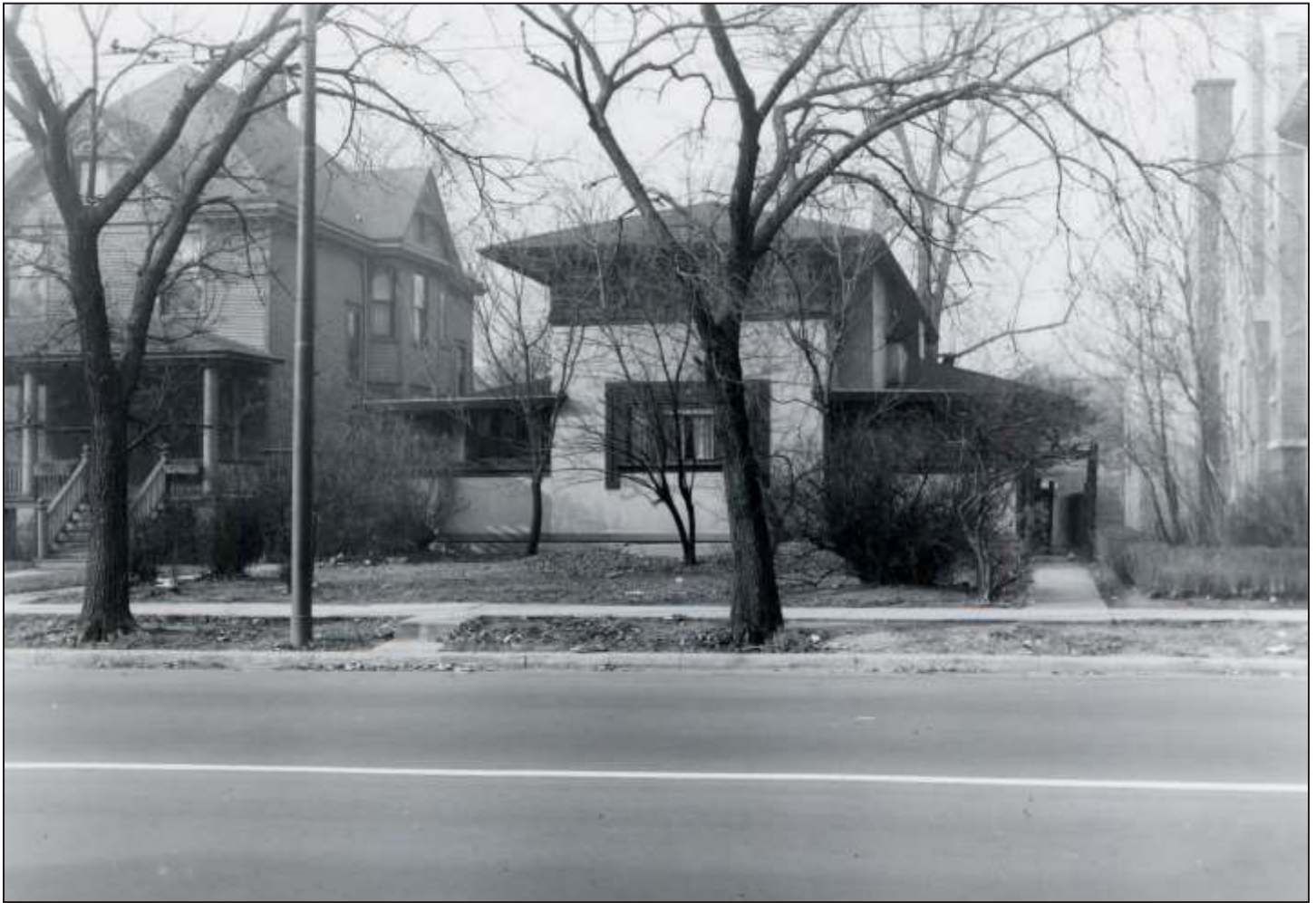
Views of principal façade on Central Avenue, Joseph Jacob (J.J.) Walser House, 1903, Frank Lloyd Wright, 42 N. Central Avenue. Photo courtesy of the Gilman Lane Photograph Collection, Oak Park Public Library Special Collections
