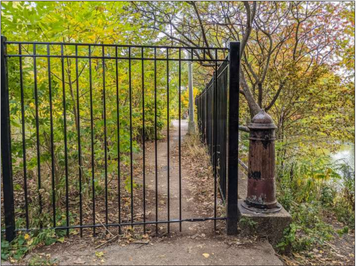
Current conditions Clarence Darrow Memorial Bridge / Columbia Bridge, 1880, Burnham & Root, 1766 Columbia Drive. Photo credit: Eric Allix Rogers
