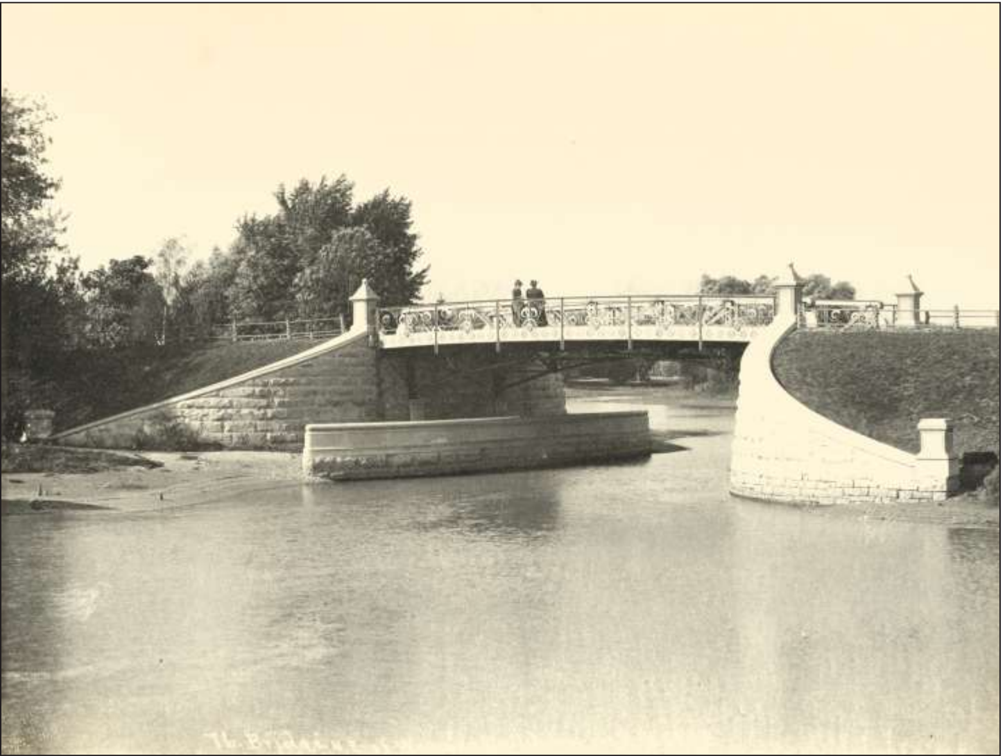
"The Bridge northeast of Woman's Building, construction stage, October 16, 1891." This view, looking northwest, shows the original configuration of the bridge trusses and superstructure, as well as the limestone abutments and retaining wall along the water. Note the piers with finials at the base and top of the east and west retaining walls. Photo credit: C. D. Arnold, Chicago Public Library, Special Collections, C. D. Arnold Photographic Collection, Box 19, Volume XI, Plate 58
