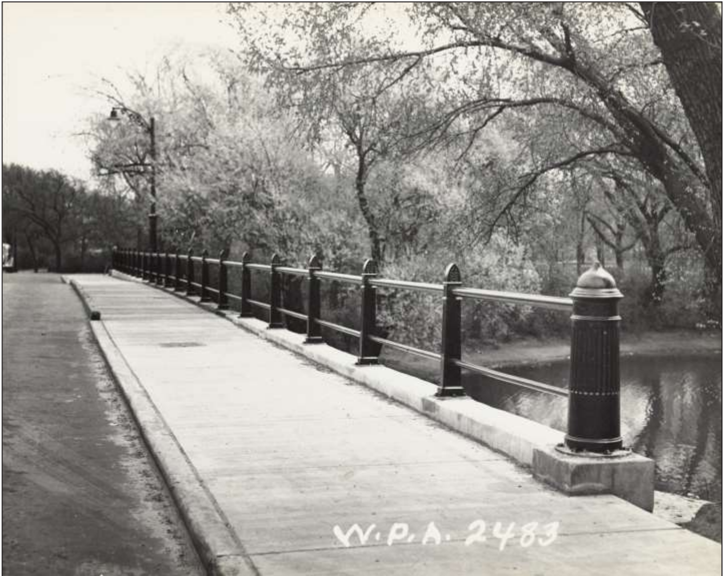
View of the Clarence Darrow Memorial Bridge in Jackson Park, Chicago, Illinois. View of sidewalk, curb, and railing, circa 1937. Photo credit: Chicago Park District, Works Progress Administration photograph 2483, Chicago Public Library, Special Collections, Chicago Park District Archives, Photographs: Jackson Park (0019) Features, Box 47, Folder 8, Photograph 4
