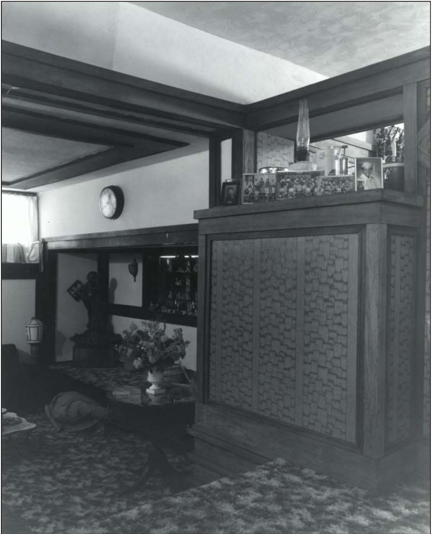
View of reception room and entry, Joseph Jacob (J.J.) Walser Residence, Chicago, Illinois, 1903, Frank Lloyd Wright, 42 N. Central Avenue. Photo credit: John Vinci, John Vinci Papers, Ryerson and Ryerson and Burnham Art and Architecture Archives, The Art Institute of Chicago. Digital File#200704_251120-007
