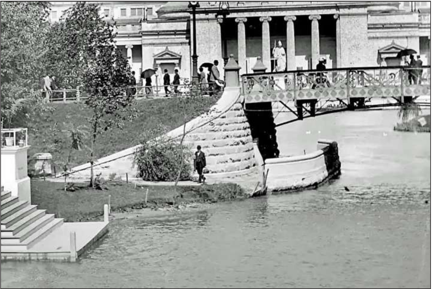
View of the west end of the bridge and the west abutment, looking north, 1893. Clarence Darrow Memorial Bridge / Columbia Bridge, 1880, Burnham & Root, 1766 Columbia Drive in Jackson Park, Chicago. Photo credit: Photo credit: Tim Samuelson personal collection
