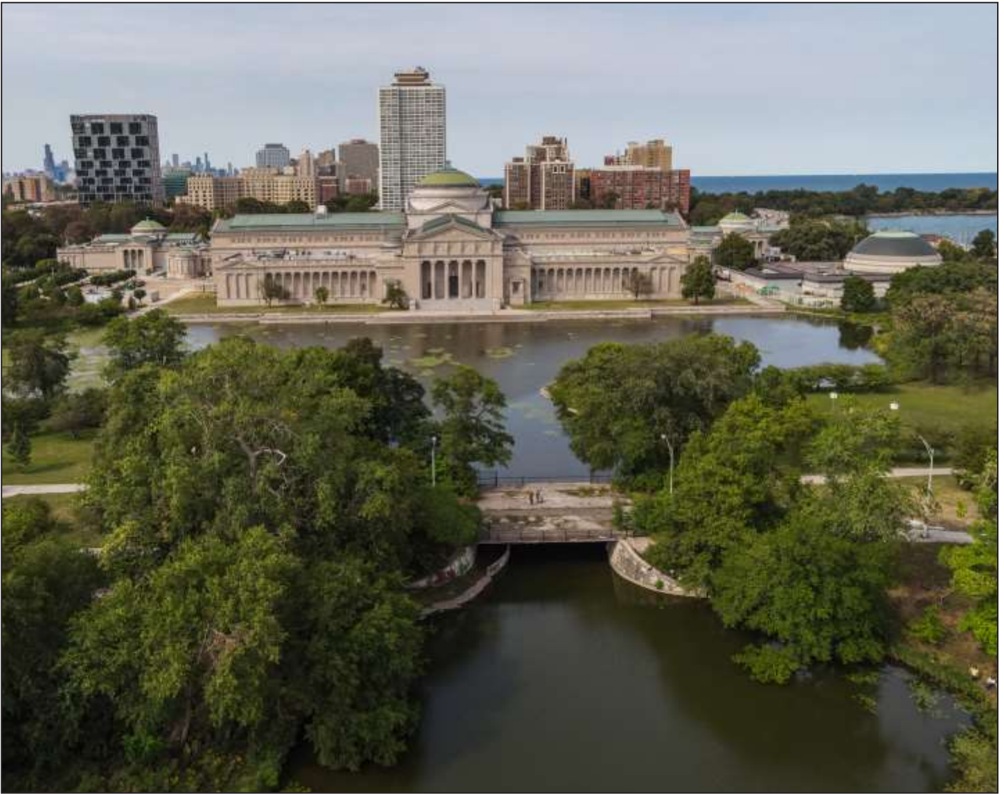
Clarence Darrow Memorial Bridge / Columbia Bridge, 1880, Burnham & Root, 1766 Columbia Drive. Photo credit: Eric Allix Rogers
