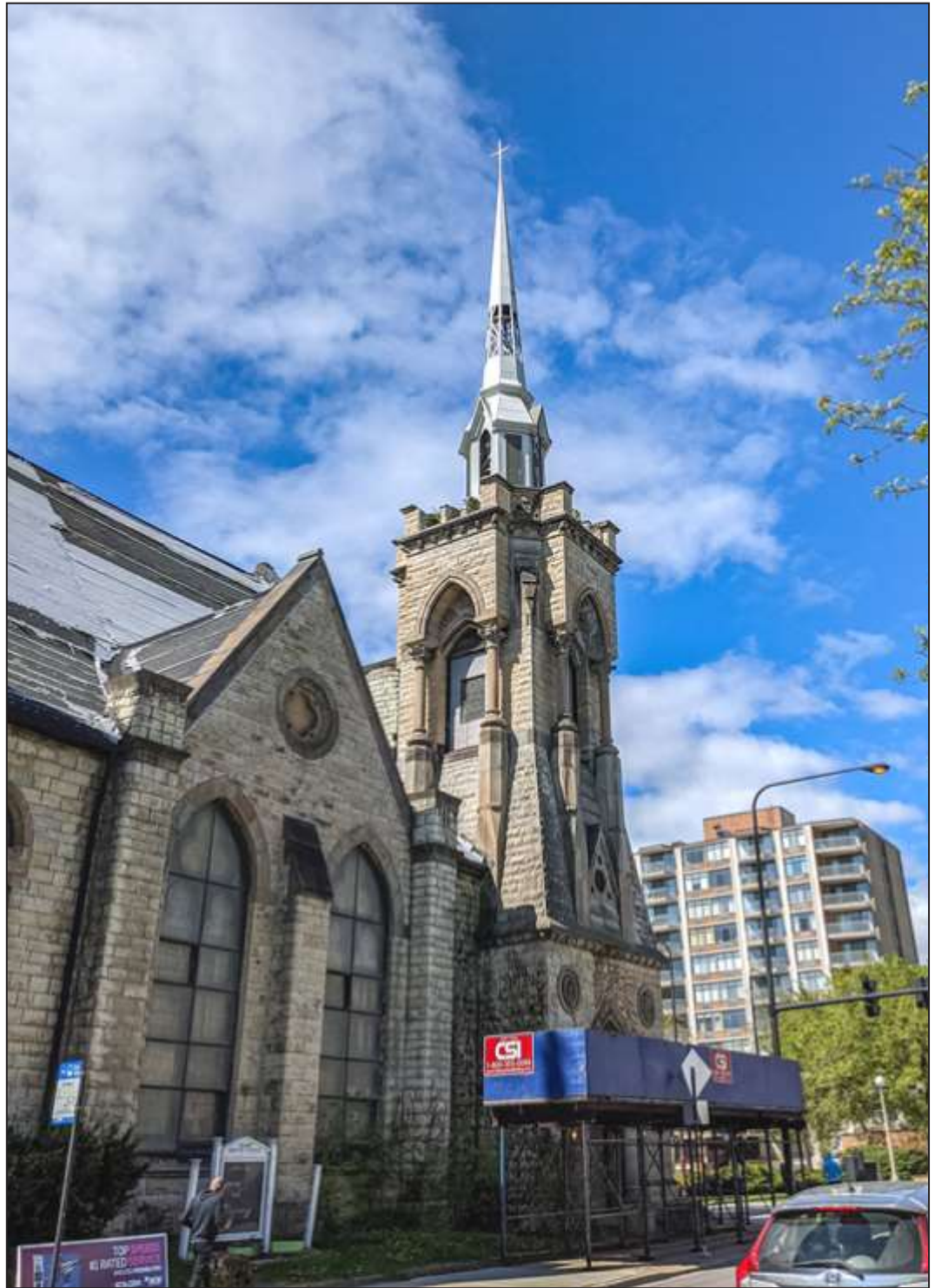
Partial view of 31st Street elevation with new replacement steeple, Olivet Baptist Church / First Baptist Church of Chicago, 1876, Wilcox and Miller, 3101 S. King Drive. Photo credit: Eric Allix Rogers
