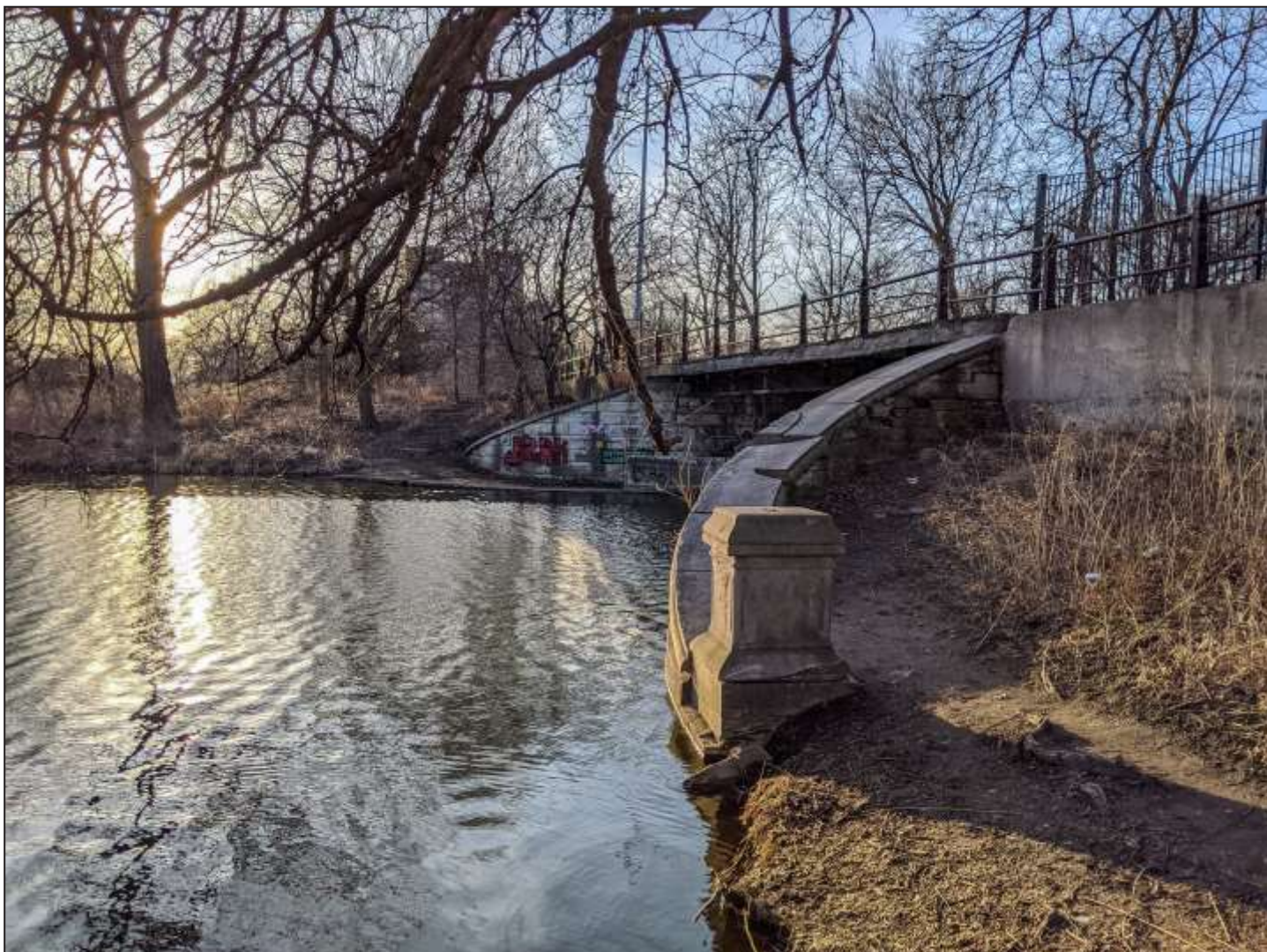
Clarence Darrow Memorial Bridge / Columbia Bridge, 1880, Burnham & Root, 1766 Columbia Drive. Photo credit: Eric Allix Rogers
