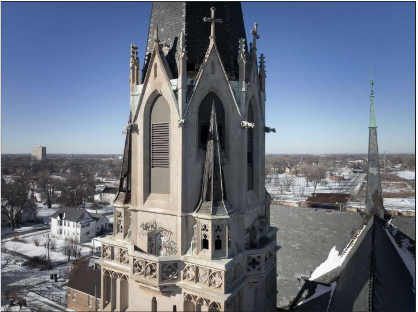
Tower detail, St. Martin de Tours / St. Martin de Porres, 1895, Henry J. Schlacks, 5848 S. Princeton Avenue. Photo Credit: Serhii Chrucky / Esto
