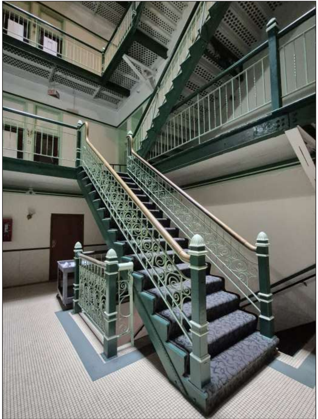
Detail of second floor atrium and stairs, The Delaware Building, Atrium 1872-1874, Wheelock & Thomas, with 1889 addition by Julius Huber, 36 W. Randolph Street. Photo credit: Ward Miller
