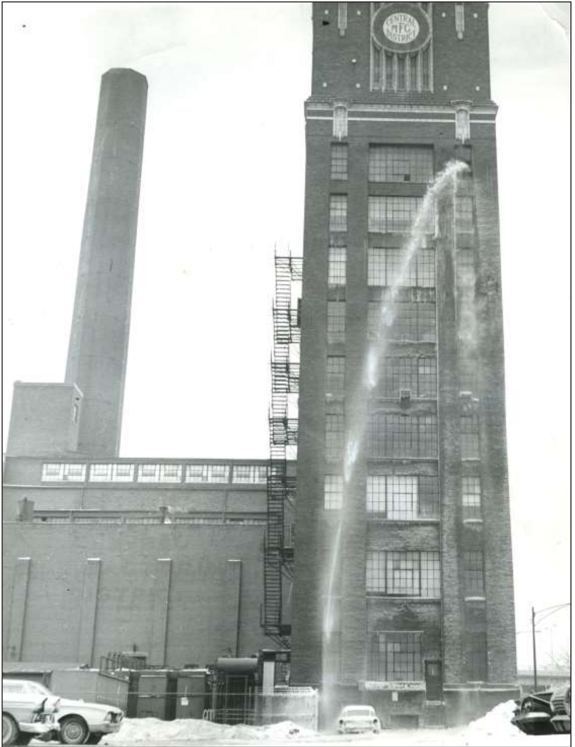
'Niagara' on South Side: Water pours from ninth floor of the Central Manufacturing tower at Pershing and Damen. The "Niagara" resulted from a break in a fill pipe leading to the automatic sprinkler system. It took more than an hour to turn off the water valve because of extreme pressure. Eight floors were flooded." Central Manufacturing District Clock Tower Building, 1917, Samuel Scott Joy, 2000 W. Pershing Road. Photo credit: Don Casper, Chicago Sun-Times, January 26, 1963 / Preservation Chicago Photo Collection
