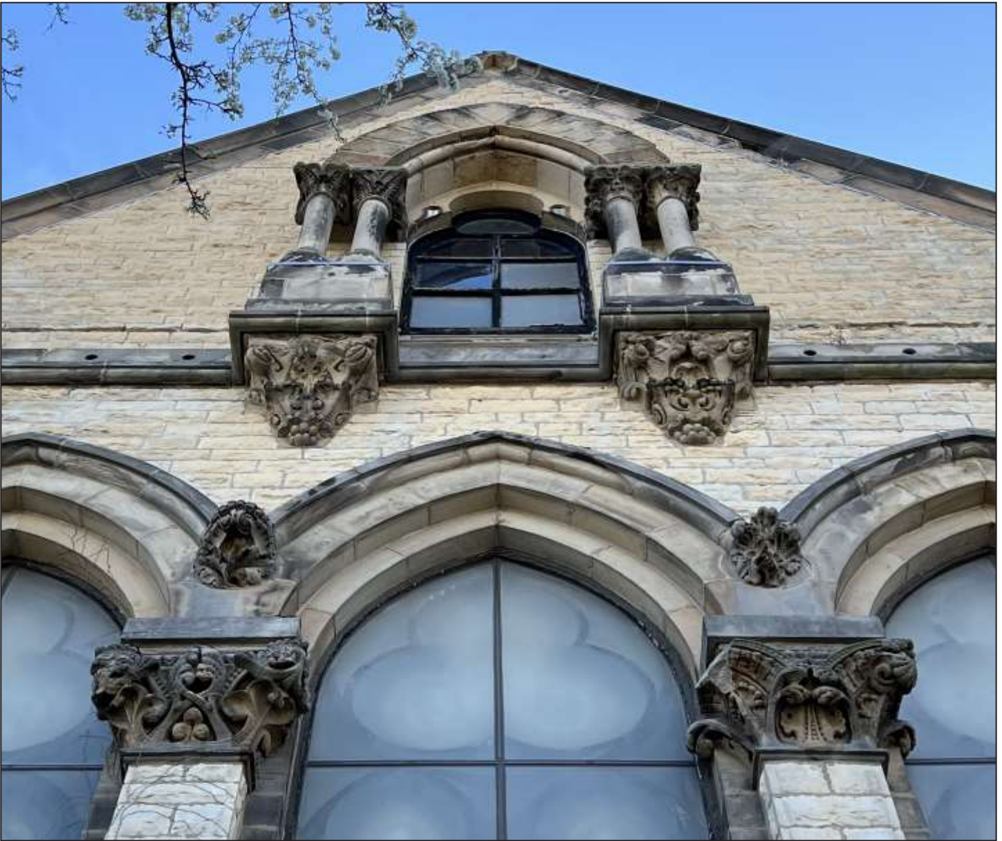
Detail of King Drive upper façade, Olivet Baptist Church / First Baptist Church of Chicago, 1876, Wilcox and Miller, 3101 S. King Drive.
