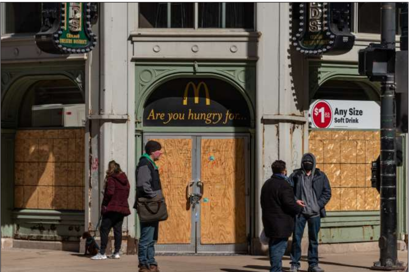
Corner storefront, Delaware Building, 1872-1874, Wheelock & Thomas, 36 W. Randolph Street. Photo credit: Eric Allix Rogers
