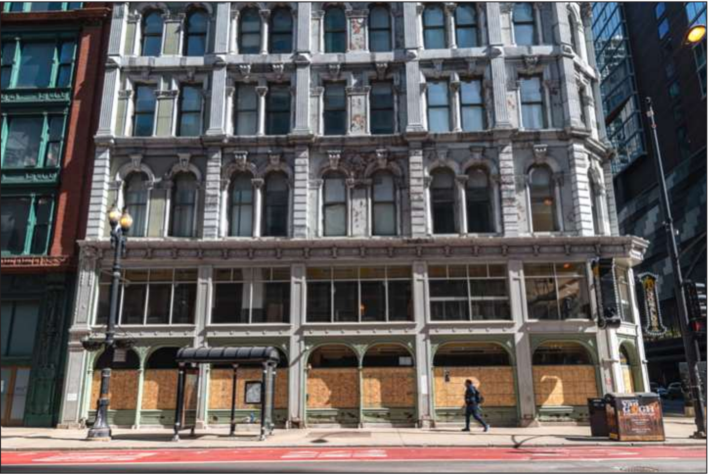
Lower floors of the Dearborn Street façade. The Delaware Building, 1872-1874, Wheelock & Thomas, with 1889 addition by Julius Huber, 36 W. Randolph Street. Photo credit: Eric Allix Rogers
