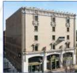
Werner Bros. Storage Chicago 7 2023 Adaptive Reuse
