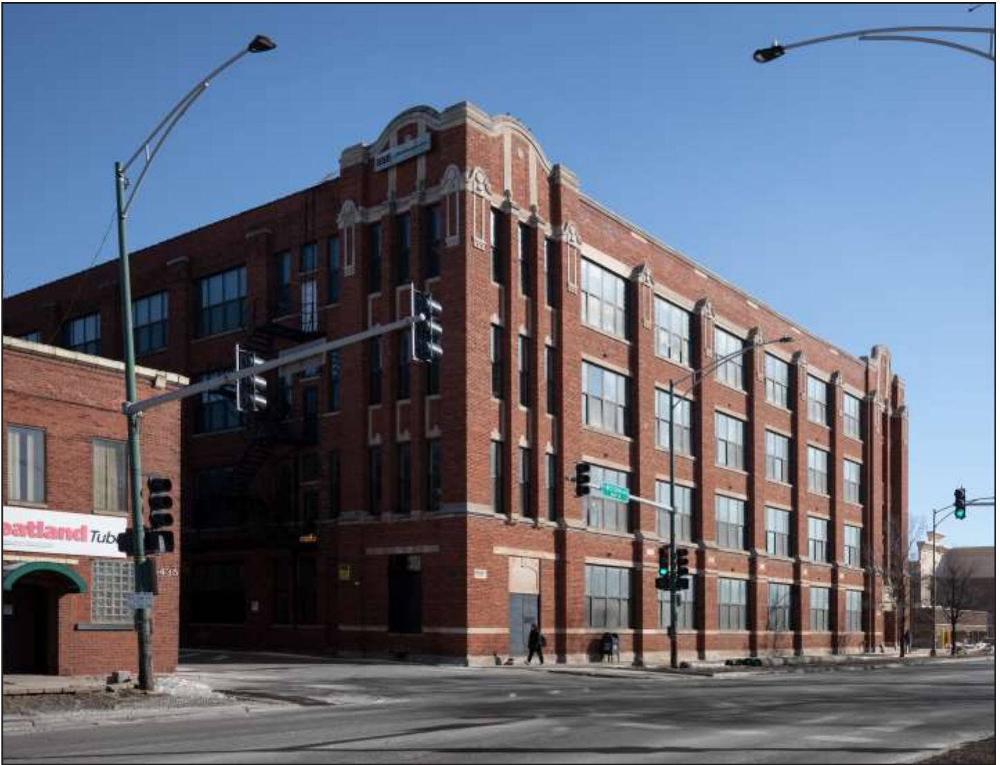
Western Boulevard Industrial Corridor, 4501 S. Western Boulevard, 555 International / O-Cedar Corporation, 1920, Davidson & Weiss. Photo credit: Serhii Chrucky / Esto
