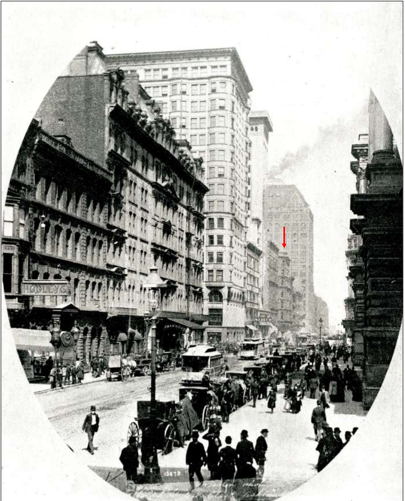
Randolph Street looking east from Hooley's Theatre, circa 1892, with the Delaware Building in the distance noted with a red arrow. All other buildings in the photograph have been lost to demolition, including the Borden Block and Schiller/Garrick Building by Adler & Sullivan, the Ashland Block by Burnham & Root, the Masonic Temple by Burnham & Root, and the Sherman House Hotel. Photo credit: Chicago and Its Makers, Paul Gilbert and Charles Lee Bryson, 1929, pg. 146 / Preservation Chicago Library Collection
