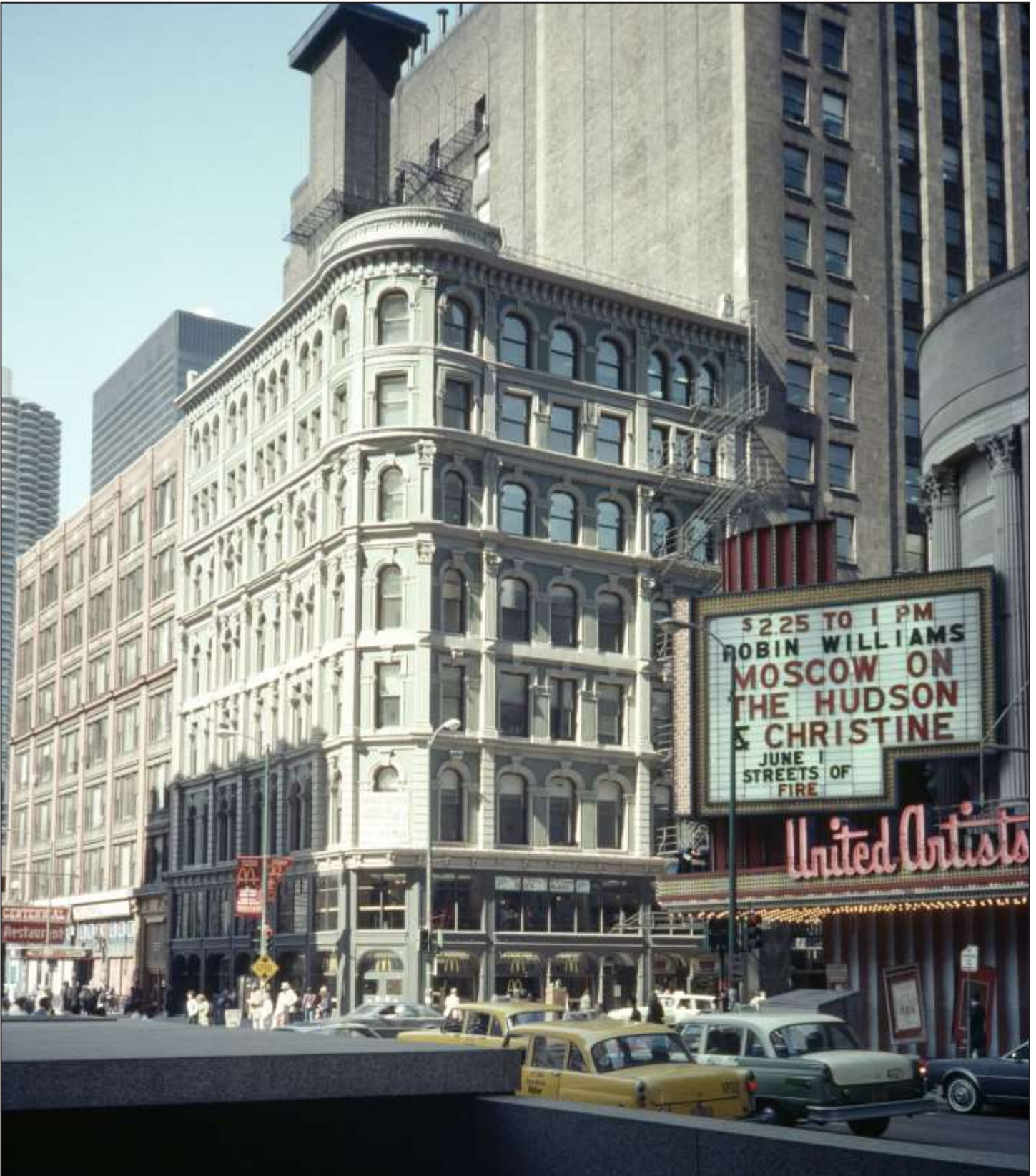
The Delaware Building, 1872-1874, Wheelock & Thomas, 36 W. Randolph Street, c. 1984. Photo credit: "Delaware Building, Chicago, IL," bruo01_02_kF, C. William Brubaker Digital Image collection, Special Collections and University Archives, University of Illinois at Chicago
