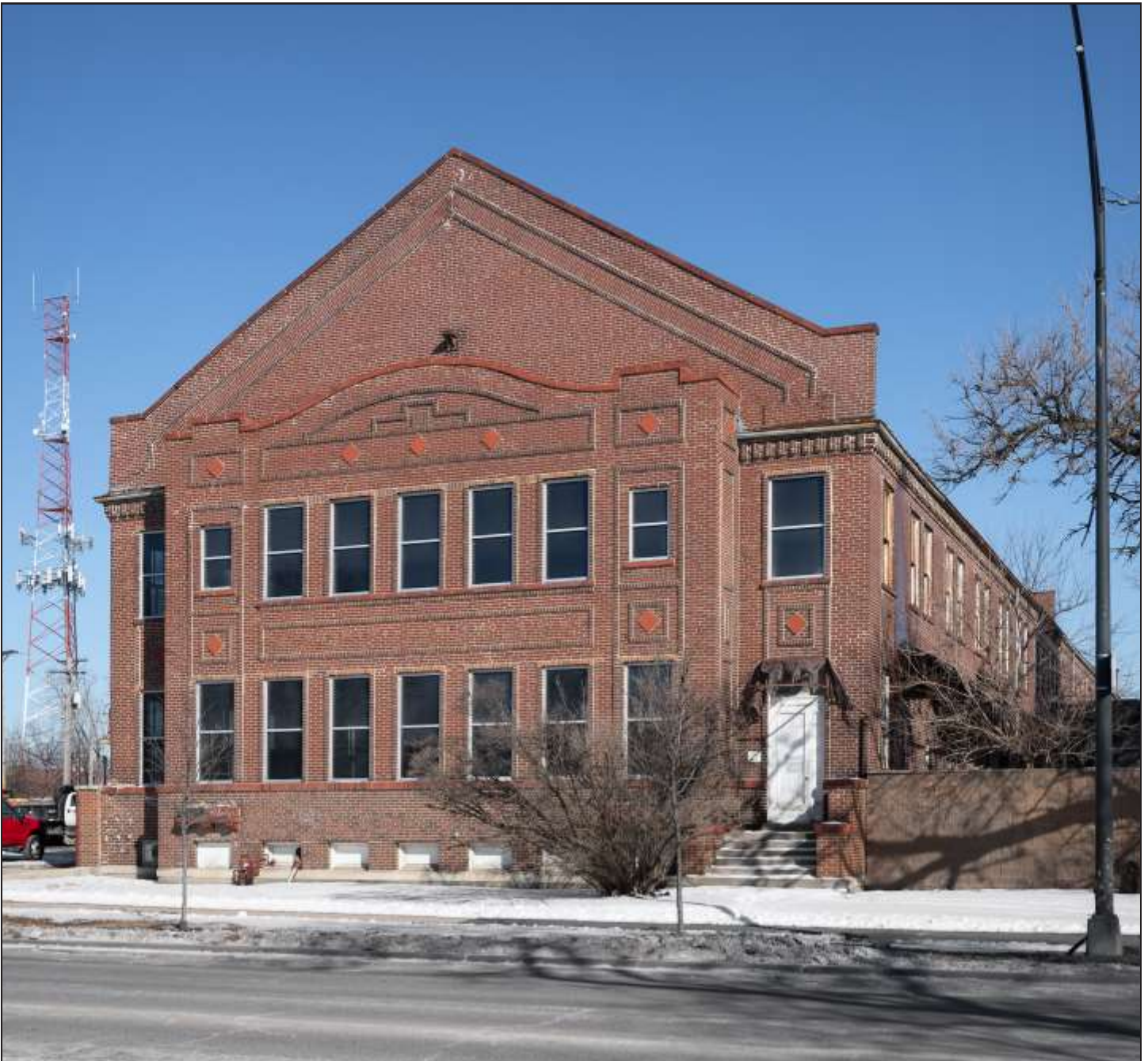
Western Boulevard Industrial Corridor, 4335 S. Western Boulevard, Kinsella Landscaping Building, 1916, Argyle E. Robinson. Photo credit: Serhii Chucky / Esto
