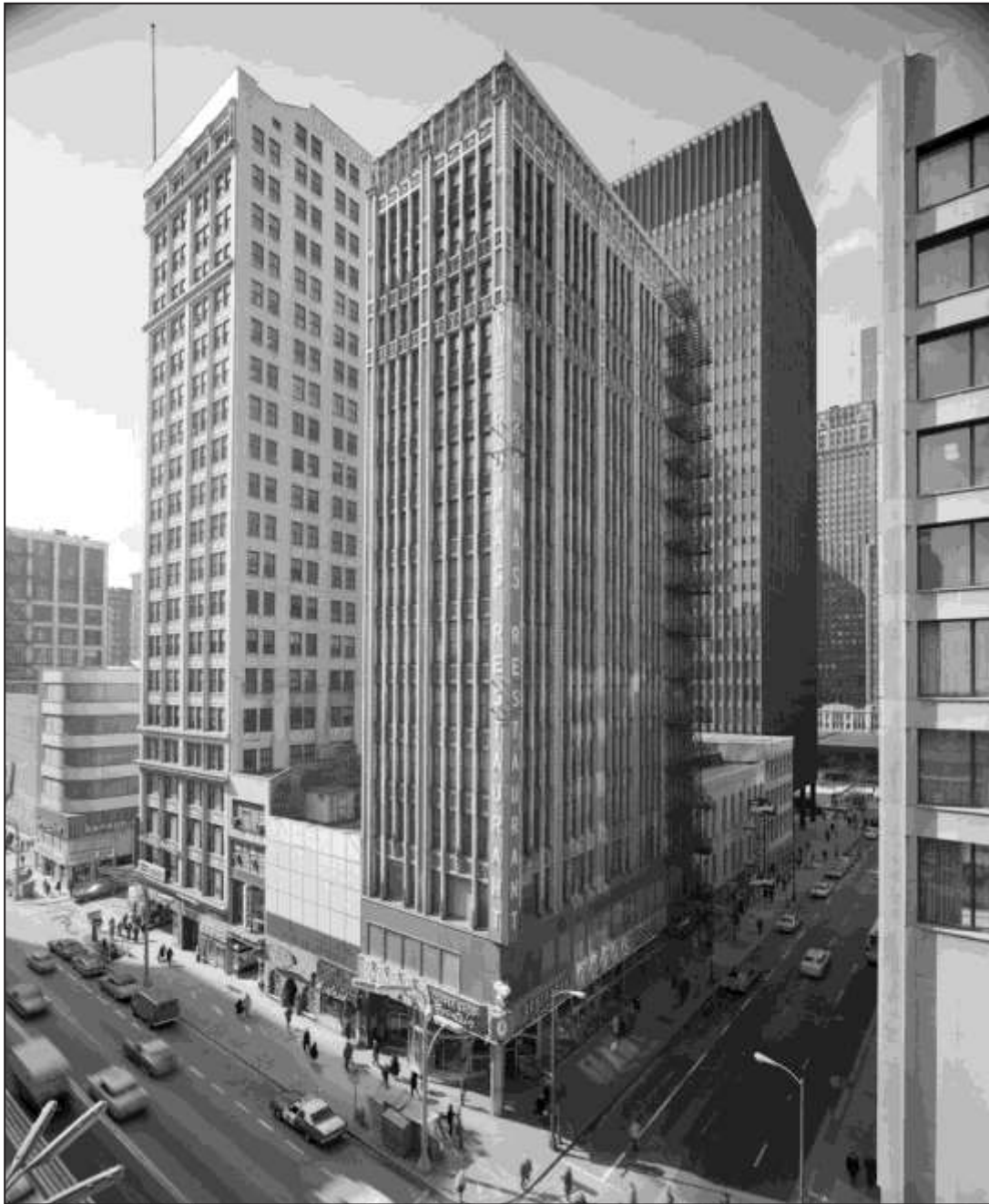
Exterior view of the Century and Consumers Buildings at 202 and 220 South State Street, Chicago, Illinois, c.1975. Photo credit: Hedrich-Blessing Collection, Chicago History Museum, HB-39113
