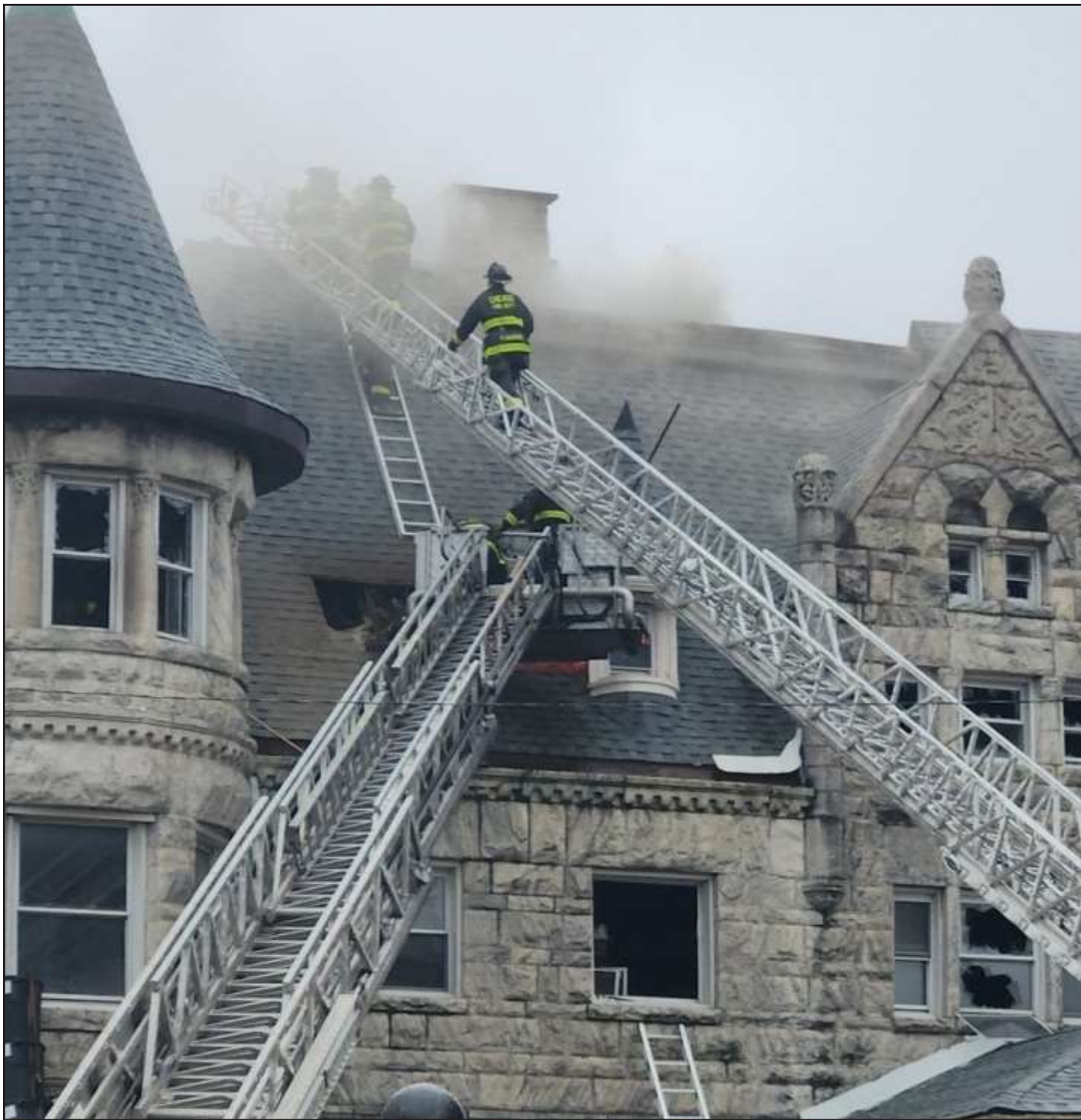
December 3, 2023 fire at Swift-Morris Mansion, 1892, Willett & Pashley, 4500 S. Michigan Avenue. Photo credit: Chicago Fire Department Media
