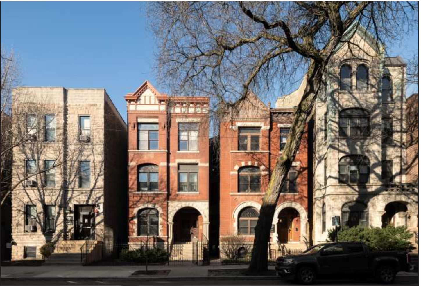
Sheffield-Belden Group, northwest corner of Sheffield and Belden Avenues. Freestanding townhouses, 2314 and 2316 N. Sheffield, John Morrell and others, 1890-1893. Photo Credit: Serhii Chrukly / Esto
