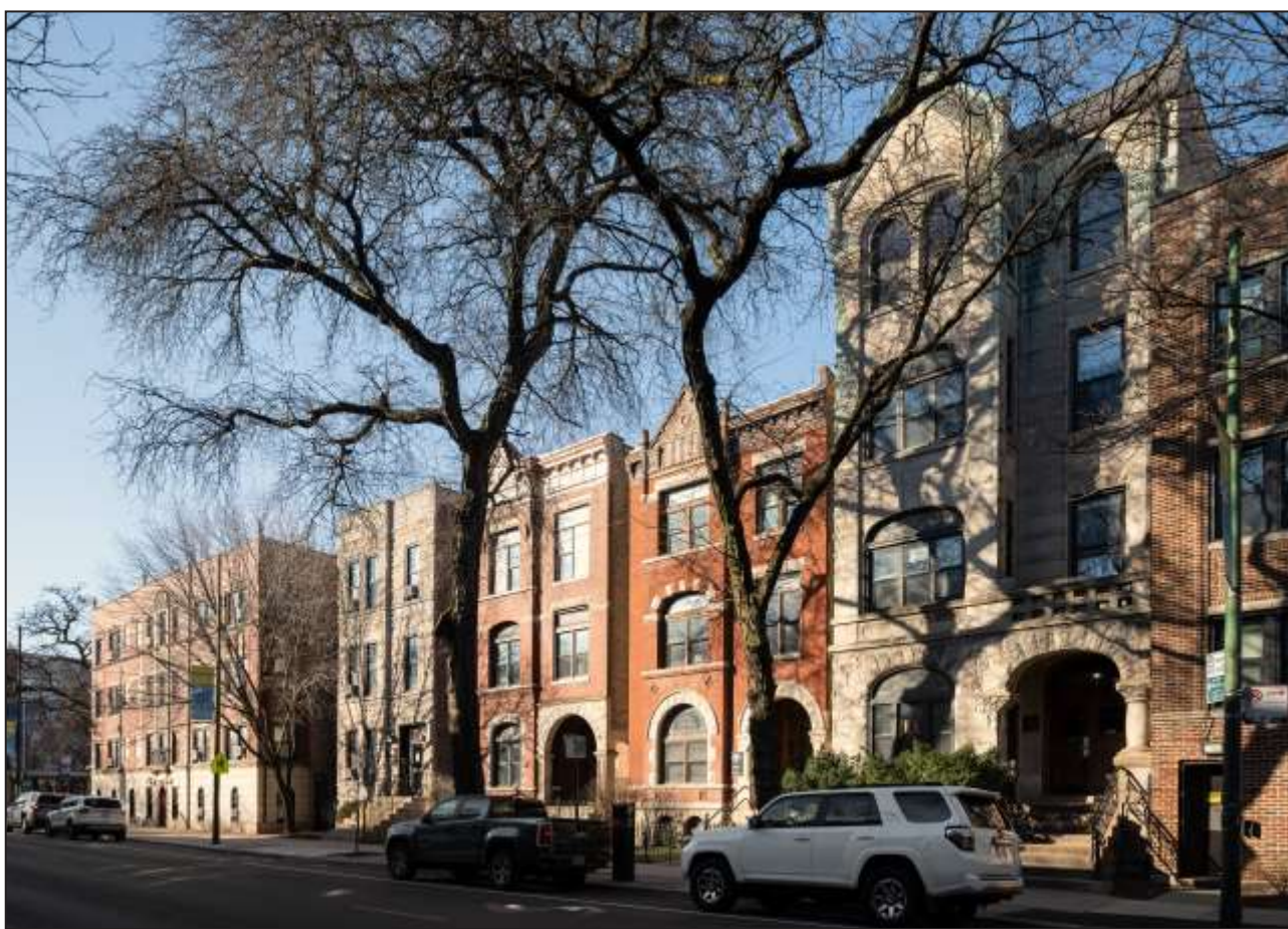
2314 N. Sheffield Avenue Detail. Photo Credit: Max Chavez / Preservation Chicago (top)
