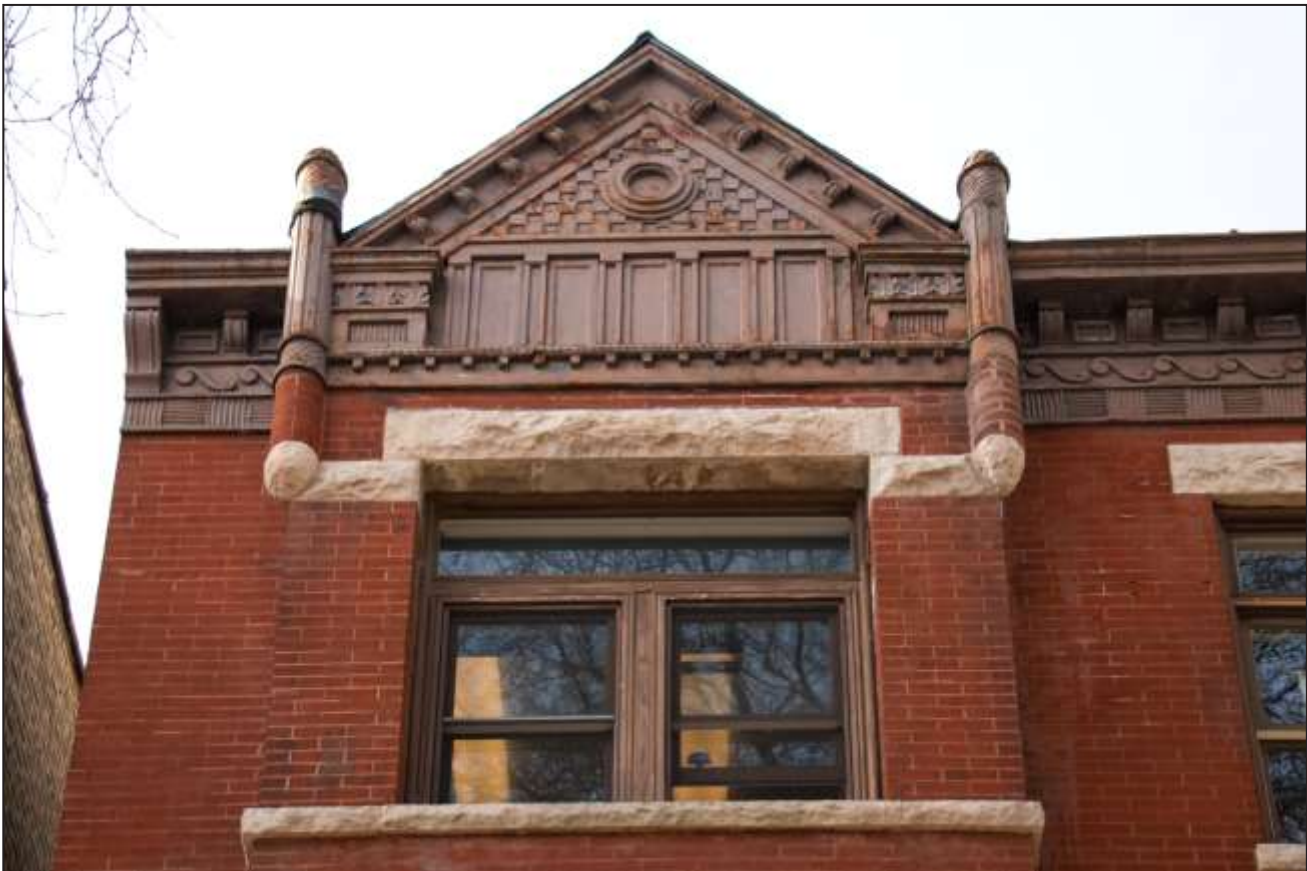
2310 and 2314 N. Sheffield Avenue Details, John Morrell, 1890-1893. Photo Credit: Max Chavez / Preservation Chicago (top & bottom)
