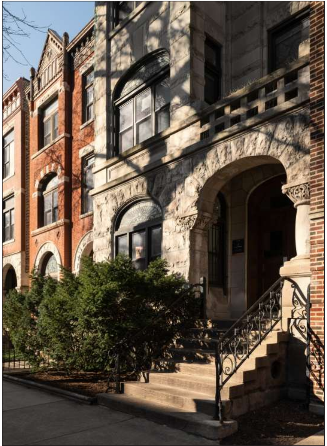
Sheffield-Belden Group, northwest corner of Sheffield and Belden Avenues. Freestanding townhouses, 2314 and 2316 N. Sheffield, John Morrell and others, 1890-1893. Photo Credit: Serhii Chucky / Esto
