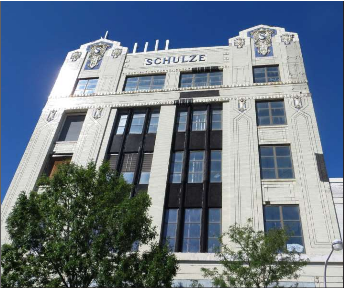
Wabash Avenue elevation, Schulze Baking Company Building, 1914, John Ahlschlager & Son, 40 E. Garfield Boulevard. Photo credit: Debbie Mercer
