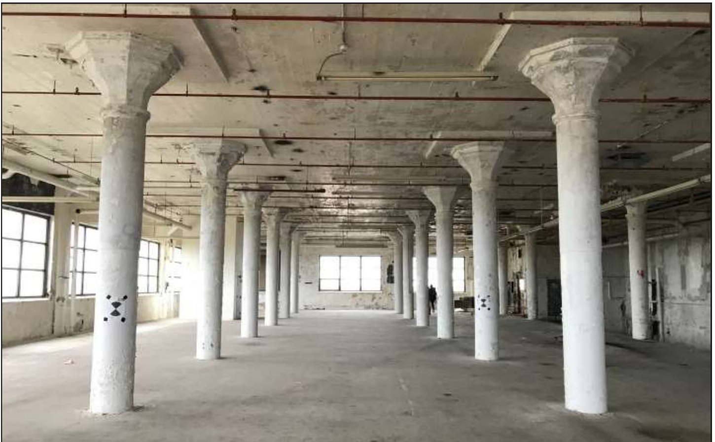
Interior view, Schulze Baking Company Building Interior, 1914, John Ahlschlager & Sons, 40 E. Garfield Boulevard. Photo credit: Debbie Mercer
