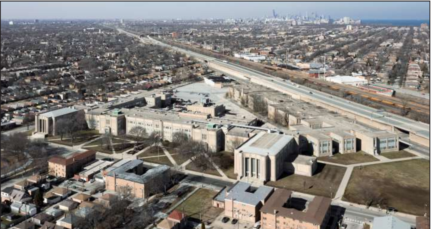
Chicago Vocational School (CVS) Anthony Avenue Wing Photo Credit: Max Chavez / Preservation Chicago Chicago Vocational School (CVS) Aerial Photograph Anthony Avenue Wing (parallel to Chicago Skyway). Photo Credit: Serhii Chrukly / Esto
