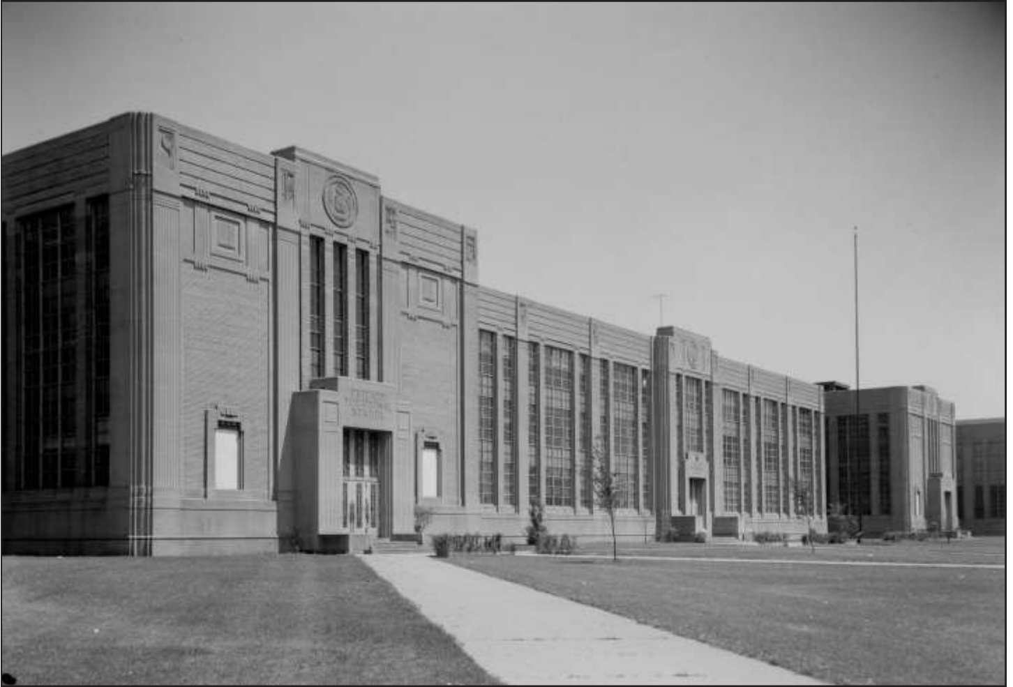
Chicago Vocational School (CVS), 1941, John Christensen, 2100 E. 87th Street. Photo Credit: Kaufmann & Fabry Co., Chicago Vocational School (CVS) Historic Exterior Photograph, East 87th Street and South Anthony Avenue, Circa 1950, Folder 201, Sheet 5, Photographic Images of Change, University of Illinois at Chicago. Library. Special Collections Department
