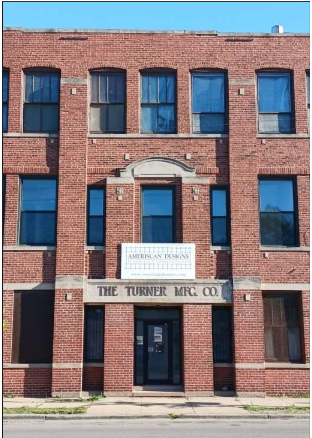
Ogden-Keeler Industrial Buildings, Turner Manufacturing Company Building, 4147-4151 W. Ogden, Alfred S. Alschuler, 1918 – 1921. Photo credit: Ward Miller / Preservation Chicago
