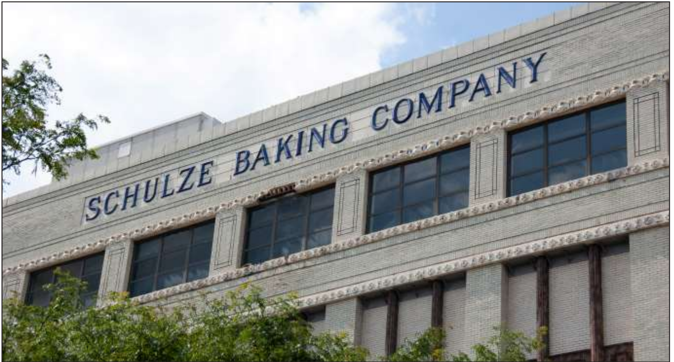
Garfield Blvd. elevation, Schulze Baking Company Bld., 1914, John Ahlschlager & Sons, 40 E. Garfield Boulevard. Photo credit: Eric Allix Rogers
