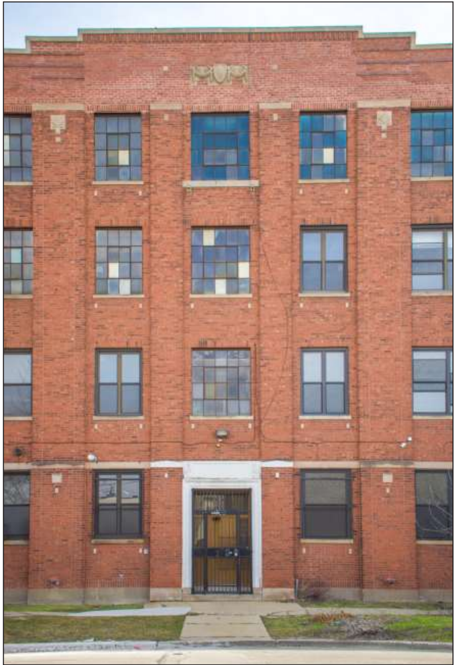
Ogden-Keeler Industrial Buildings, Turner Manufacturing Company Building, 4147-4151 W. Ogden, Alfred S. Alschuler, 1918 – 1921. Photo credit: Max Chavez / Preservation Chicago
