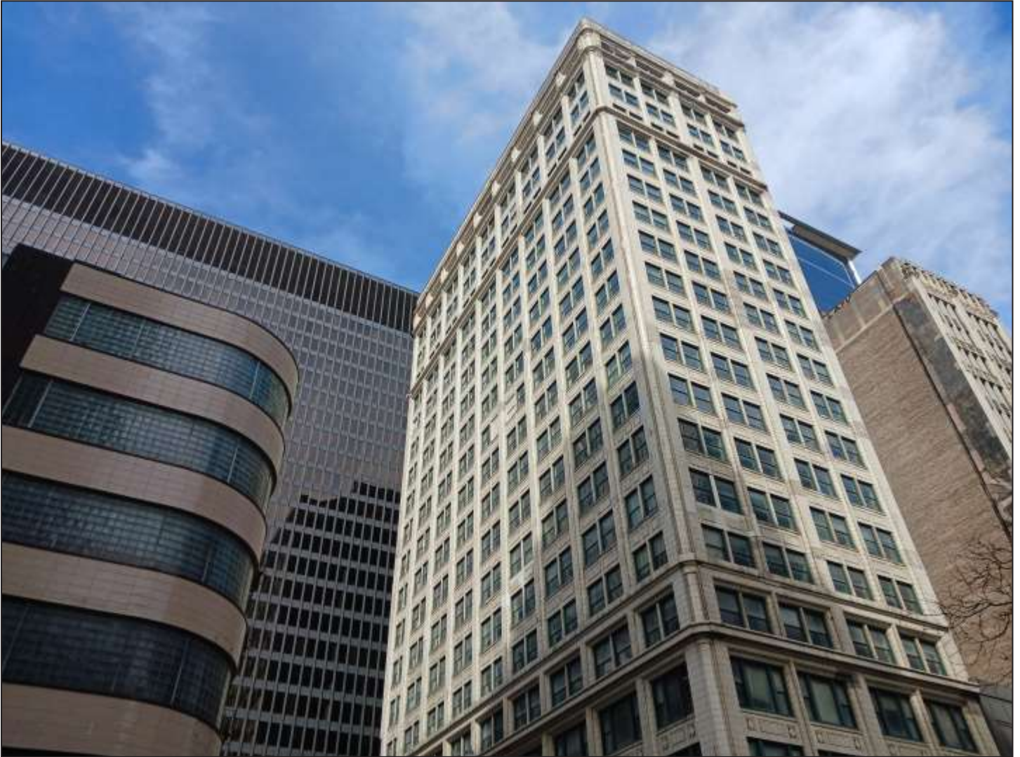
The Century and Consumers Buildings, Benson & Rixon Store with Dirksen Courthouse to the rear. Photo credit: Ward Miller / Preservation Chicago
