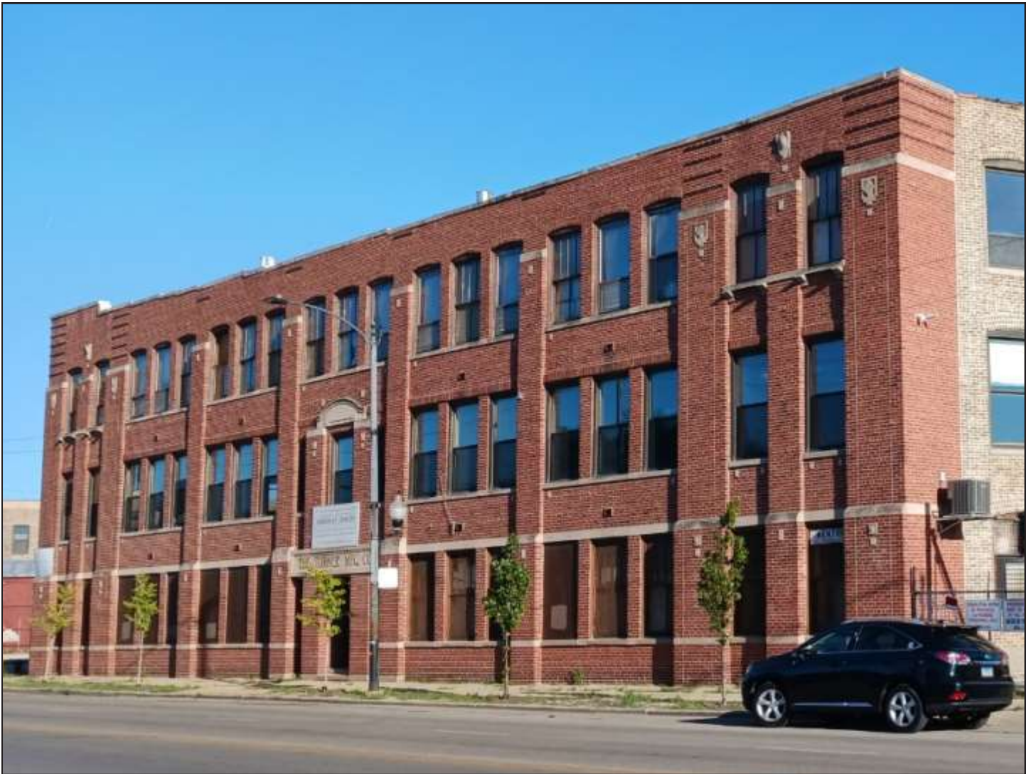
Ogden-Keeler Industrial Buildings, Turner Manufacturing Company Building, 4147-4151 W. Ogden, Alfred S. Alschuler, 1918 – 1921. Photo credit: Ward Miller / Preservation Chicago
