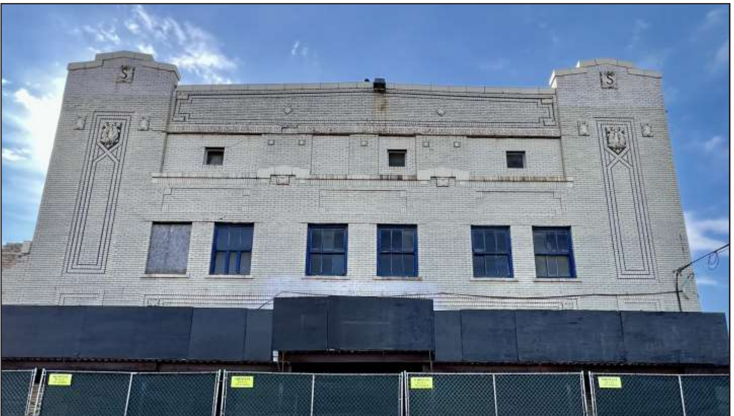
Schulze Baking Company Building Garage, 1914, John Ahlschlager & Sons, 21 E. 54th Street . Photo credit: Debbie Mercer
