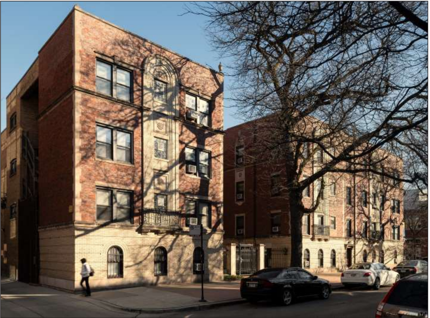
Sheffield-Belden Group, northwest corner of Sheffield and Belden Avenues. Courtyard building, 1000-1012 W. Belden and 2300-2302 N. Sheffield Avenue, Maher & McGraw, 1926. Photo Credit: Serhii Chrucky / Esto
