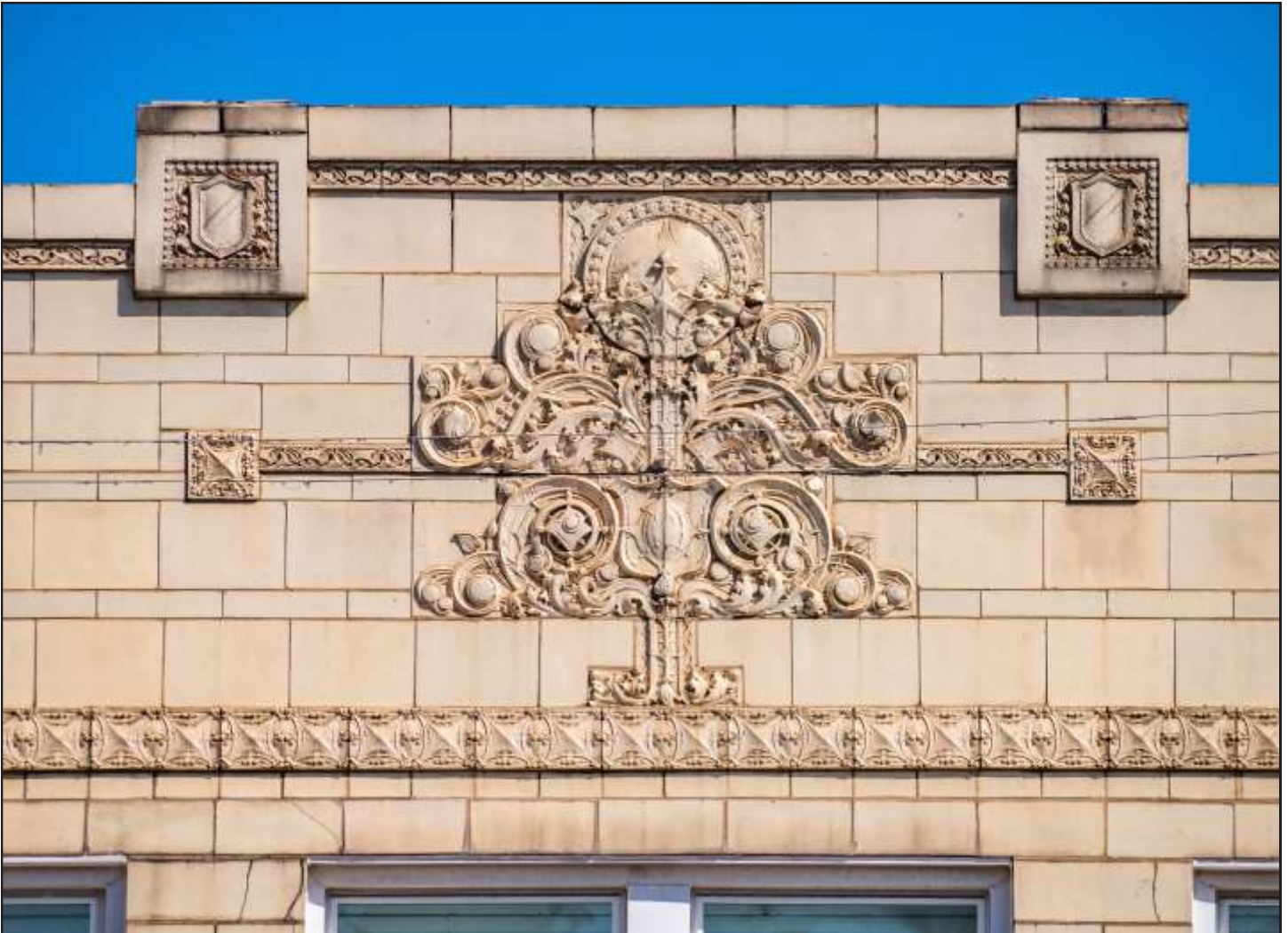
Sullivan-esque-style terra cotta ornament on the Polskie Centrum Medyczne Building, 1923, Rissman & Hirshfeld, 3015-3027 N. Milwaukee Avenue.
