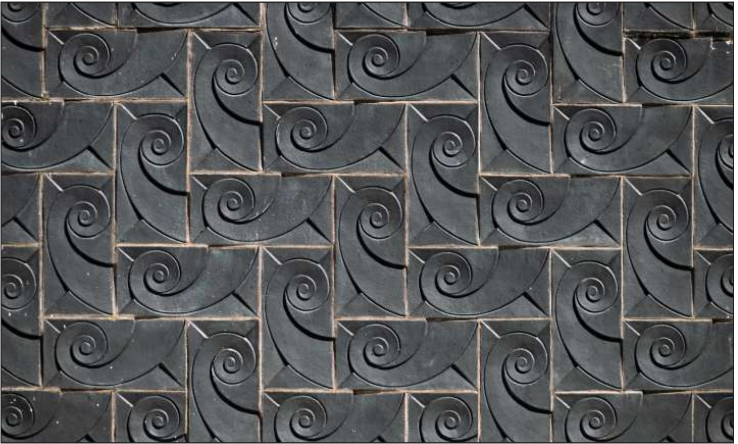
Terra cotta ornament at Lincoln-Melrose Building, 1930, Dubin & Dubin, 3232 N. Lincoln Avenue. Photo credit: Serhii Chrucky
