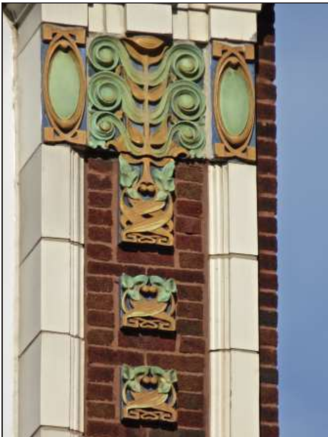
2542-2544 W. North Avenue, 1913, Harlev & Aga. Photo credit: Debbie Mercer
