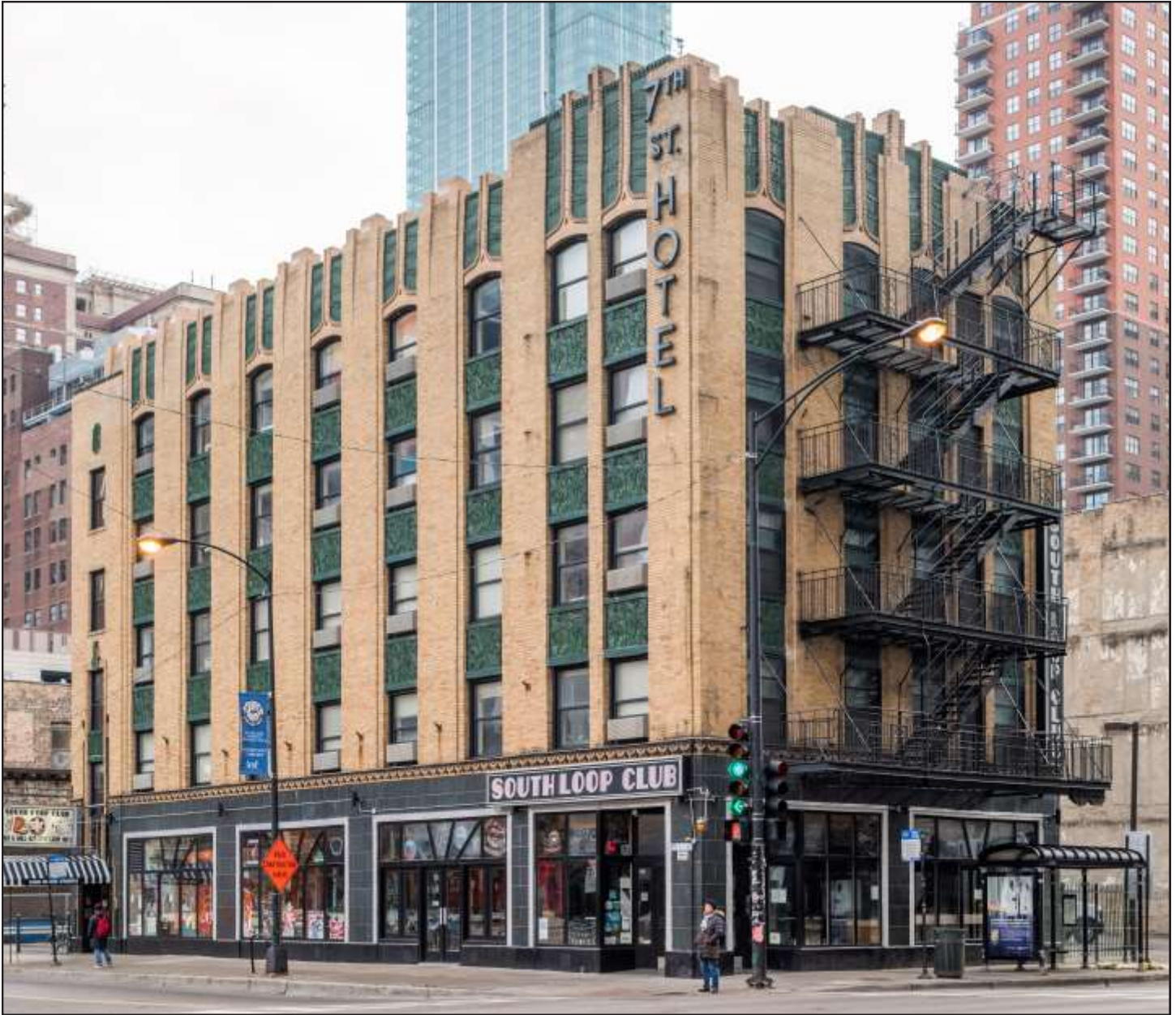
7th Street Hotel Building / Carter Hotel, 1930, Michaelson & Rognstad, 701 S. State Street / 1 E. Balbo Drive. Photo credit: Serhii Chrucky
