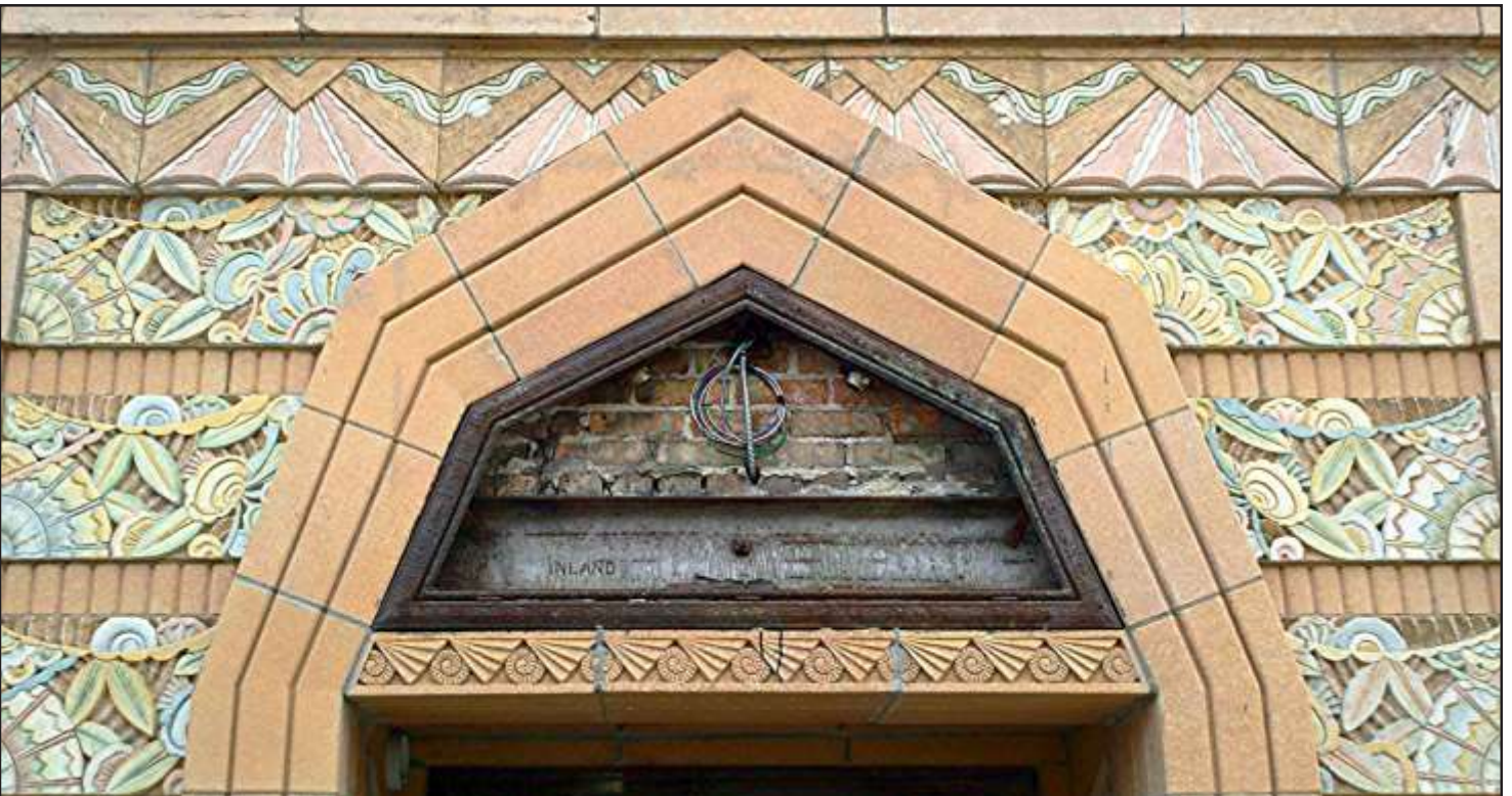
Former Viceroy Hotel / Union Park Hotel, 1929, Benjamin Albert Comm, 1519 W. Warren Boulevard. Photo credit: Debbie Mercer
