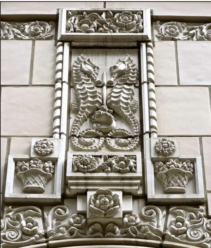
15 N. Wabash Avenue, 1903, Otis and Clark. Photo credit: Debbie Mercer
