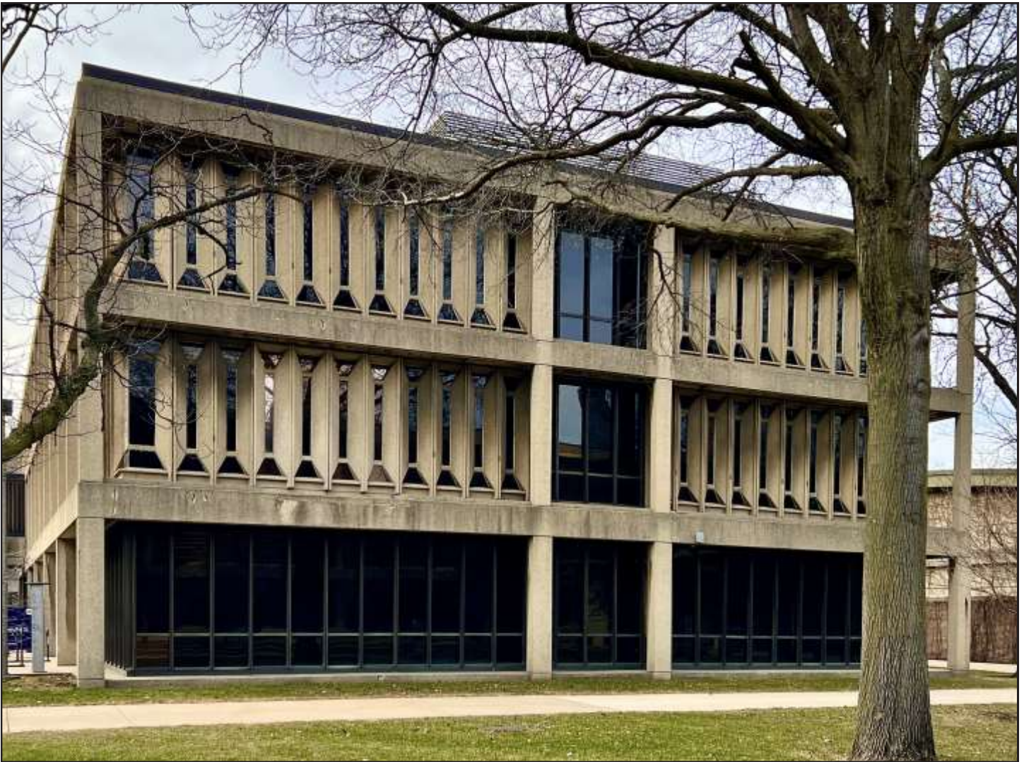
Taft Hall at the University of Illinois Chicago, 1965, Walter Netsch of Skidmore, Owings & Merrill (SOM), 826 S. Halsted Street. Photo credit: Max Chavez / Preservation Chicago
