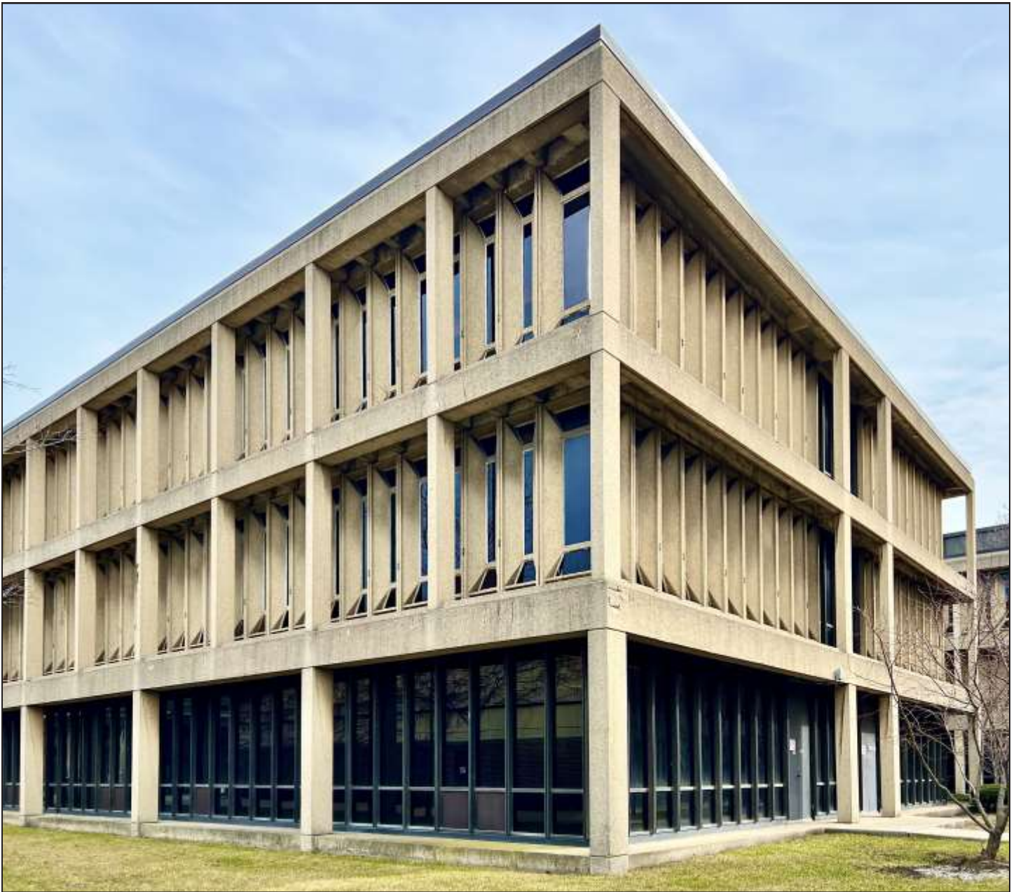
Taft Hall at the University of Illinois Chicago, 1965, Walter Netsch of Skidmore, Owings & Merrill (SOM), 826 S. Halsted Street. Photo credit: Max Chavez / Preservation Chicago
