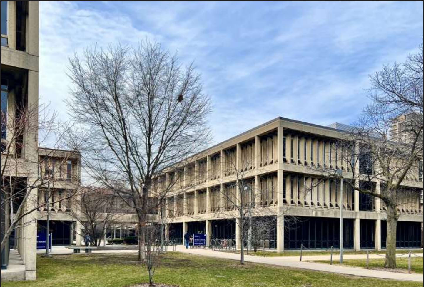
Taft Hall at the University of Illinois Chicago, 1965, Walter Netsch of Skidmore, Owings & Merrill (SOM), 826 S. Halsted Street. Photo credit: Max Chavez / Preservation Chicago
