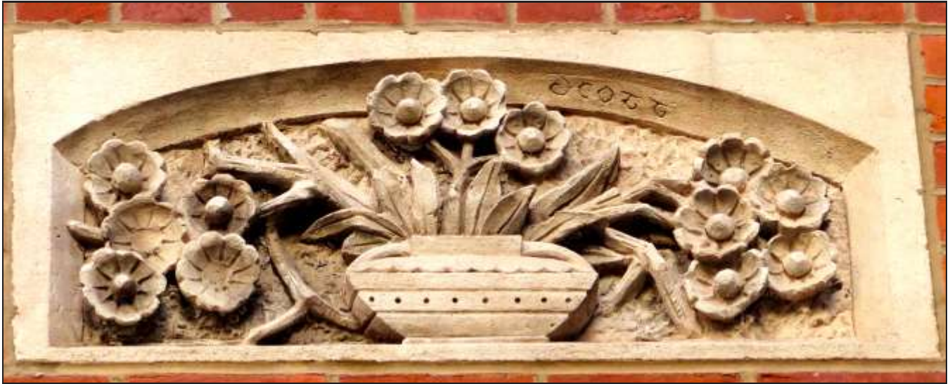
Oldest known terra cotta in Chicago. Isaac Scott terra cotta, signed and dated Scott 1877, located on the exterior of the 1401 N. Dearborn Street, 1877, architects Asa Lyon and Isaac Scott. Terra cotta manufactured by Chicago Terra Cotta Company. Photo credit: Bill Tyre
