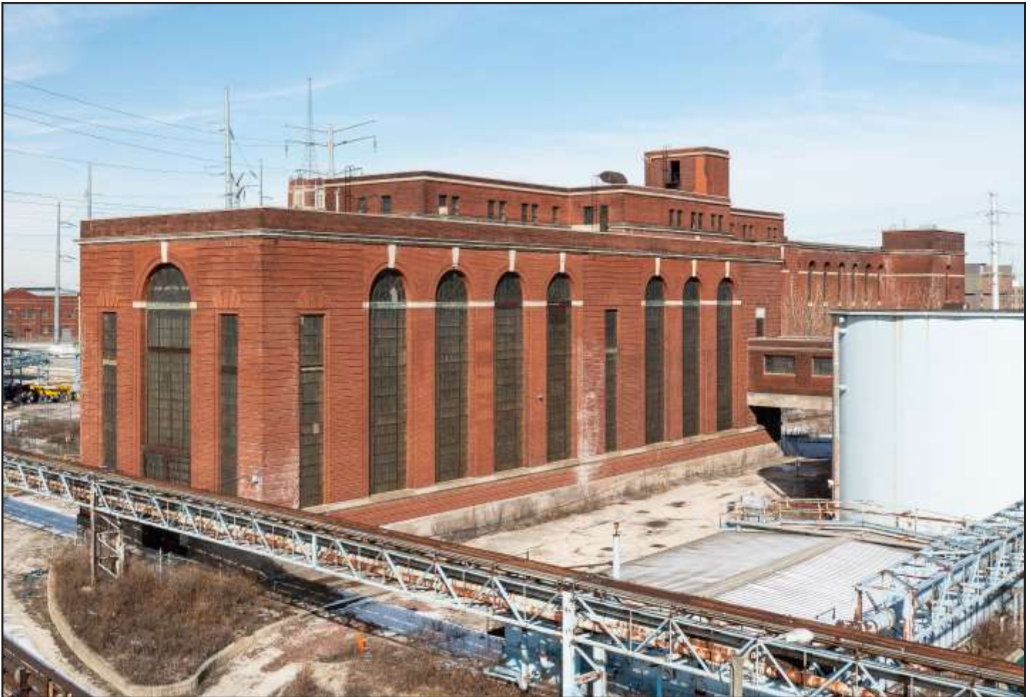
Fisk Power Station, 1903, Shepley, Rutan and Coolidge, 1111 W. Cermak Road with additions by others. Photo credit: Serhii Chrucky
