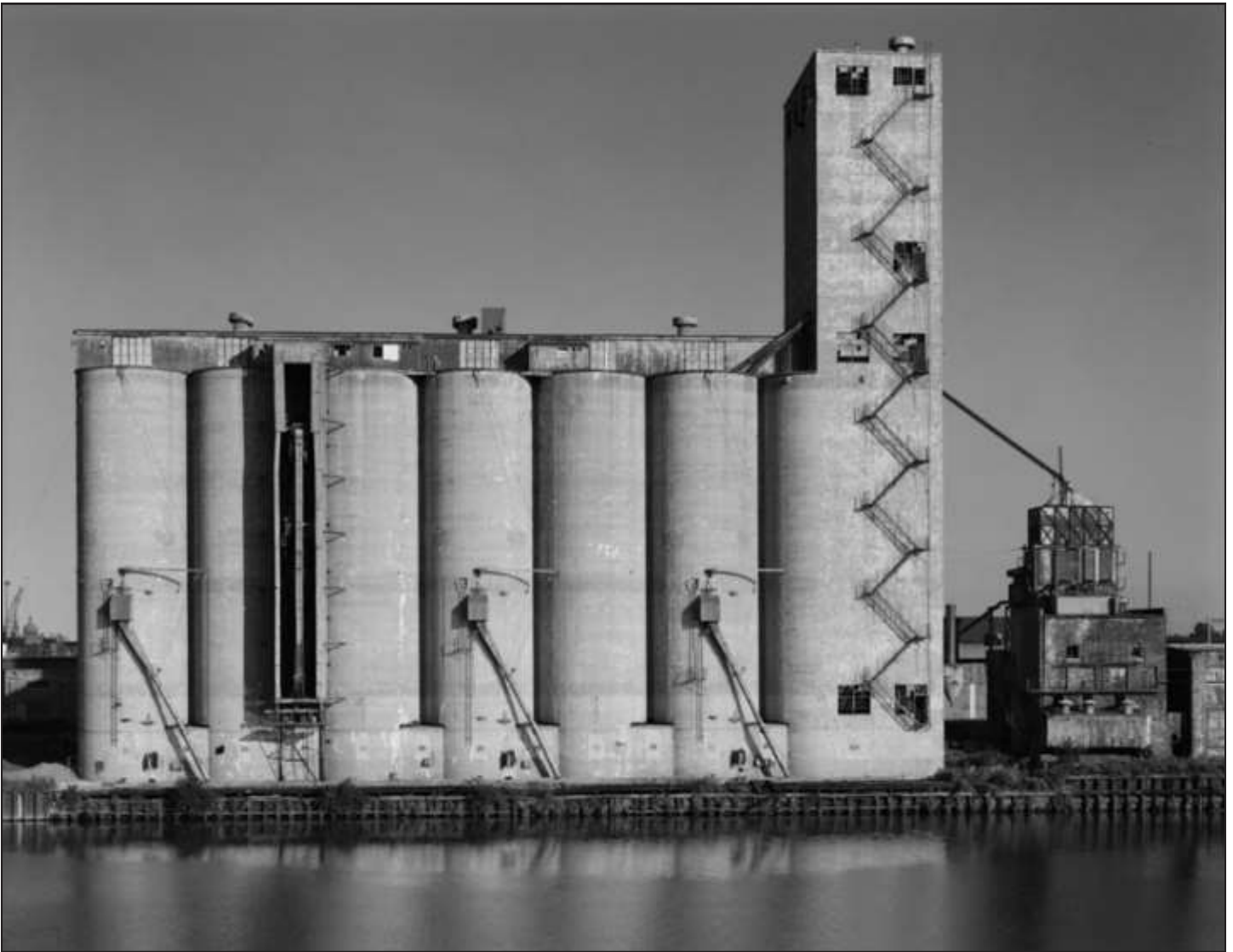
View of chimney and elevator from Damen Avenue Bridge - Santa Fe Railroad, Grain Elevator, South side of sanitary & ship canal, Chicago, Cook County, IL, Photo credit: Library of Congress, Historic American Engineering Record, HAER ILL, 16-CHIG, 155--4
