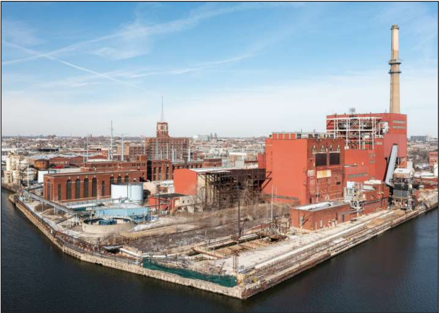
Fisk Power Station, 1903, Shepley, Rutan and Coolidge, 1111 W. Cermak Road with additions by others. Photo credit: Serhii Chrucky
