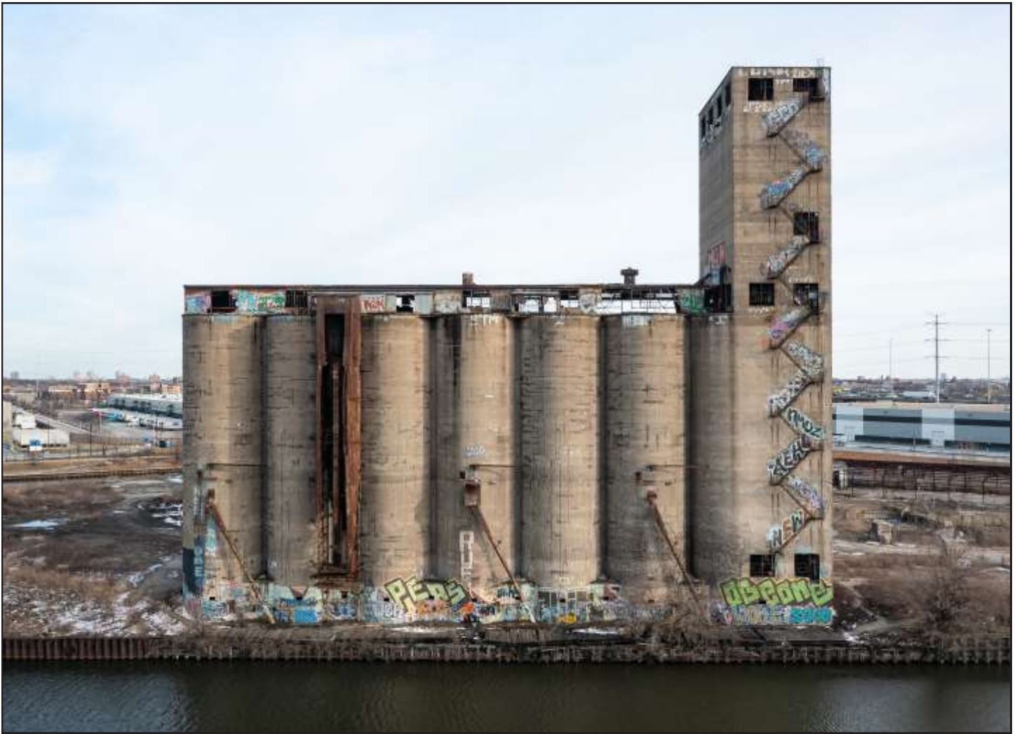
Damen Grain Silos, 1906, John Metcalf (civil engineer), 2860 S. Damen Avenue. Photo credit: Serhii Chrucky
