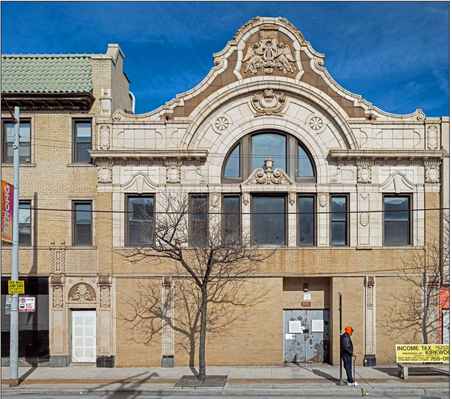
Jeffery Theater Building and Spencer Arms Hotel, 1924, William P. Doerr, 1952 E. 71st Street & 1950 E. 71st Street. Photo Credit: Serhii Chucky
