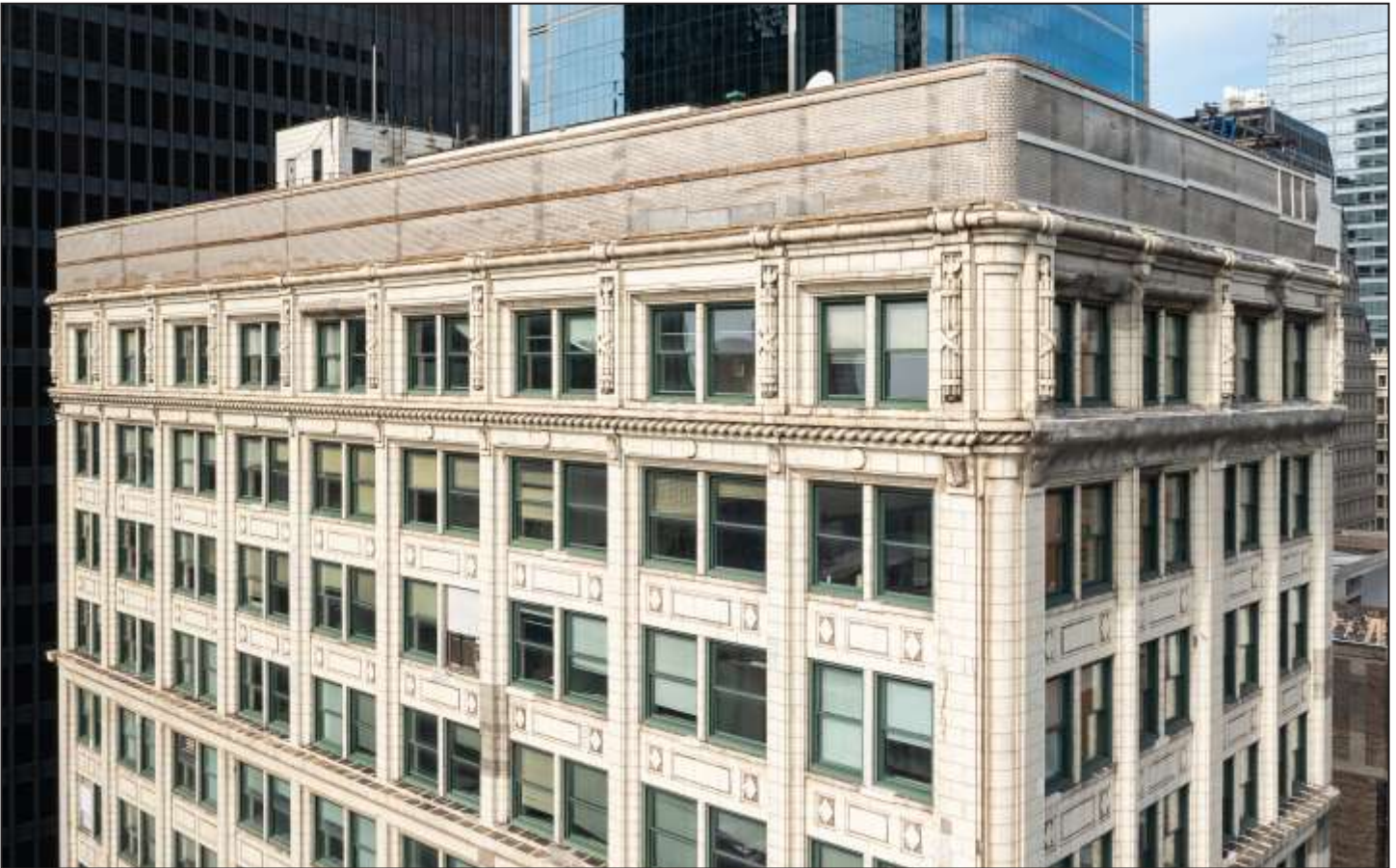
Detail of upper façade and cornice of Consumers Building, 1913, Jenney, Mundie & Jensen, 220 S. State Street, c. 2023. Photo credit: Serhii Chrucky
