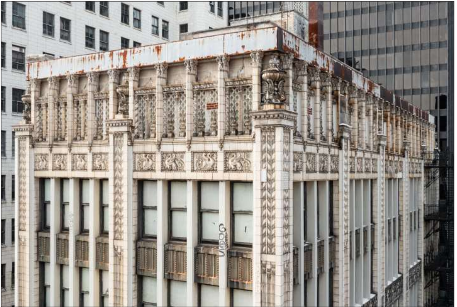
Detail of upper façade and cornice of Century Building, 1915, Holabird and Roche, 202 S. State Street. Photo credit: Serhii Chucky
