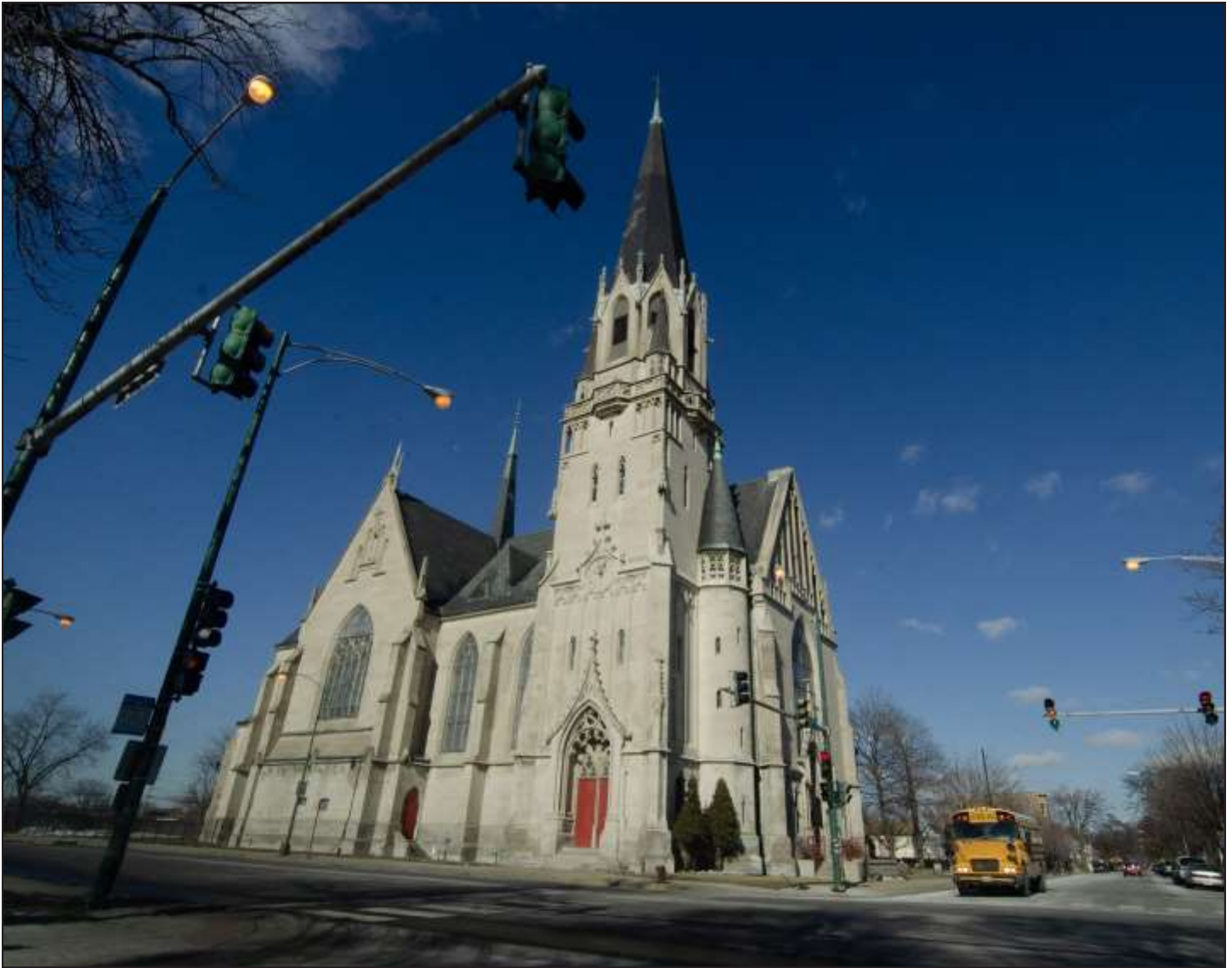
St. Martin de Tours Church, 1895, Henry J. Schlacks, 5848 S. Princeton Avenue. Photo Credit: Eric Allix Rogers
