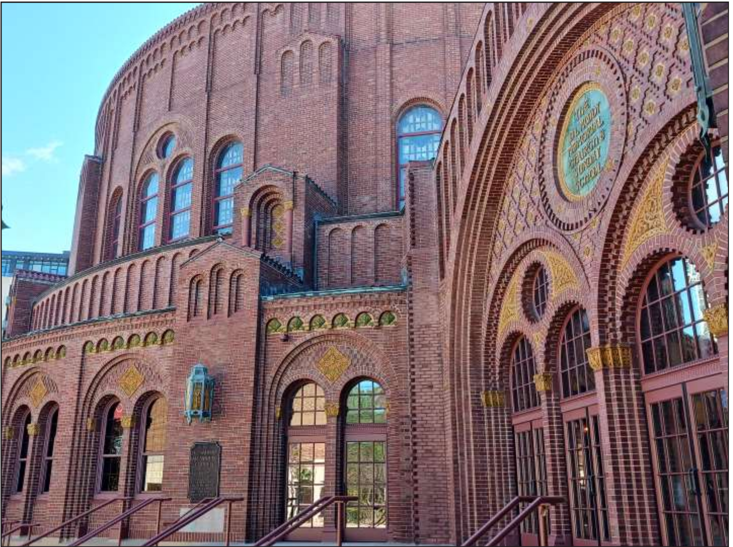
D.L. Moody Memorial Church, 1924, Fugard & Knapp, 1630 N. Clark Street. Photo Credit: Ward Miller / Preservation Chicago
