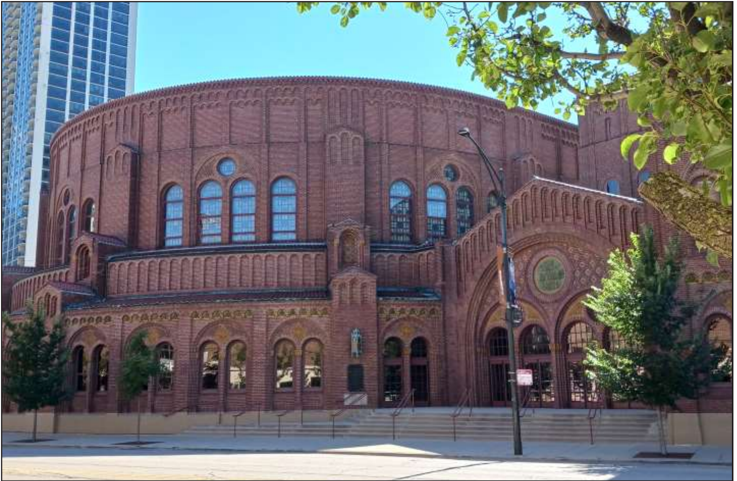
D.L. Moody Memorial Church, 1924, Fugard & Knapp, 1630 N. Clark Street. Photo Credit: Ward Miller / Preservation Chicago
