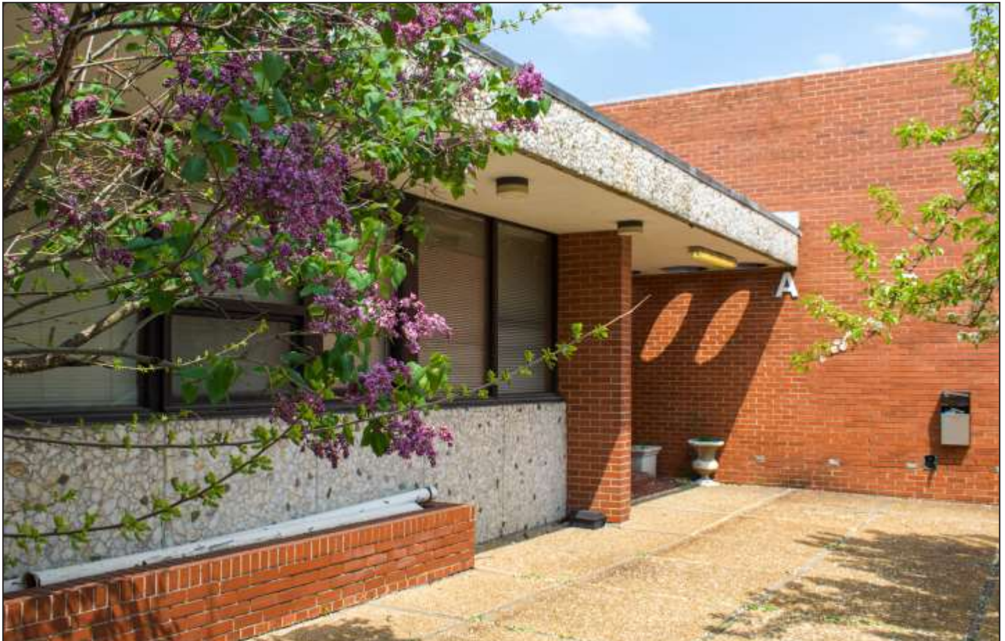
Peterson Avenue Midcentury Modern District, 3550 W. Peterson Avenue. Photo Credit: Max Chavez / Preservation Chicago
