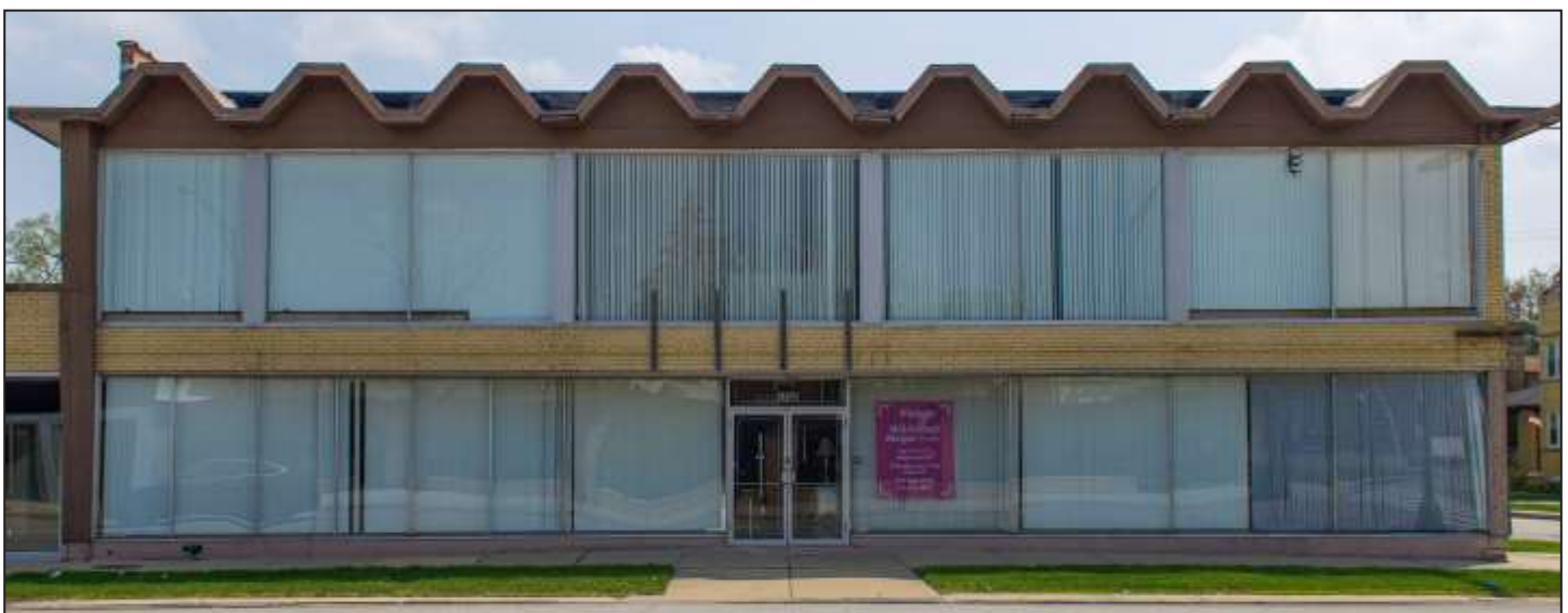
Peterson Avenue Midcentury Modern District, 3455 W. Peterson Avenue. Photo Credit: Max Chavez / Preservation Chicago
