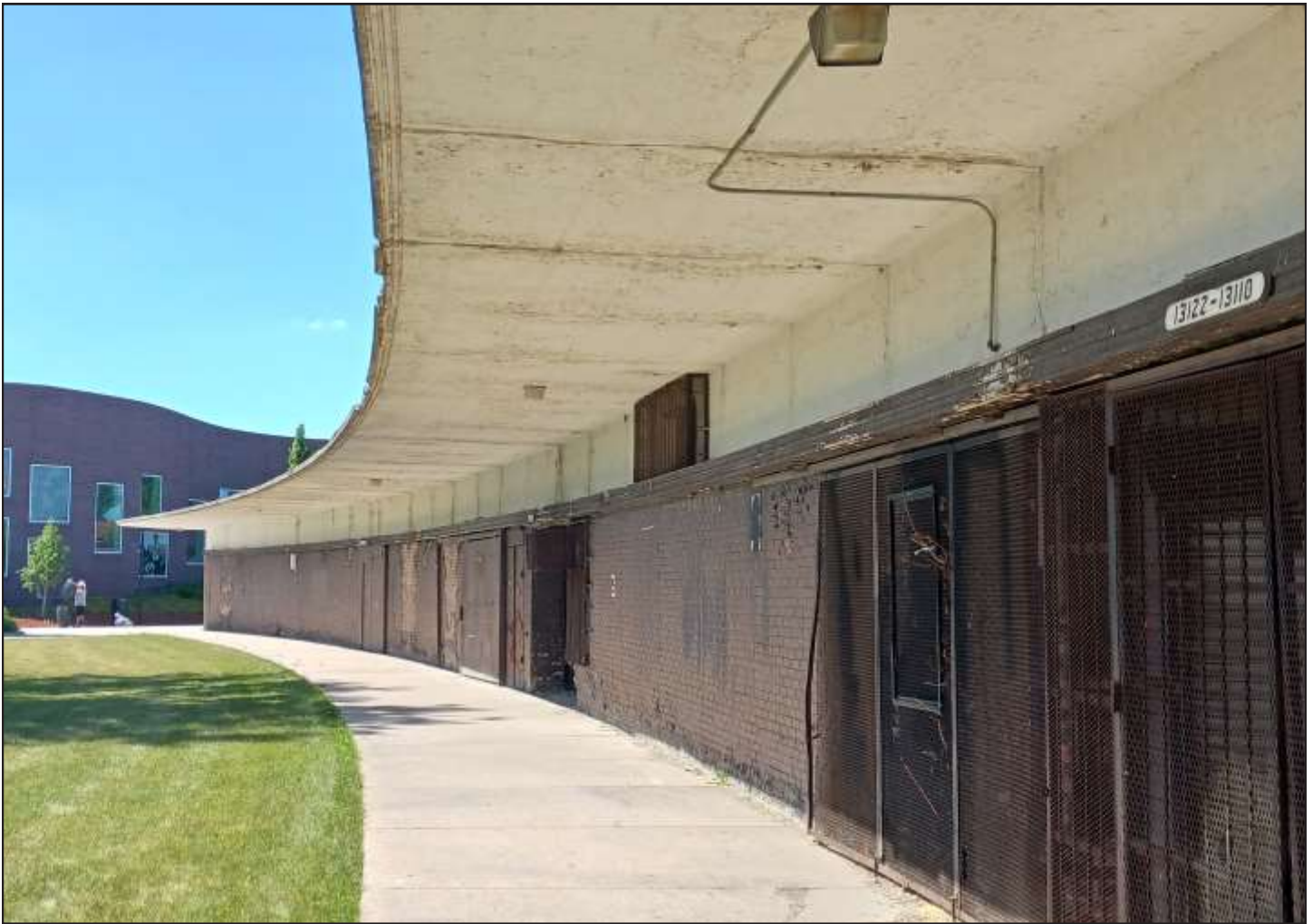
Altgeld Gardens Commercial Building 'Up Top', 1946, Keck & Keck, 13100 S. Ellis Avenue. Photo Credit: Ward Miller / Preservation Chicago
