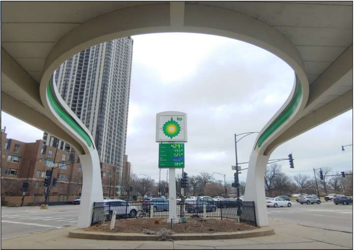
Archway Standard Station/BP Service Station, 1971, George Terp, 1647 N. LaSalle Street. Photo Credit: Ward Miller / Preservation Chicago
