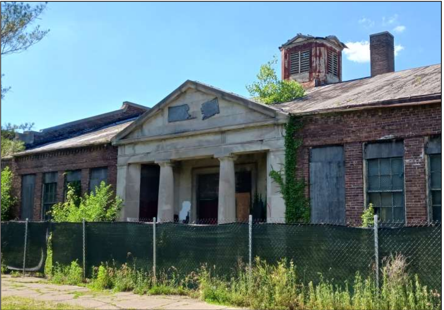
Altgeld Gardens Carver School 'C Building', 1944, Naess & Murphy, between 133rd Street and 133rd Place. Photo Credit: Ward Miller
