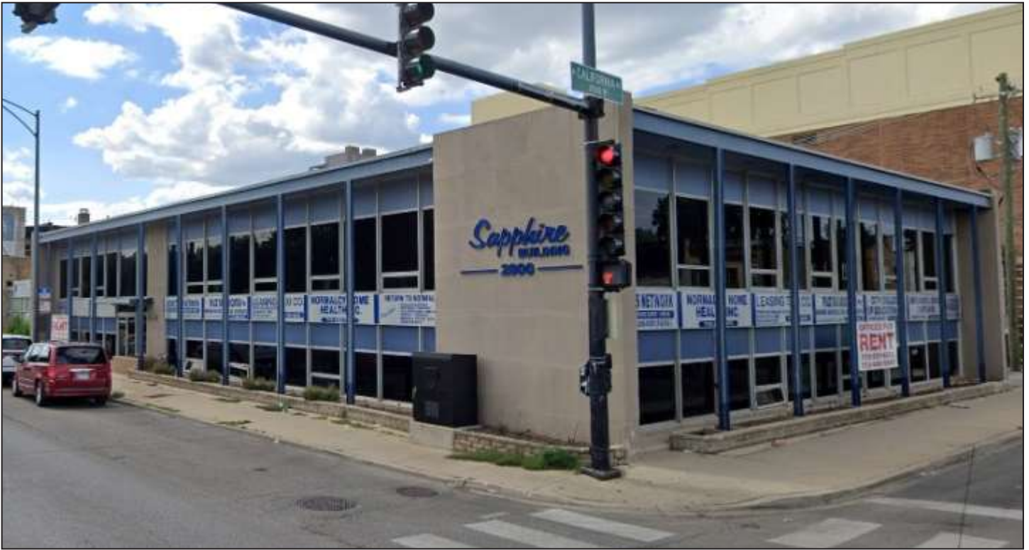
Peterson Avenue Midcentury Modern District, The Sapphire Building / Business House, 1960, Henry L. Newhouse II, 2800 W. Peterson Avenue. Demolished May 2022. Photo Credit: Google Maps
