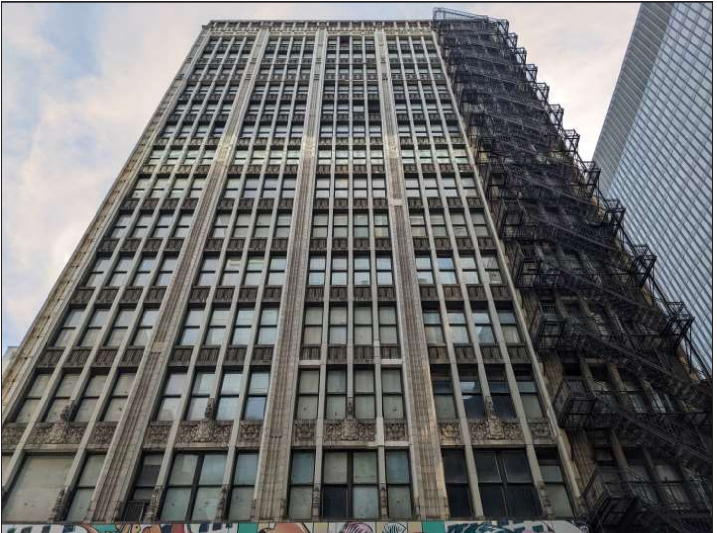
The Century Building, 1915, Holabird and Roche, 202 S. State Street. Photo credit: Eric Allix Rogers
