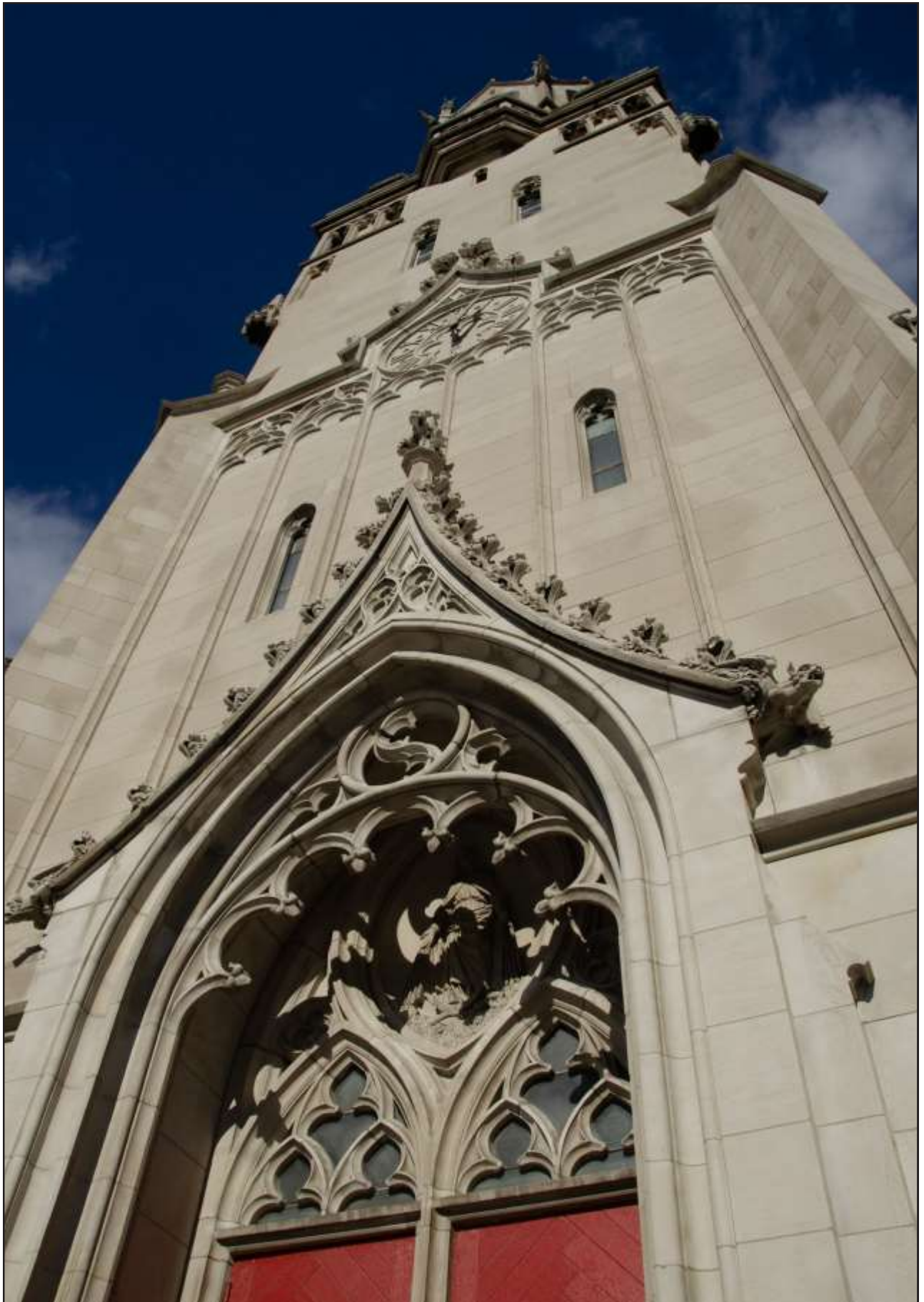
St. Martin de Tours Church, 1895, Henry J. Schlacks, 5848 S. Princeton Avenue. Photo Credit: Eric Allix Rogers
