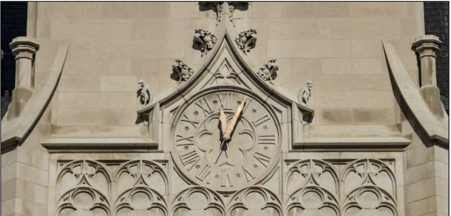
St. Martin de Tours Church, 1895, Henry J. Schlacks, 5848 S. Princeton Avenue. Photo Credit: Eric Allix Rogers
