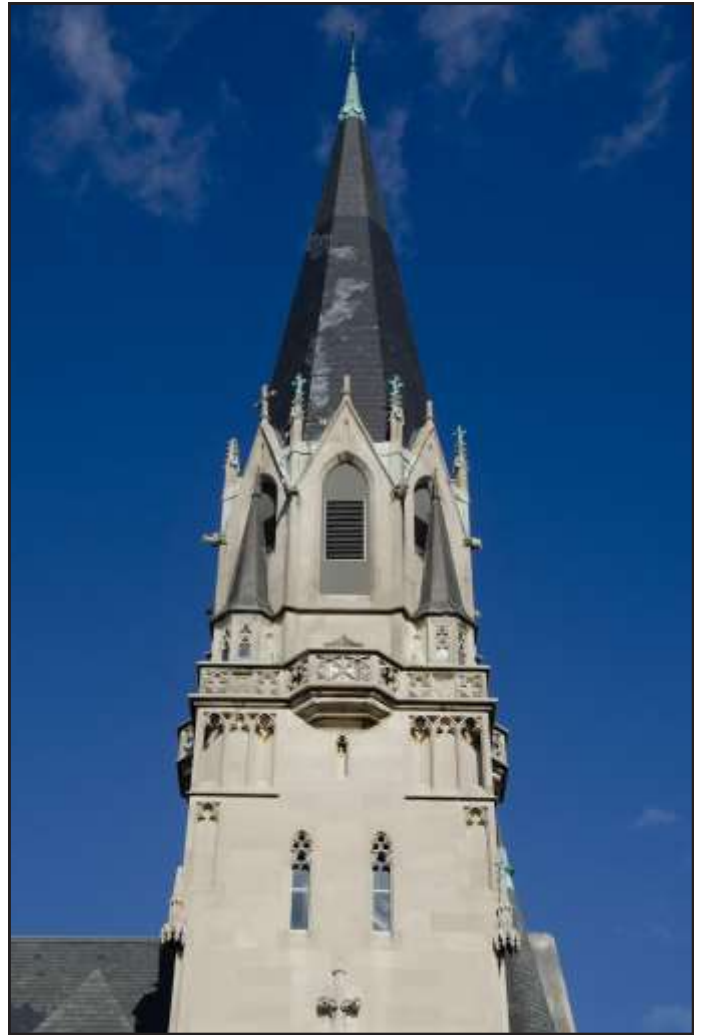
St. Martin de Tours Church, 1895, Henry J. Schlacks, 5848 S. Princeton Avenue. Photo Credit: Eric Allix Rogers
