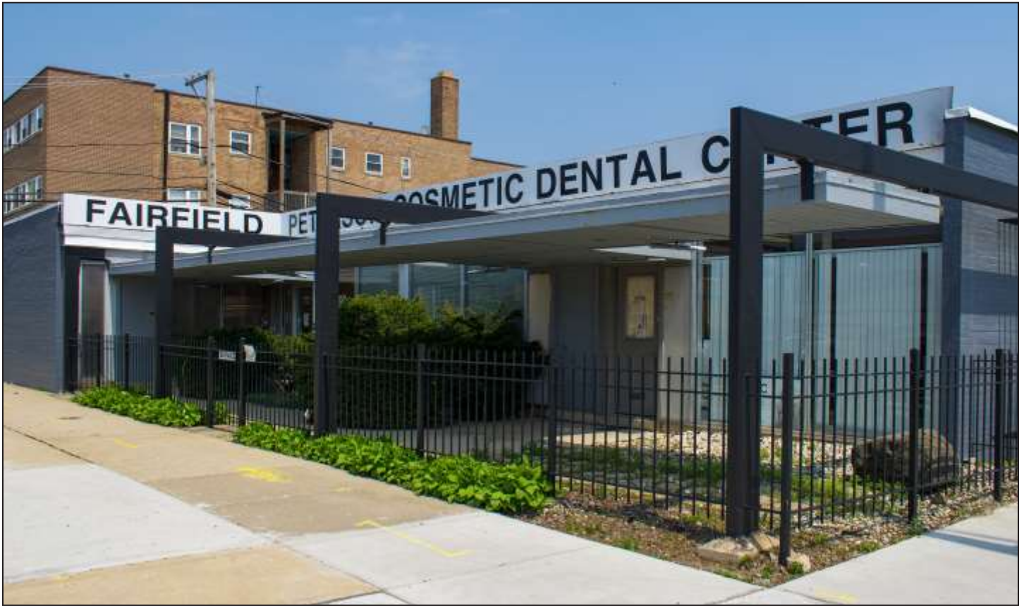
Peterson Avenue Midcentury Modern District, 2722 W. Peterson Avenue. Photo Credit: Max Chavez / Preservation Chicago
