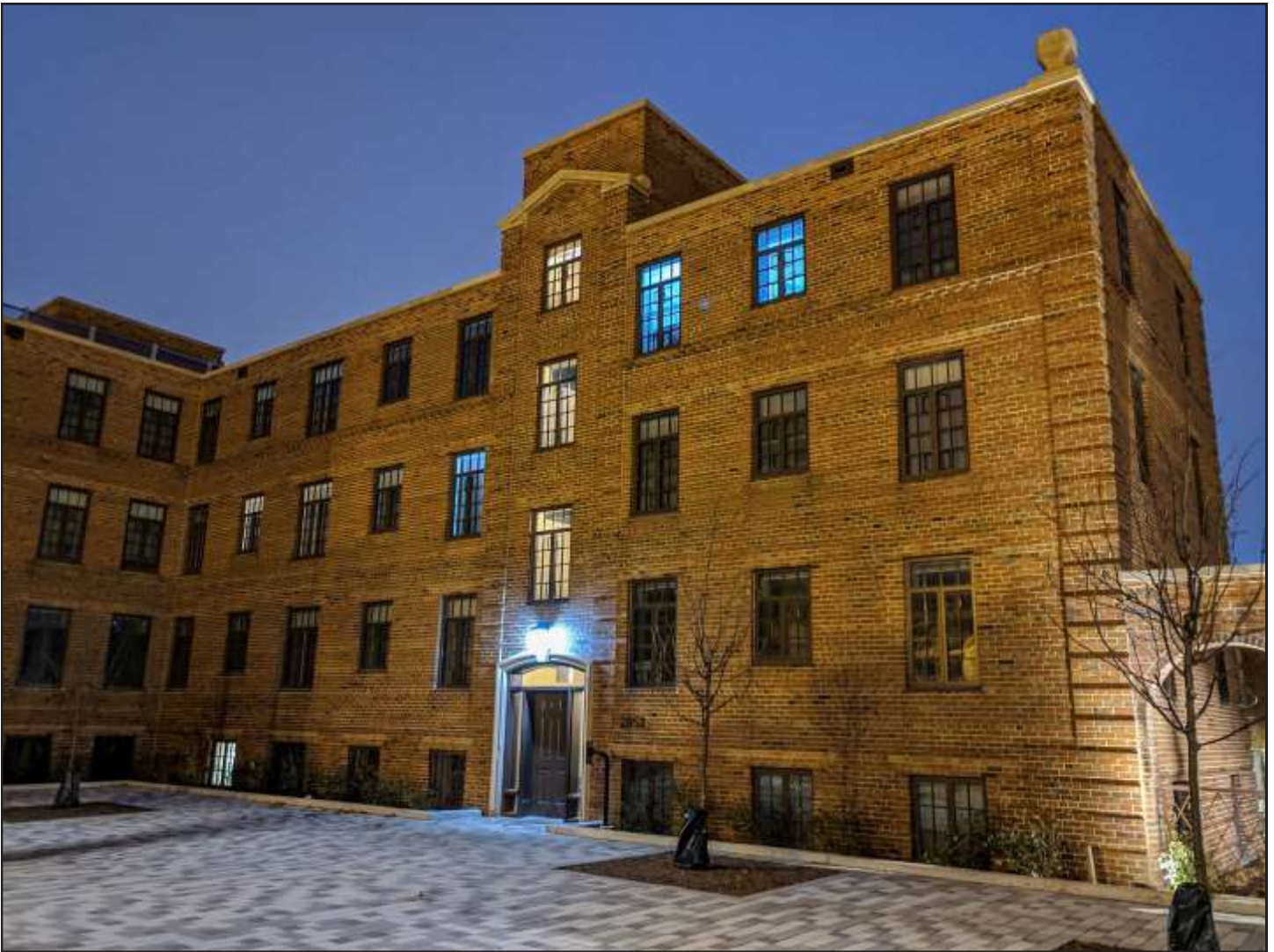
Lathrop Homes North Campus after comprehensive restoration. Photo Credit: Eric Allix Rogers
