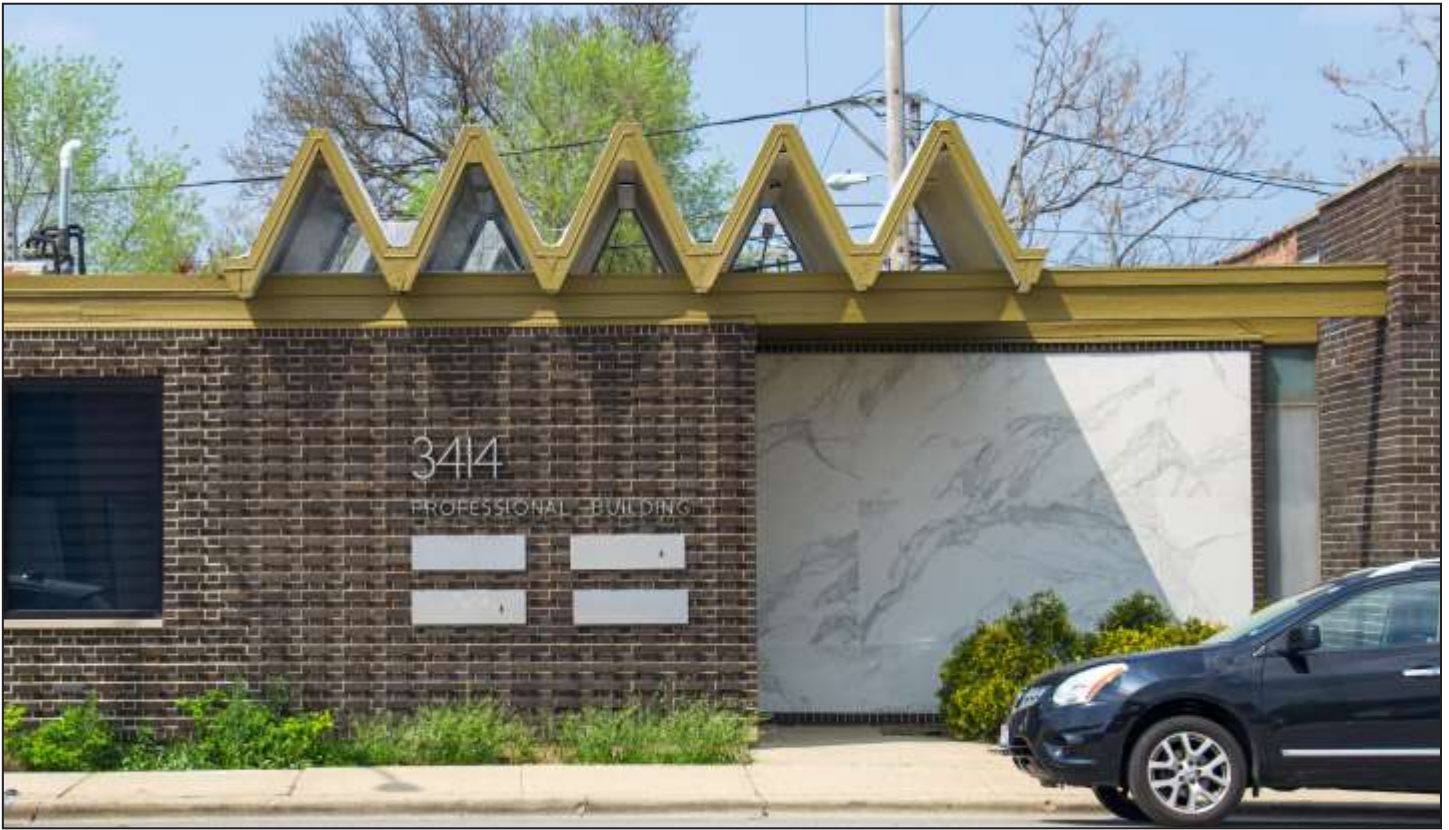
Peterson Avenue Midcentury Modern District, 3414 W. Peterson Avenue. Photo Credit: Max Chavez / Preservation Chicago
