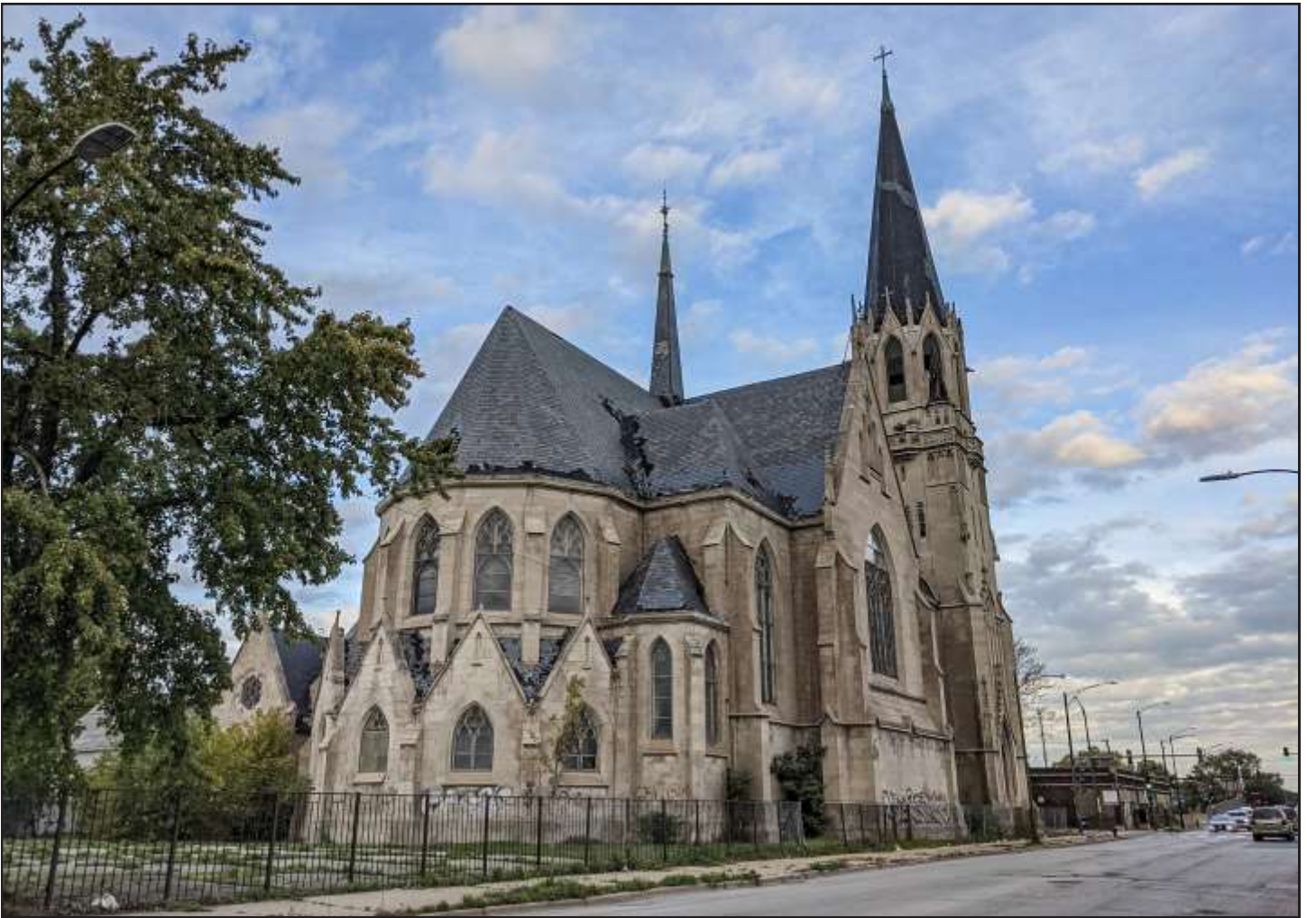
St. Martin de Tours Church, 1895, Henry J. Schlacks, 5848 S. Princeton Avenue. Photo Credit: Eric Allix Rogers
