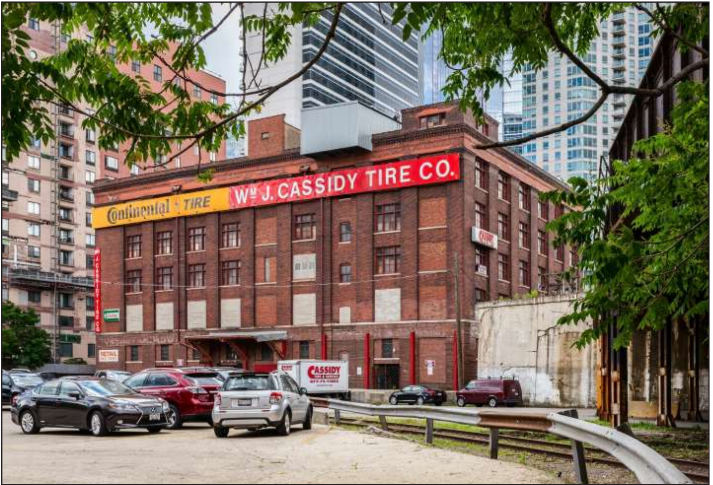
Tyler & Hippach Glass Company Building / William J. Cassidy Tire Building, 1902, Henry J. Schlacks, 344 N. Canal Street © Serhii Chrukky
