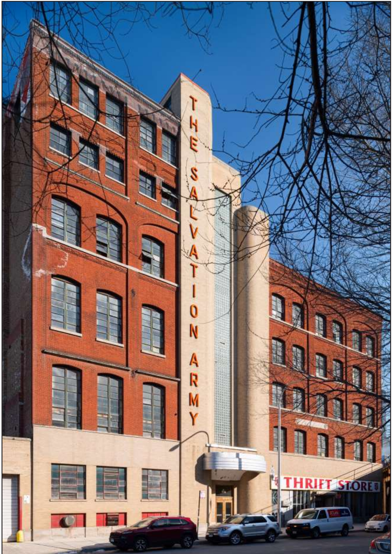
Braun & Fitts Butterine Factory / Wrigley Lodge / Salvation Army Bldg., 1891, Furst & Rudolph, 509 N. Union Avenue © Serhii Chrucky
