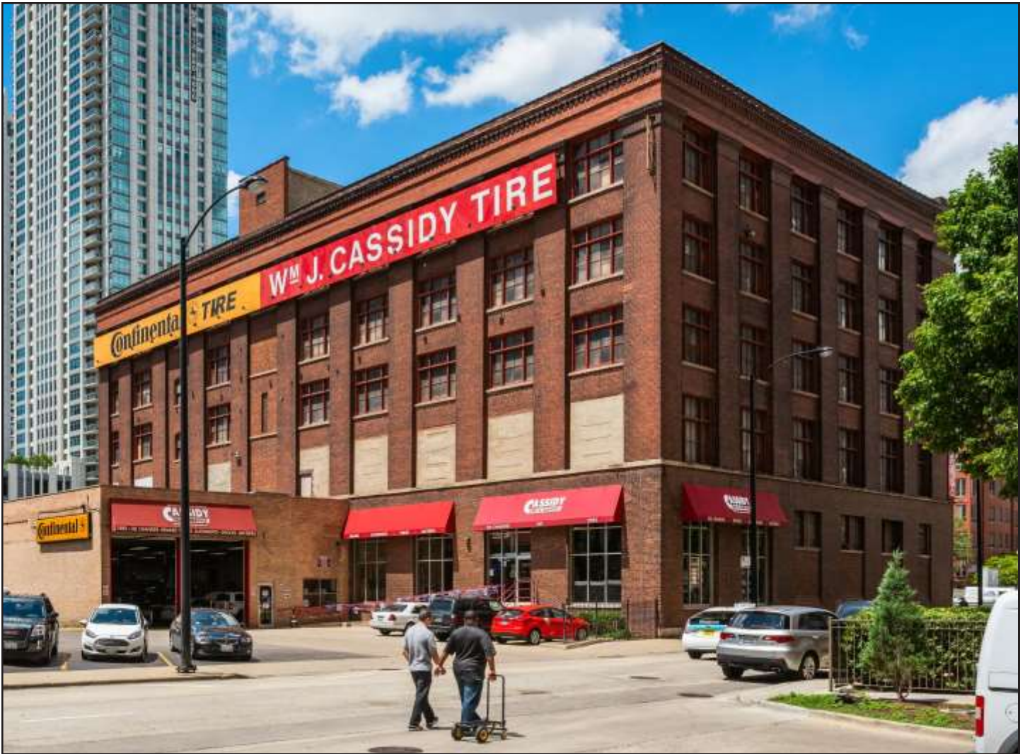
Tyler & Hippach Glass Company Building / William J. Cassidy Tire Building, 1902, Henry J. Schlacks, 344 N. Canal Street © Serhii Chucky
