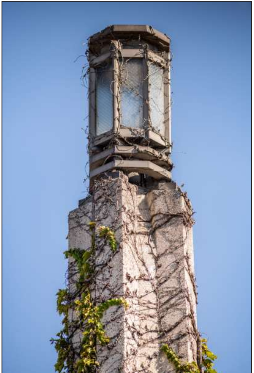
Lake Shore Drive's North Avenue Bridge Detail © Serhii Chrukky
