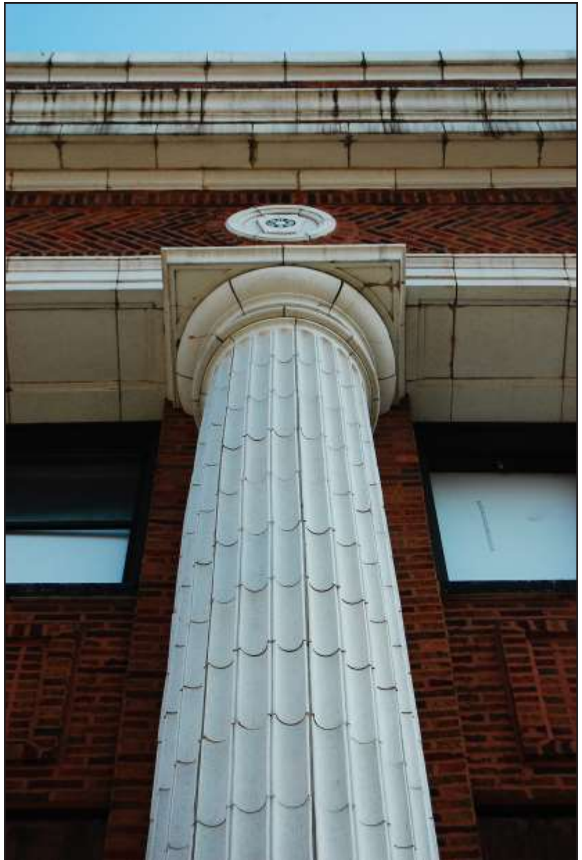
South Chicago Masonic Temple 91st Street Column Façade Detail © Eric Allix Rogers
