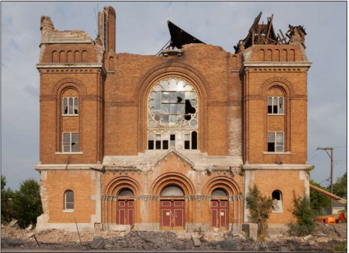
Demolition in 2014 of St. Laurence Church in South Shore © Noah Vaughn
