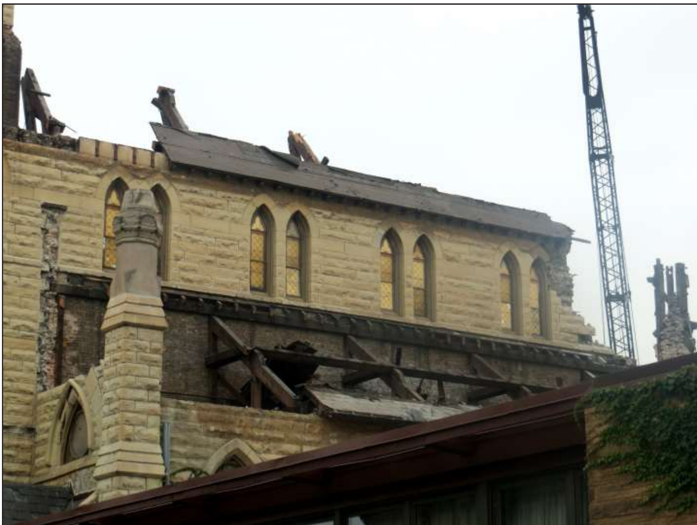
Demolition in 2013 of 'Old' St. James Church in Bronzeville © Deborah Mercer
