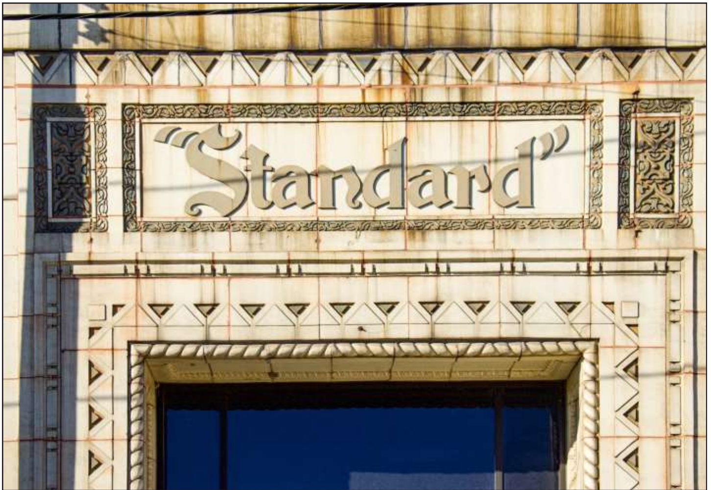
Central Manufacturing District - Original East District, Standard Sanitary Mfg. Co. Doorway, 3716 S. Iron, Alfred Alschuler, 1924. © Max Chavez
