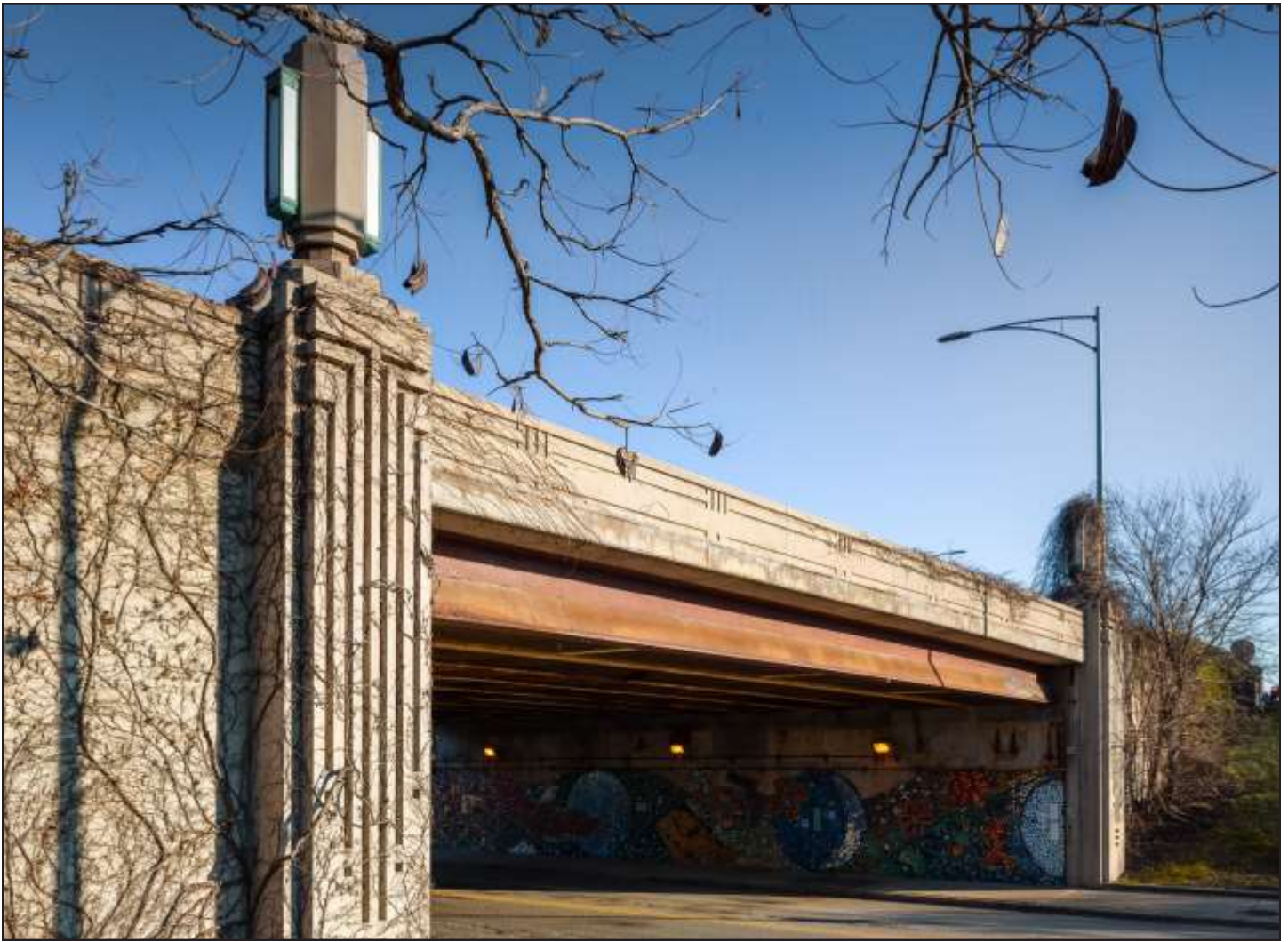
Foster Avenue Bridge over North Lake Shore Drive © Serhii Chrukky
