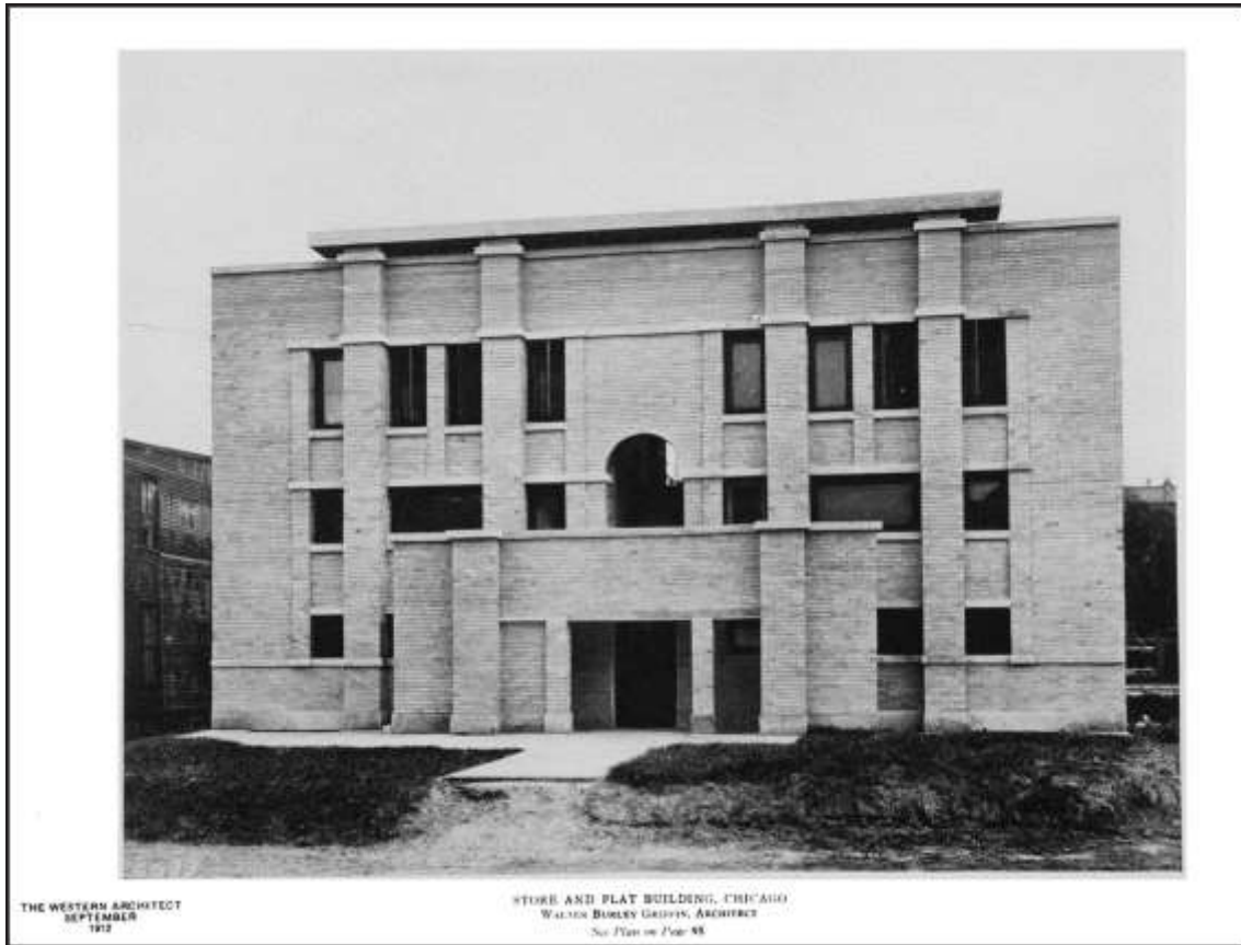
Cornell Store & Flats historic image, north facade, 1230-32 E. 75th Street © The Western Architect, September 1912
