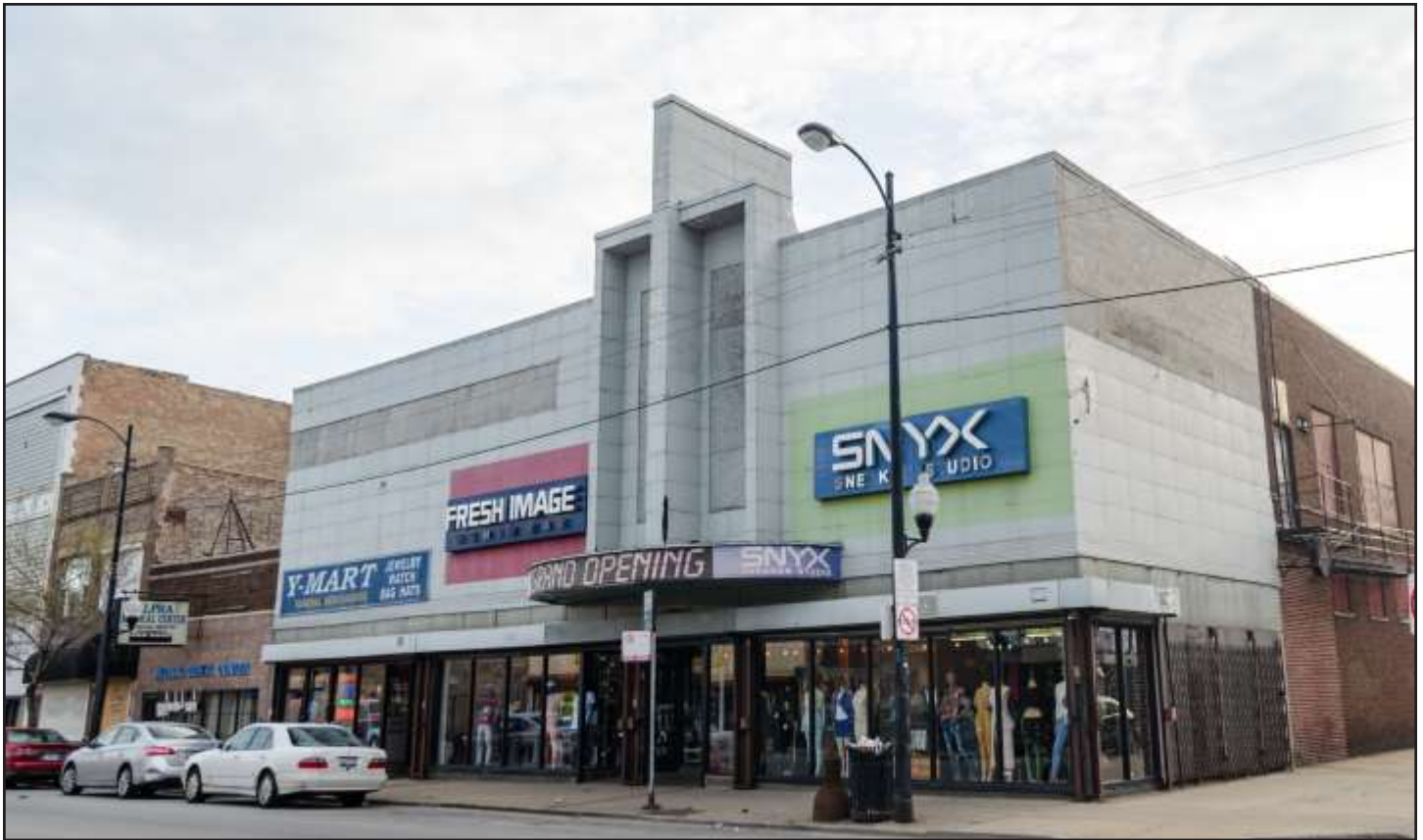
112th Place block on Roseland's Michigan Avenue Commercial District © Eric Allix Rogers
