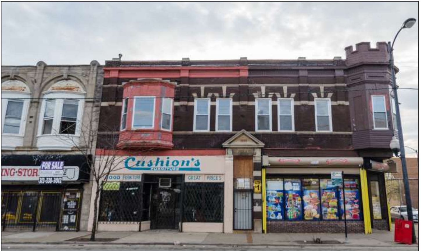
113th Place corner on Roseland's Michigan Avenue Commercial District © Eric Allix Rogers
