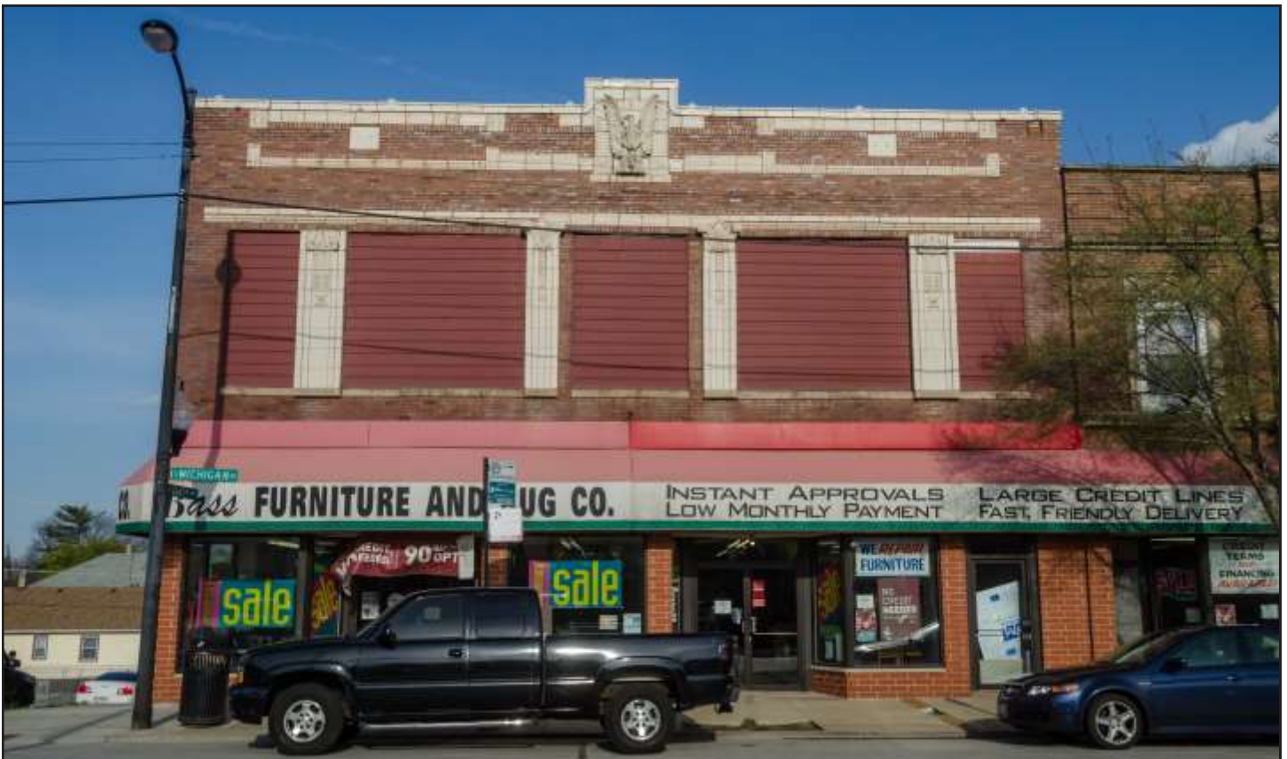
114th Place block on Roseland's Michigan Avenue Commercial District © Eric Allix Rogers
