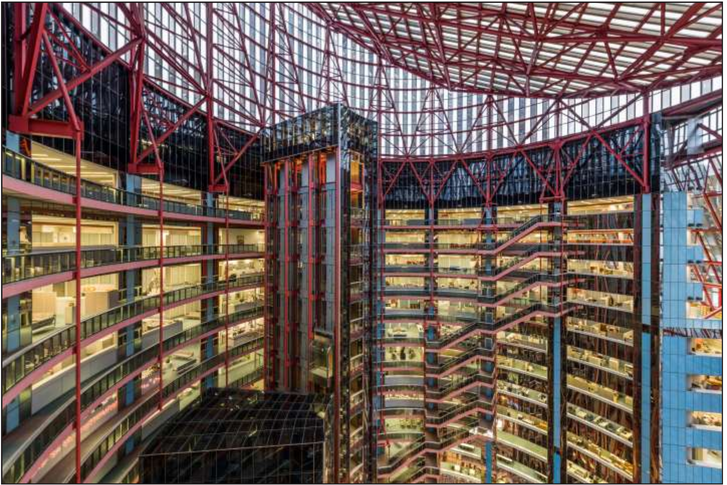
Upper floors, offices, elevator towers, and skylight of Thompson Center atrium © Serhii Chrucky
