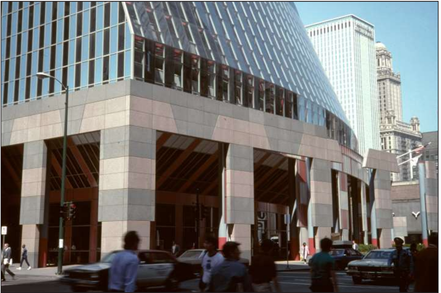
Original granite cladding and deconstructivist plinths at Thompson Center c. 1985 © C. William Brubaker, photographer. bruo03_05_gF, C. William Brubaker digital image collection, Special Collections and University Archives, University of Illinois at Chicago
