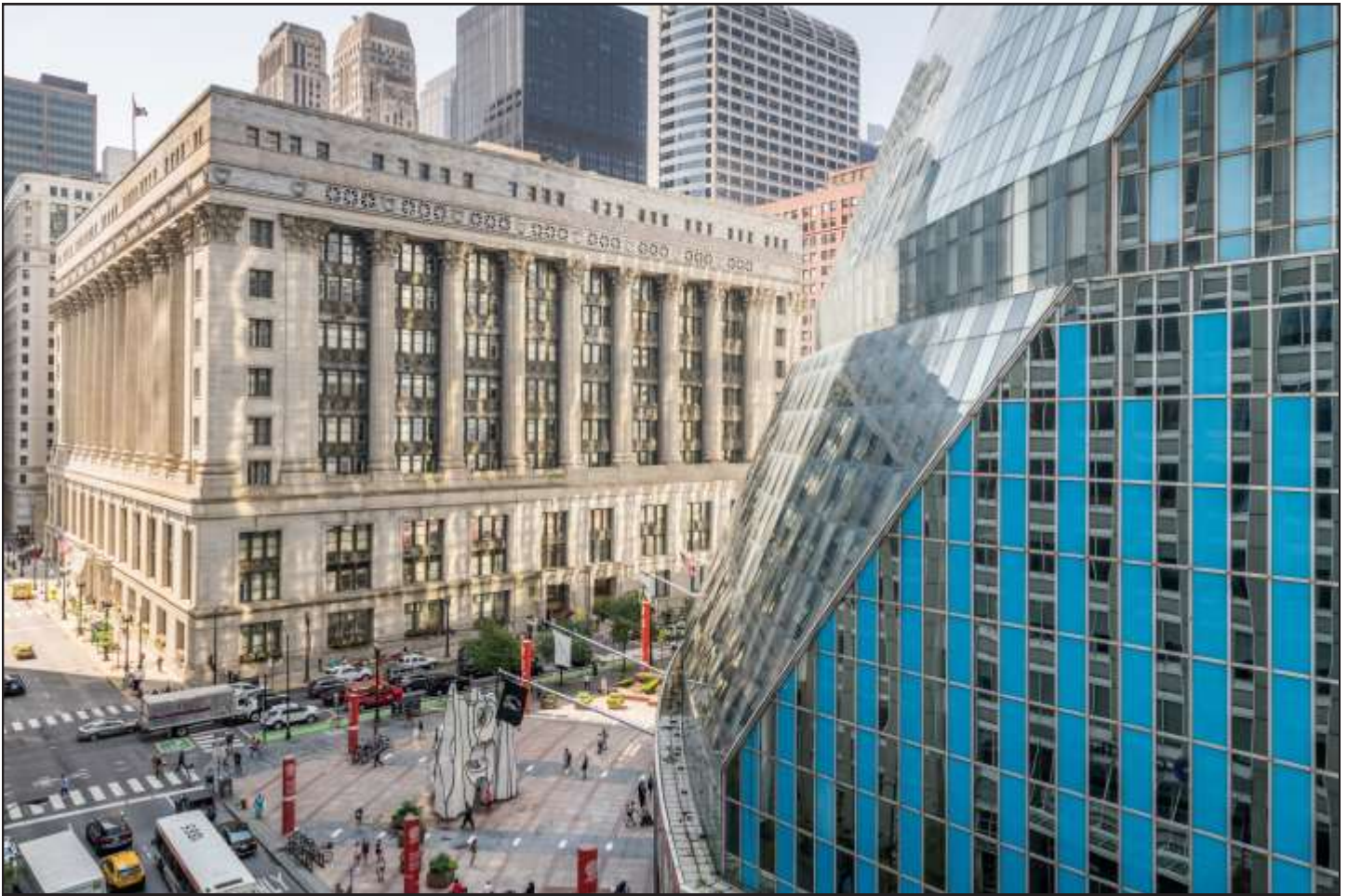
Chicago City Hall/Cook County Building across from the Thompson Center and Plaza with sculpture by Jean Dubuffet. © Serhii Chrucky
