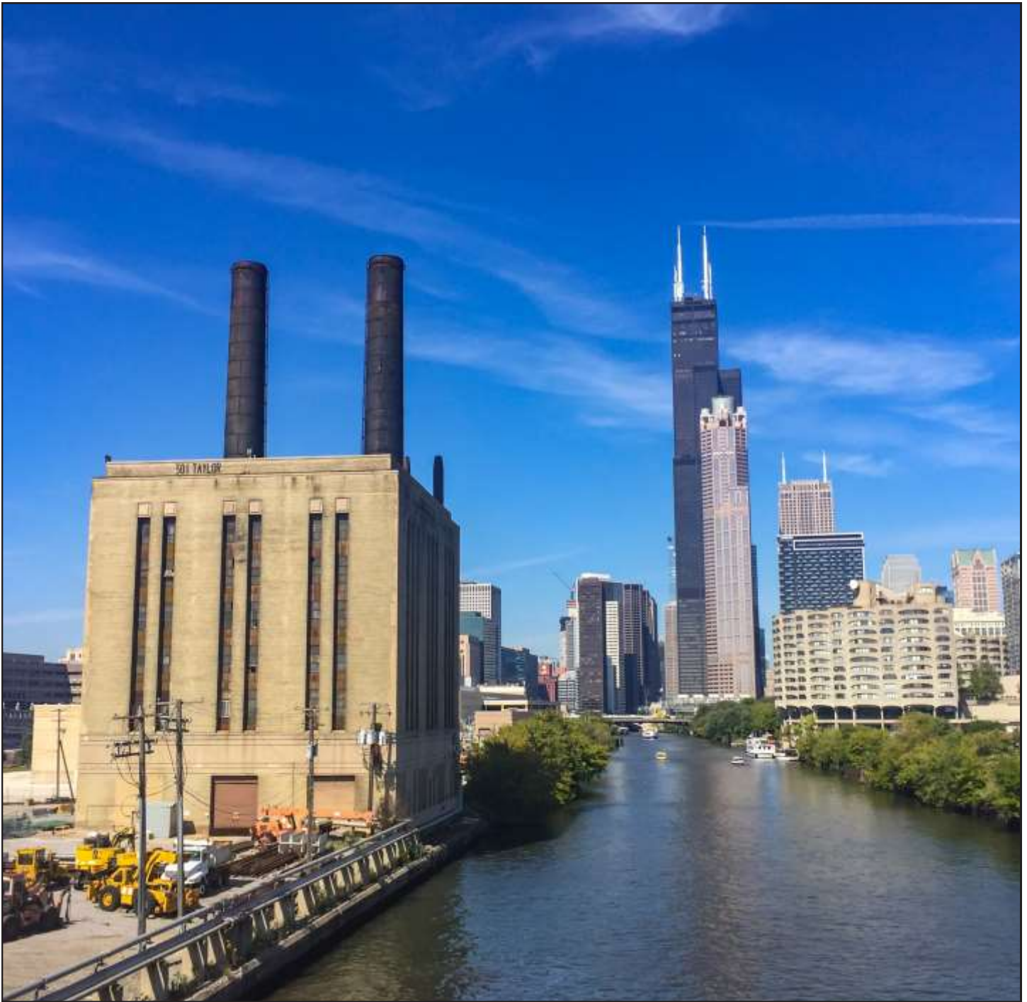
Looking northward at Chicago Union Station Power House with Chicago Loop in the distance © Eric Allix Rogers
