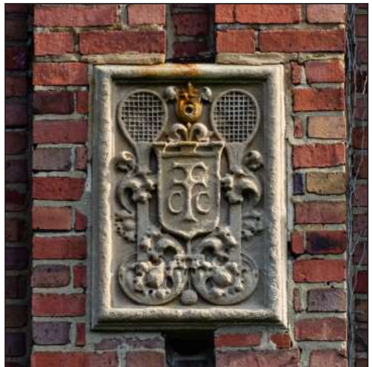
Chimney Detail on the Chicago Town & Tennis Club © Eric Allix Rogers
