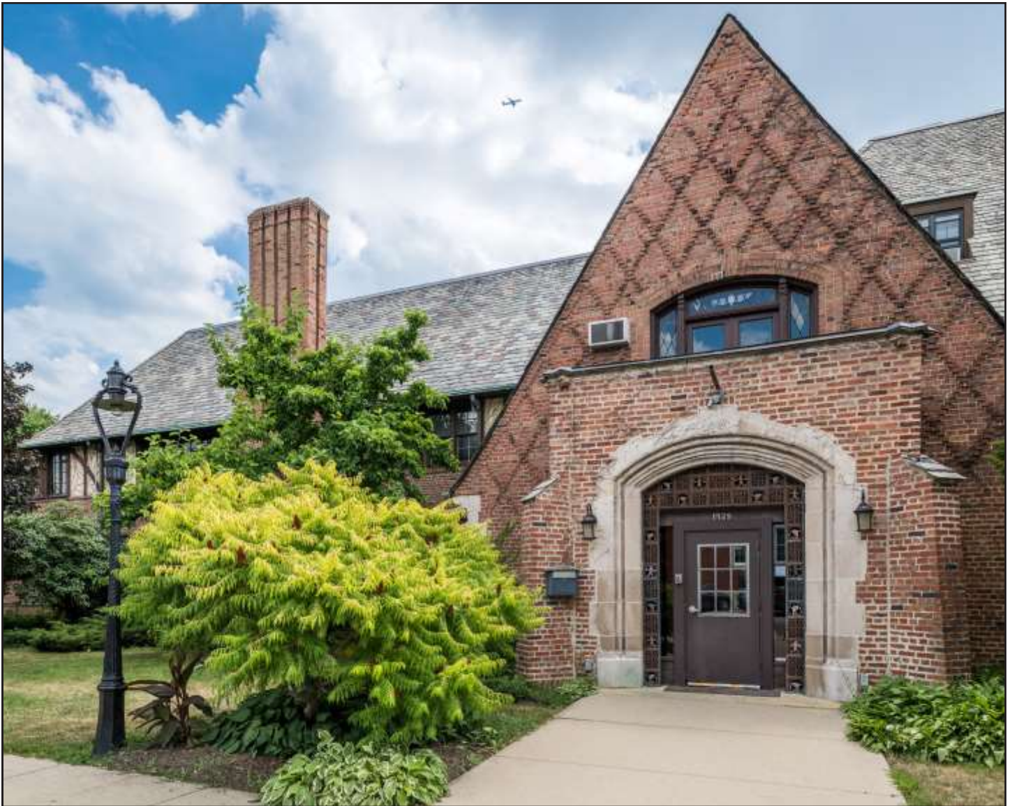
Main Entrance on North Elevation to the Chicago Town & Tennis Club / Unity Church © Serhii Chrucky
