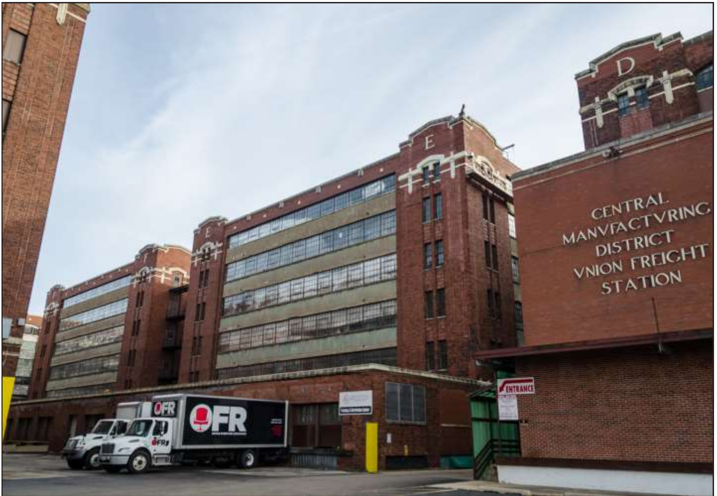
North elevation of interior buildings in central courtyard with CMD Freight Station. Central Manufacturing District - Pershing Road © Eric Allix Rogers
