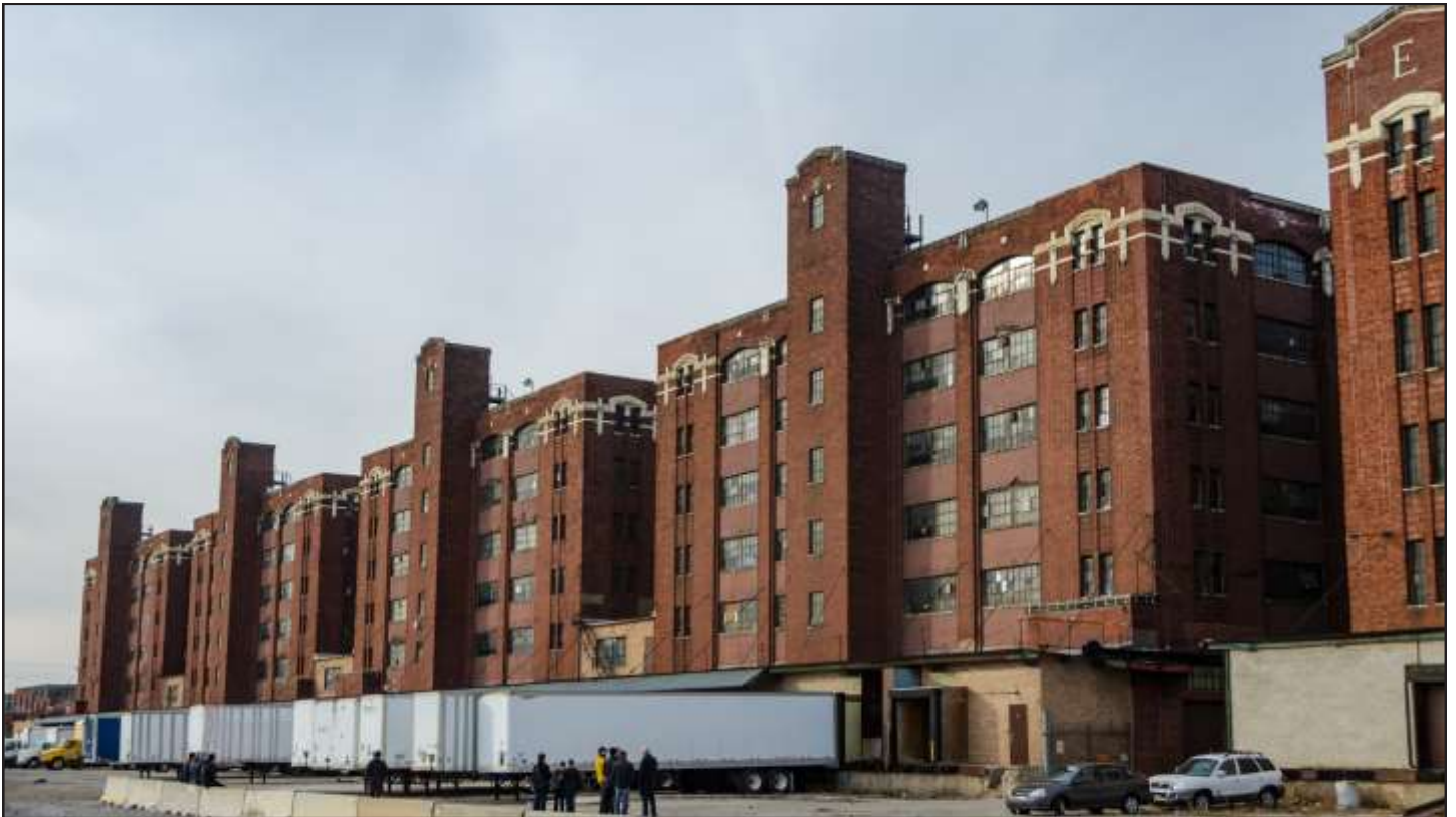
South facades (rear) and loading docks of interior buildings, Central Manufacturing District - Pershing Road © Eric Allix Rogers
