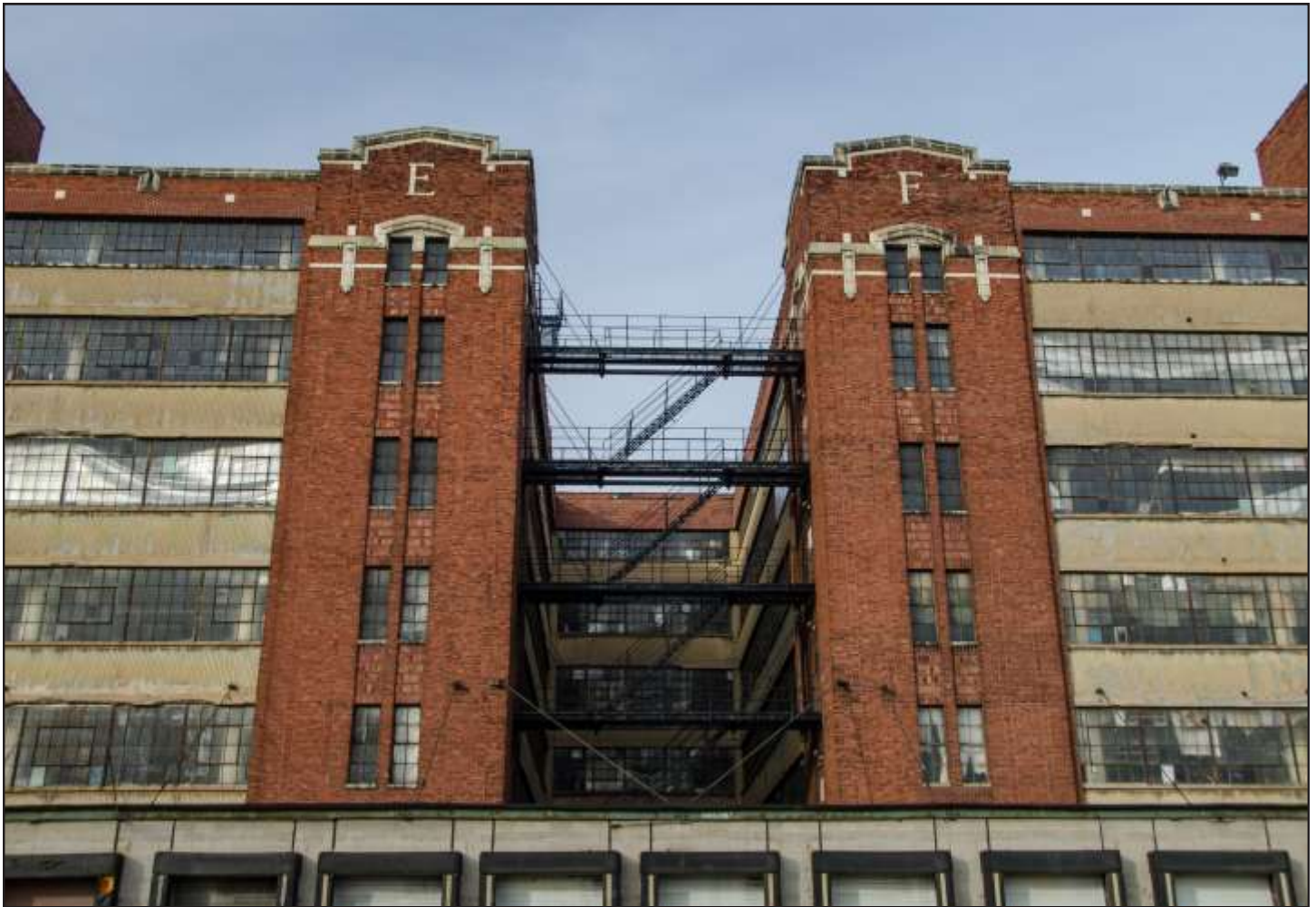
Southern façade (rear) of interior buildings with interconnecting structures, Central Manufacturing District - Pershing Road © Eric Allix Rogers
