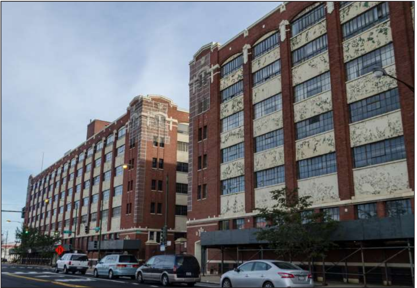
North elevation of buildings fronting Pershing Road, Central Manufacturing District - Pershing Road © Eric Allix Rogers
