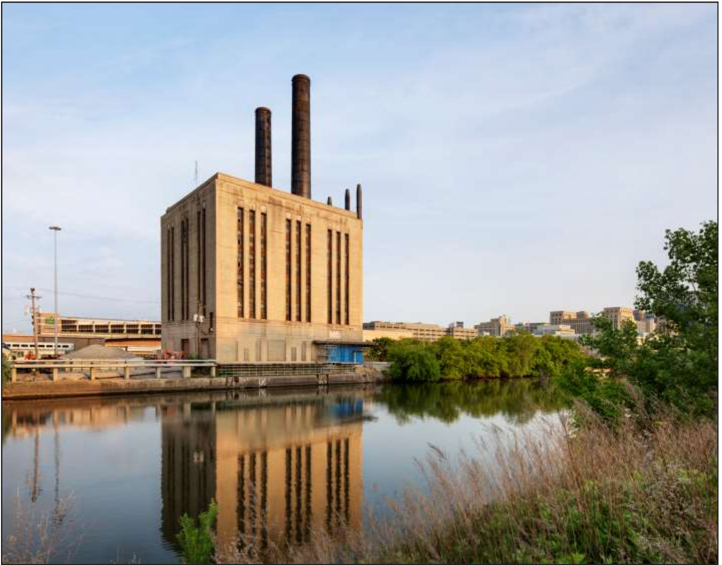
Chicago Union Station Power House across the Chicago River © Darris Lee Harris
