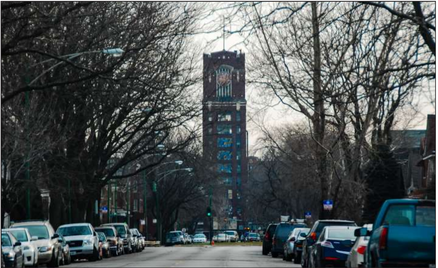
CMD Clock Tower building from Damen Avenue looking south, Central Manufacturing District - Pershing Road © Eric Allix Rogers
