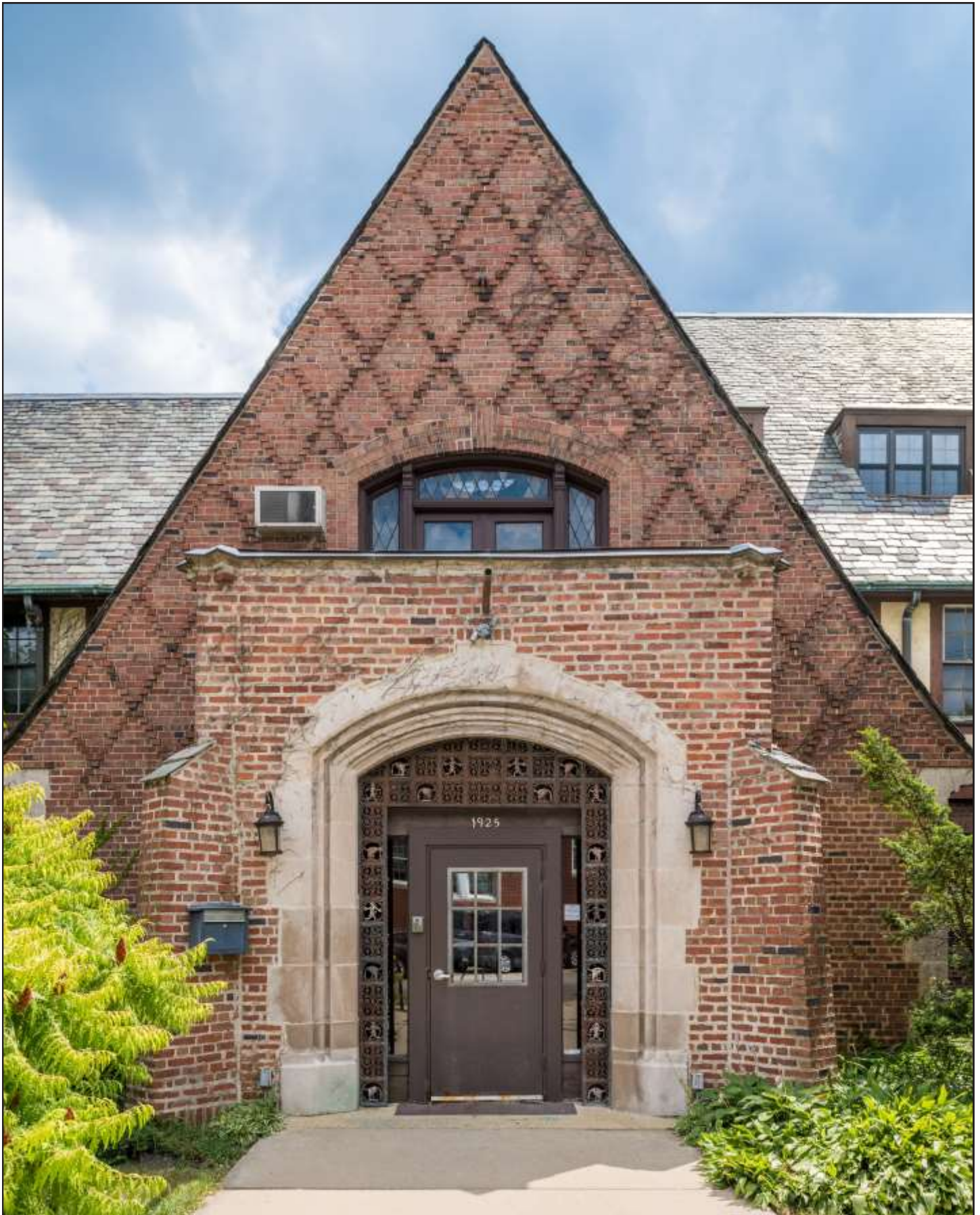
Main Entrance on Thome Avenue of the Chicago Town & Tennis Club / Unity Church © Serhii Chucky
