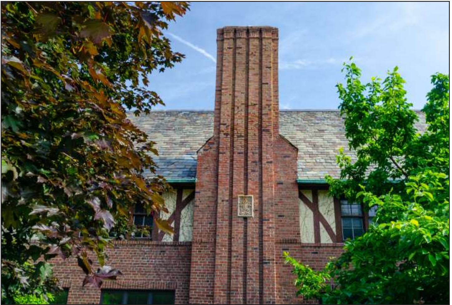
Chimney detail on the north elevation of Chicago Town & Tennis Club / Unity Church © Eric Allix Rogers
