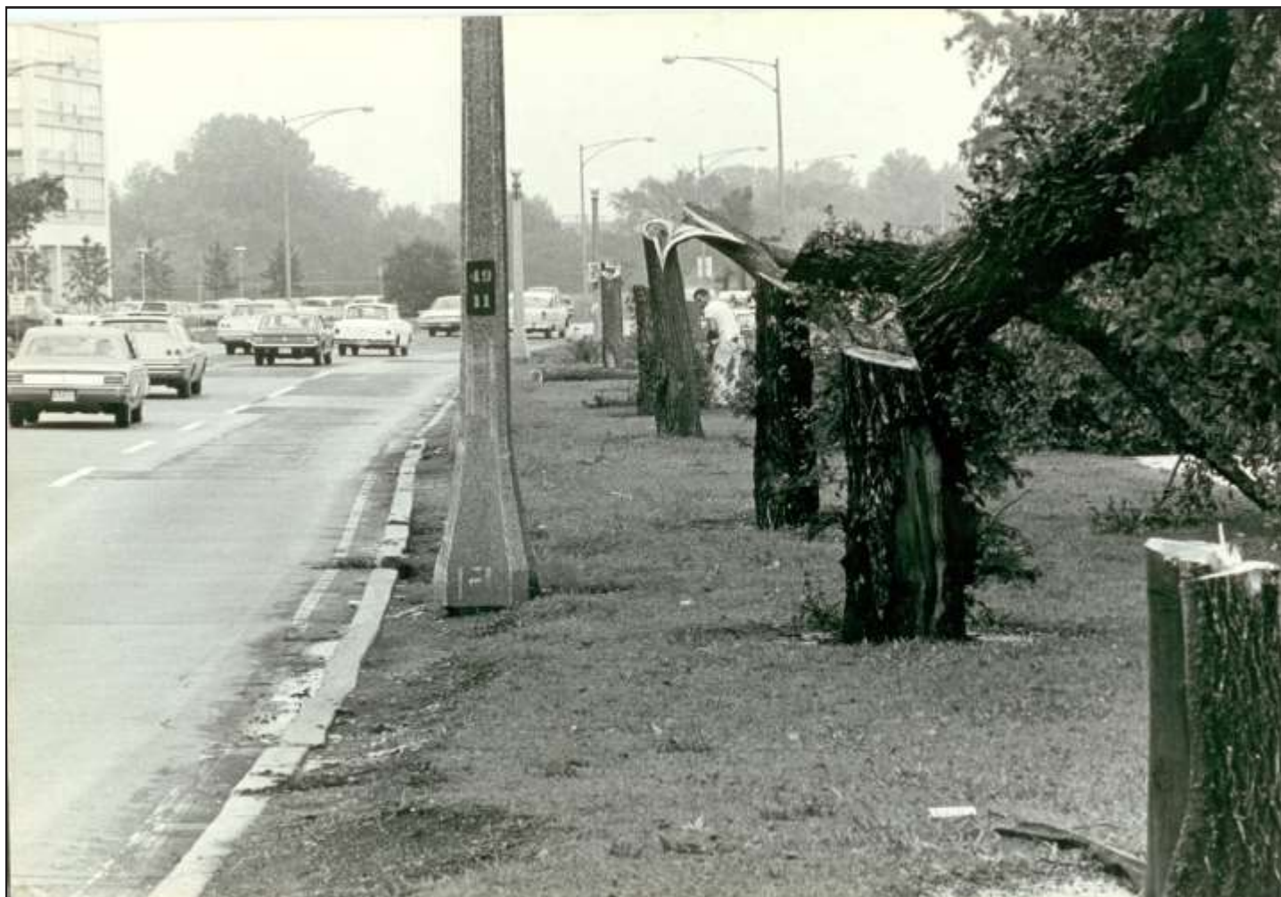
Tree cut and removal on the Lakefront in Hyde Park for the widening of South Lake Shore Drive in September 1965 © Nancy Hays
