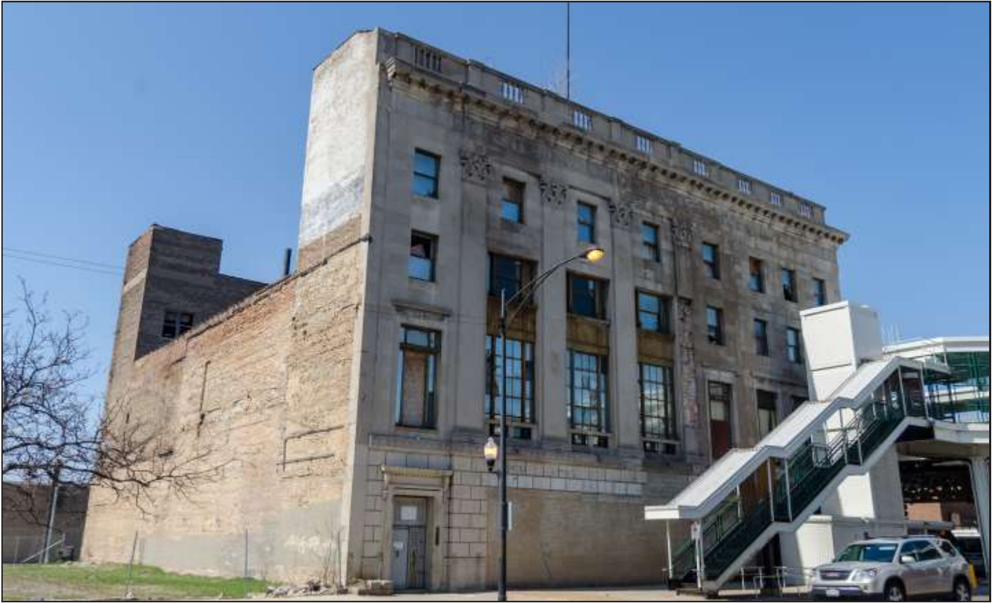
Existing Conditions of the Washington Park National Bank fronting Cottage Grove Avenue © Eric Allix Rogers
