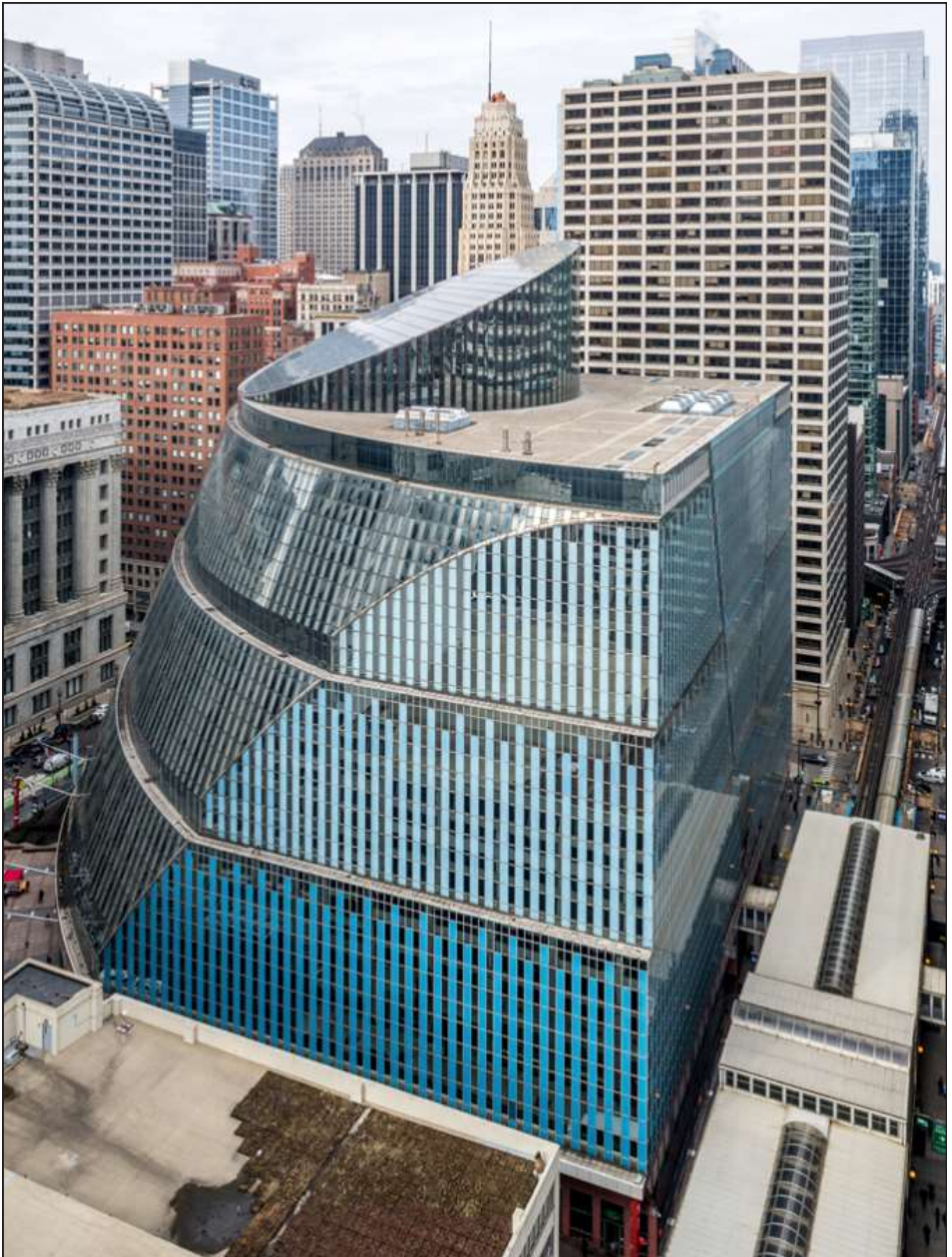
Aerial views of the Thompson Center's Clark and Randolph Street elevations with projecting skylight © Serhii Chruky
