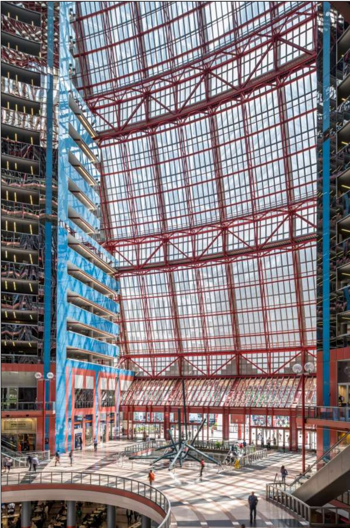
Thompson Center's glass curtain wall structure at principal entryway with view into lower concourse level © Serhii Chucky
