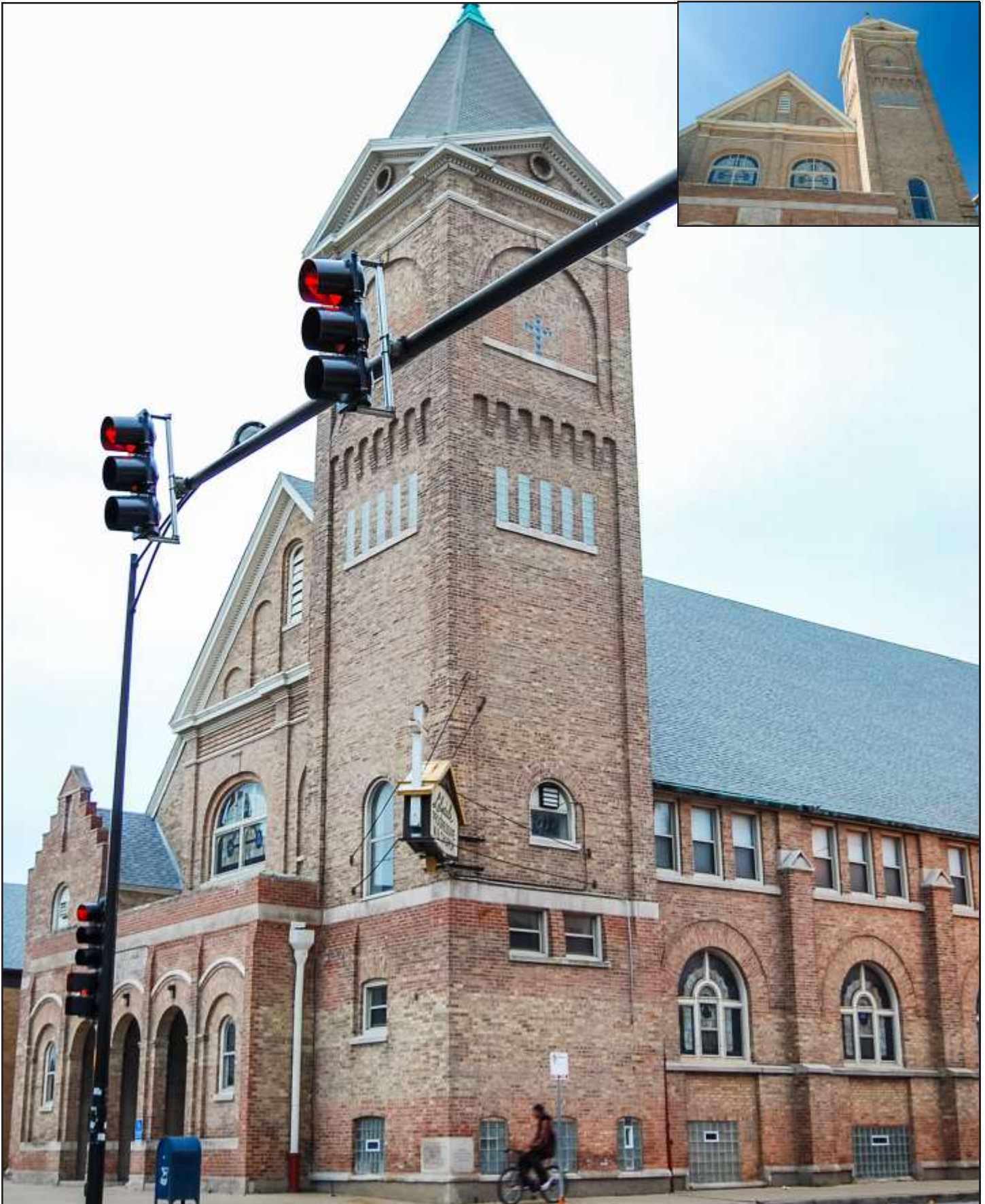
First Reform Church of Roseland, now known as Lilydale Progressive M.B., built in 1887 by Dutch settlers and abolitionists, at 107th Street and South Michigan Avenue in Roseland's Michigan Avenue Commercial District © Eric Allix Rogers
