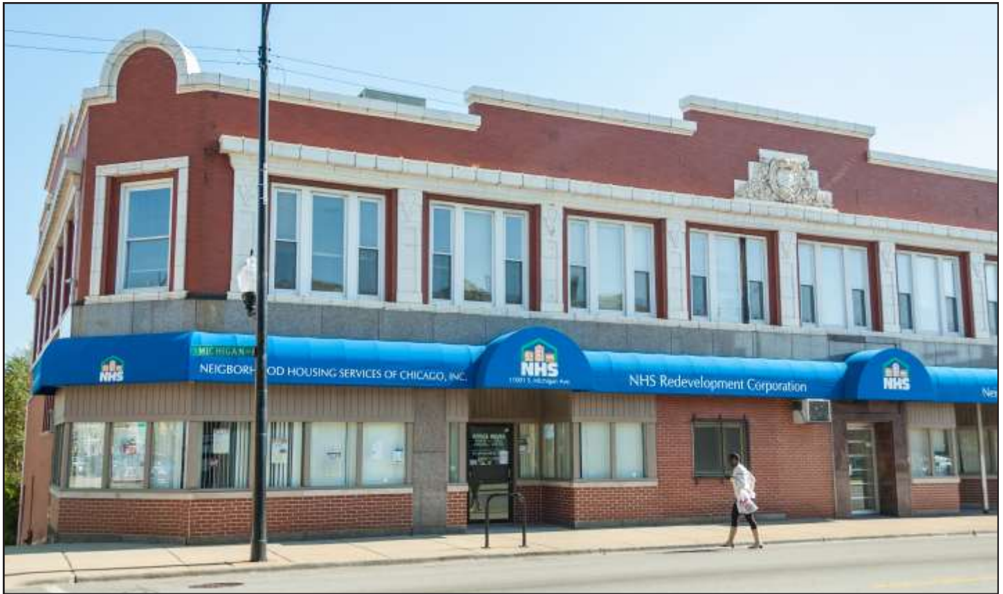
110th Street corner on Roseland's Michigan Avenue Commercial District © Eric Allix Rogers
