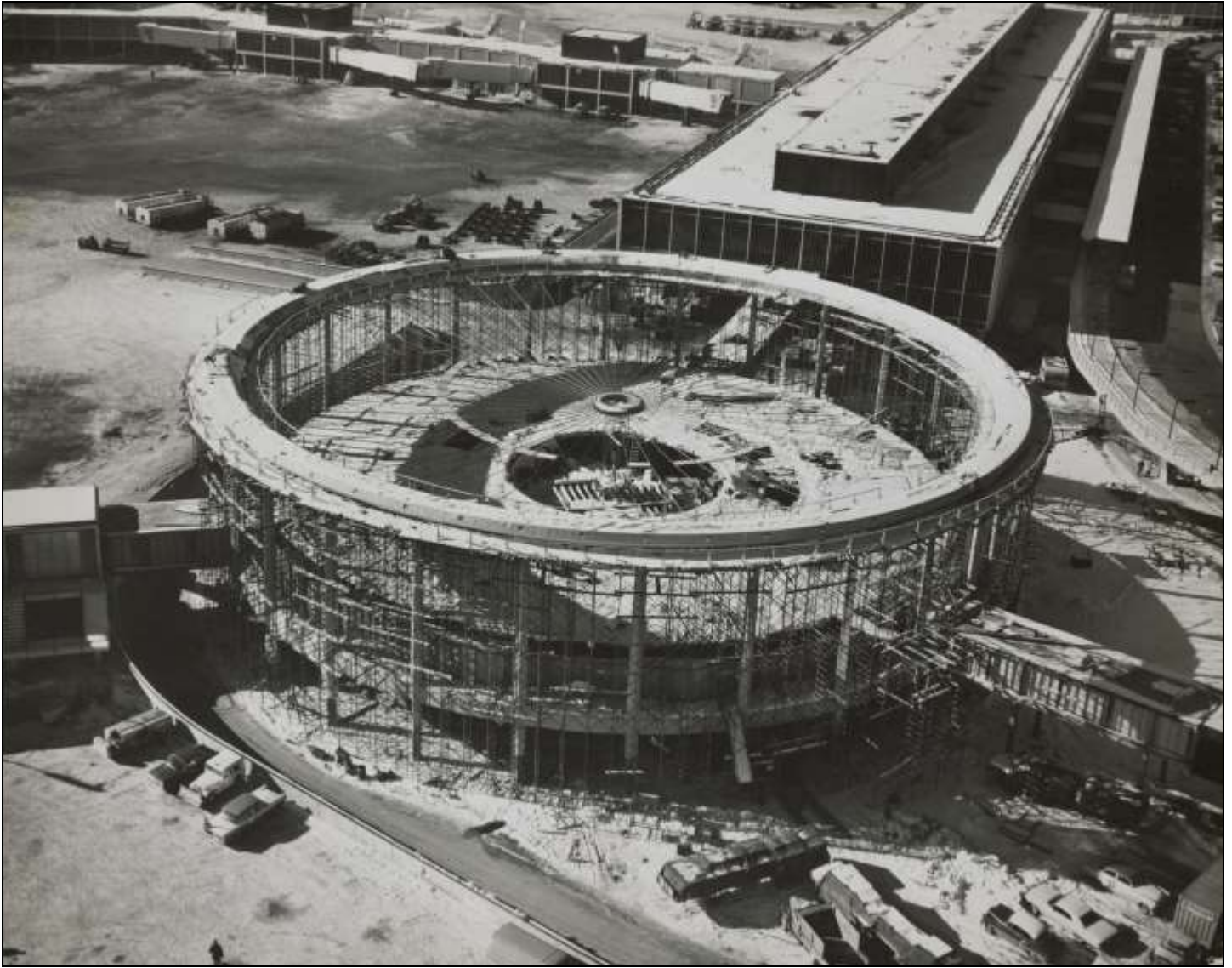
Seven Continents Building / O'Hare Rotunda Building, construction aerial view. Chicago Aerial Survey Co., photographer, Courtesy Gertrude Lempp Kerbis Archive, Ryerson and Burnham Archives, The Art Institute of Chicago
