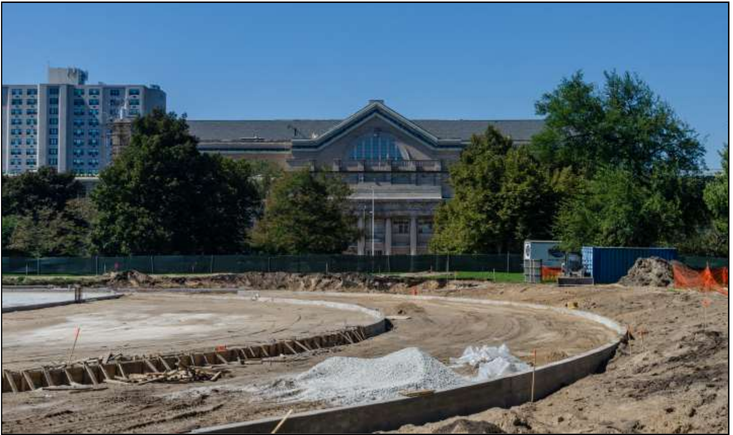
Track under construction adjacent to proposed Obama Presidential Center in Jackson Park © Eric Allix Rogers
