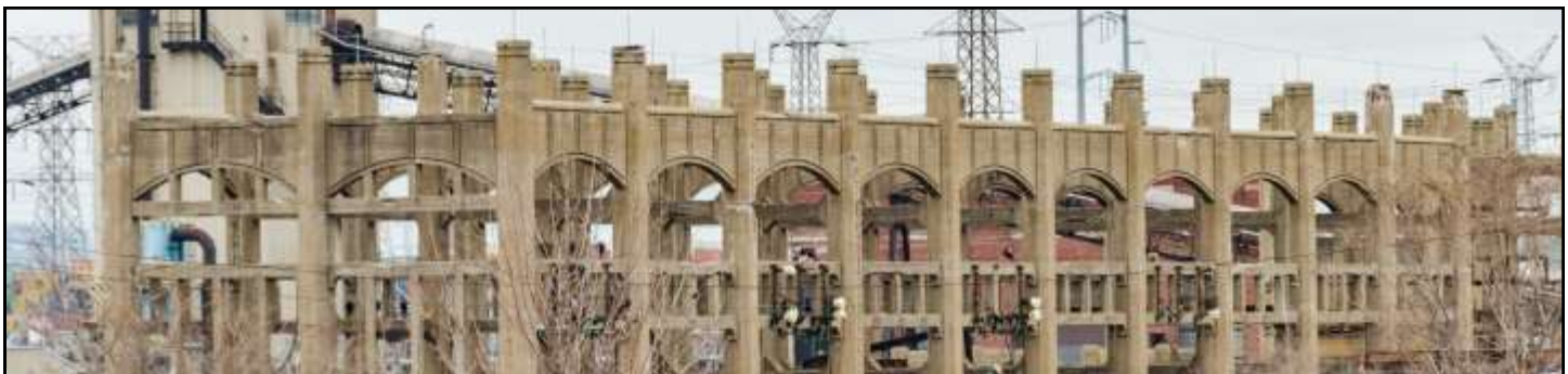
Crawford Power Station © Eric Allix Rogers
