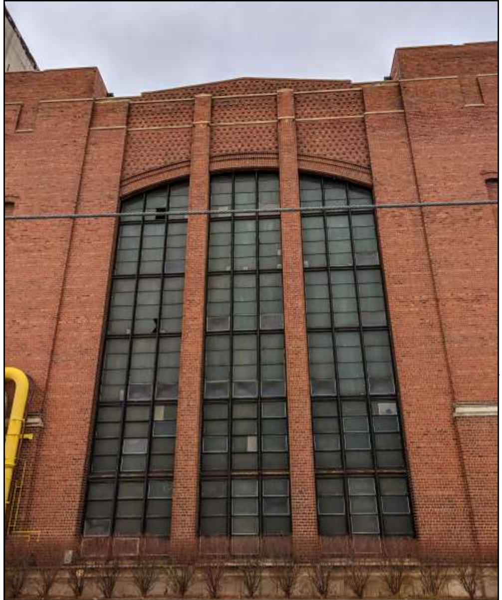
Crawford Power Station © Eric Allix Rogers
