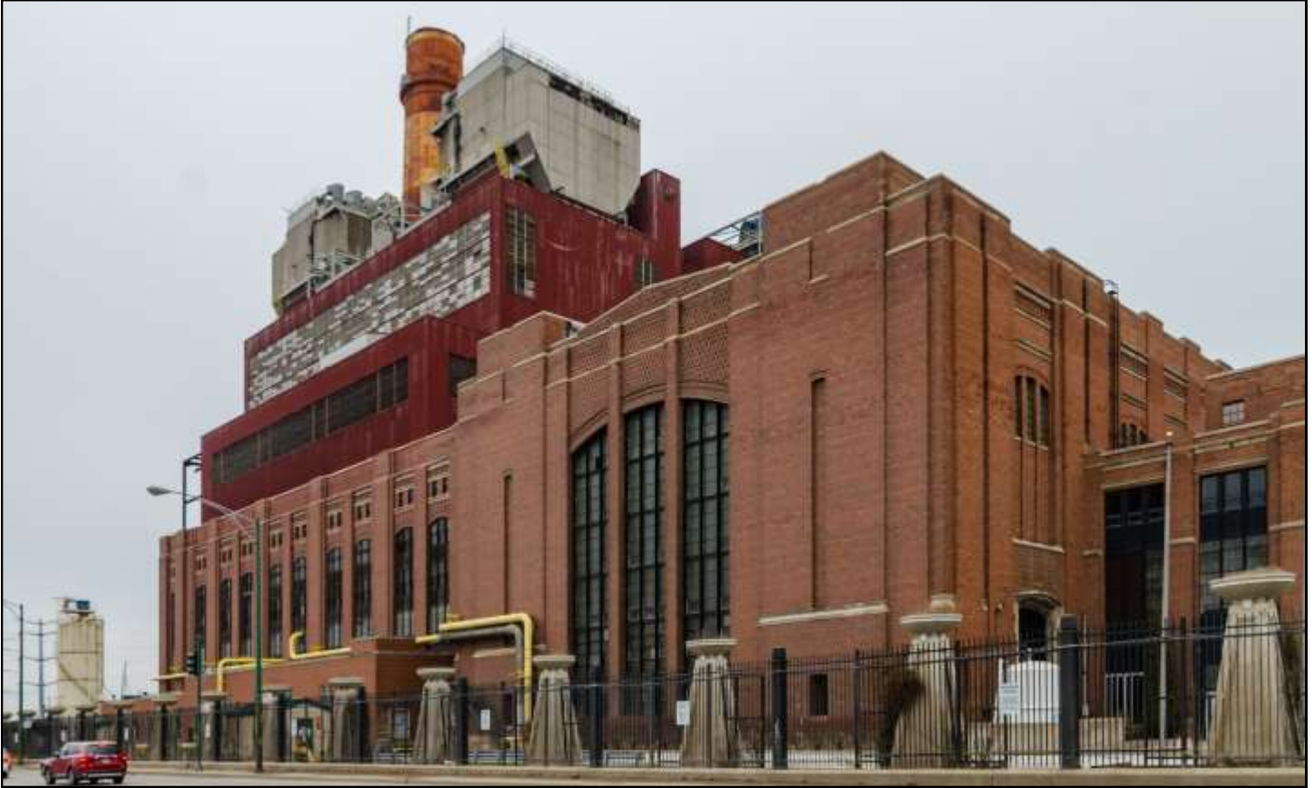
Crawford Power Station © Eric Allix Rogers
