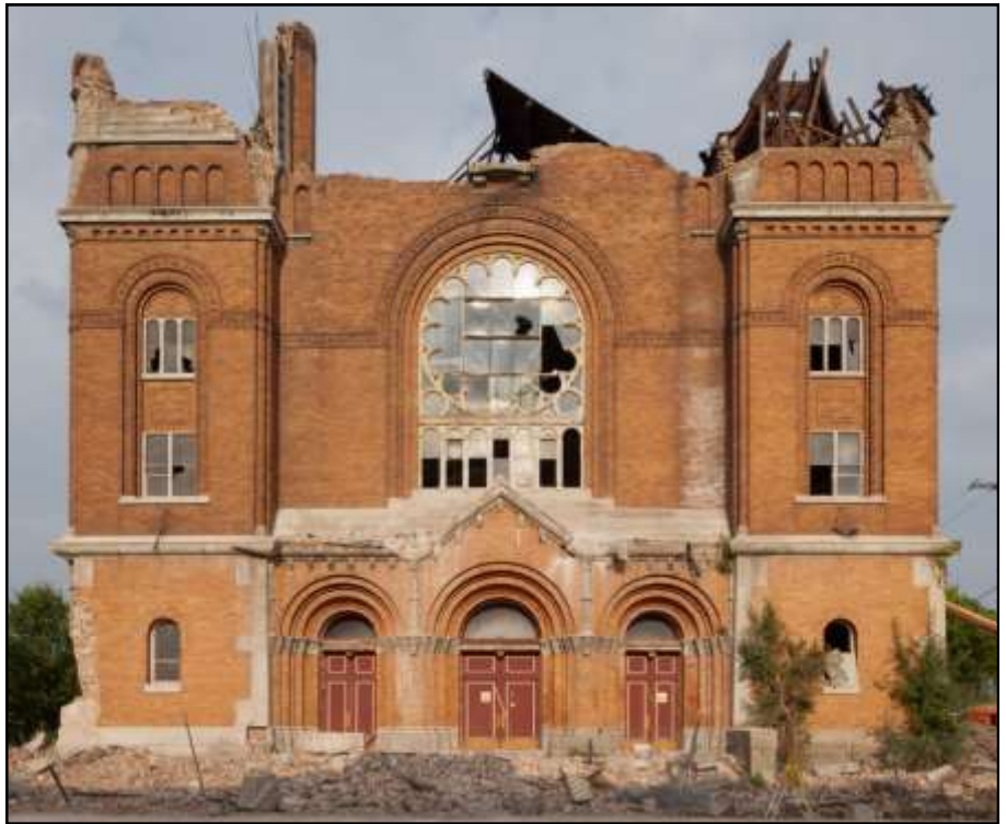
St. Laurence Catholic Church during demolition 2014 © Noah Vaughn
