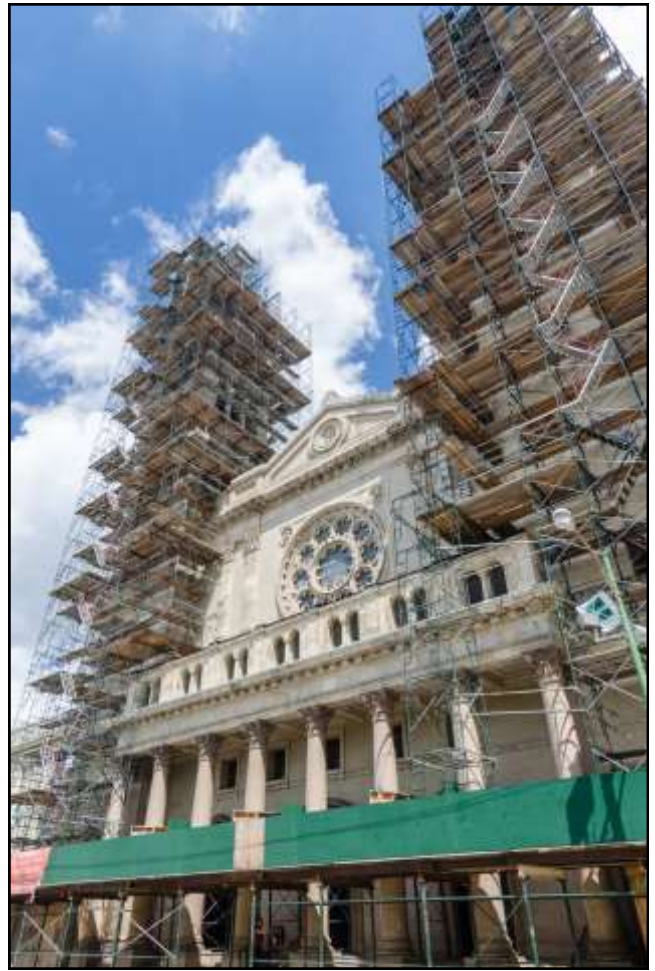
St. Adalbert with and without scaffolding © Eric Allix Rogers
