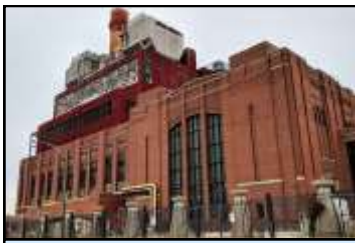
Crawford Power Station
