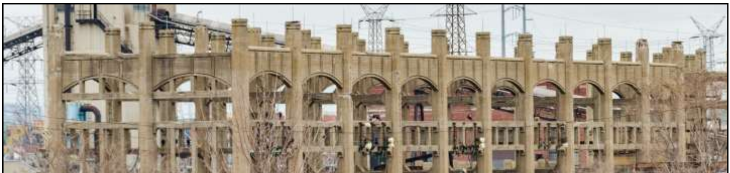
Crawford Power Station © Eric Allix Rogers
