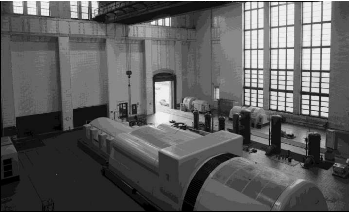
Crawford Power Station Turbine Hall Interior View © Library of Congress
