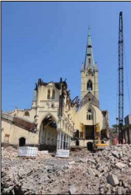
'Old' St. James Catholic Church during demolition 2013 © Gabriel X. Michael
