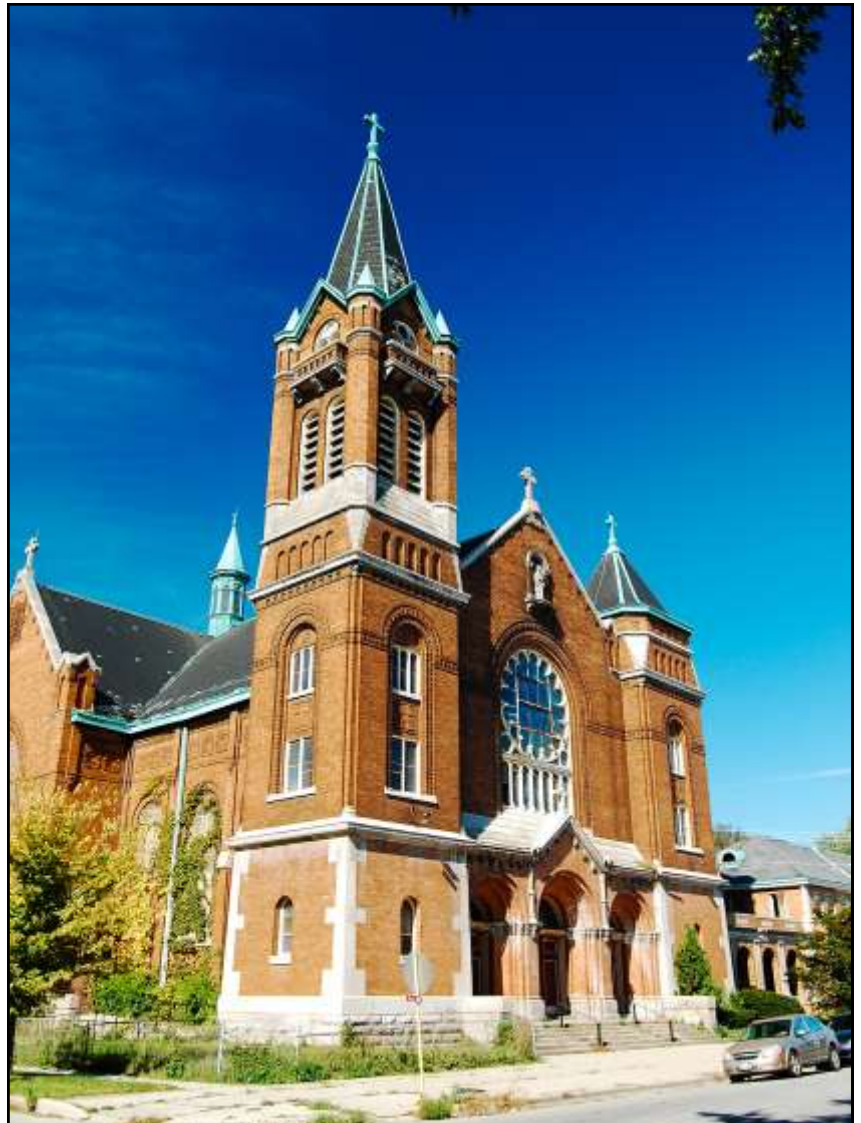
St. Laurence Catholic Church prior to demolition © Eric Allix Rogers
