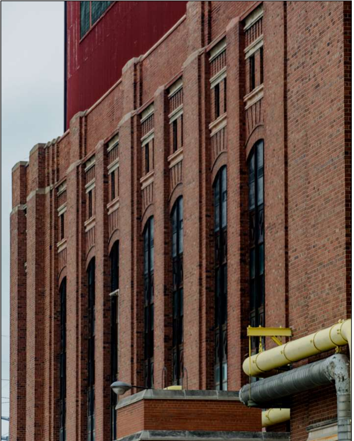
Crawford Power Station © Eric Allix Rogers
