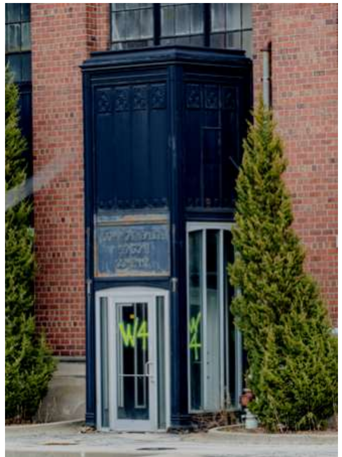
Crawford Power Station © Eric Allix Rogers
