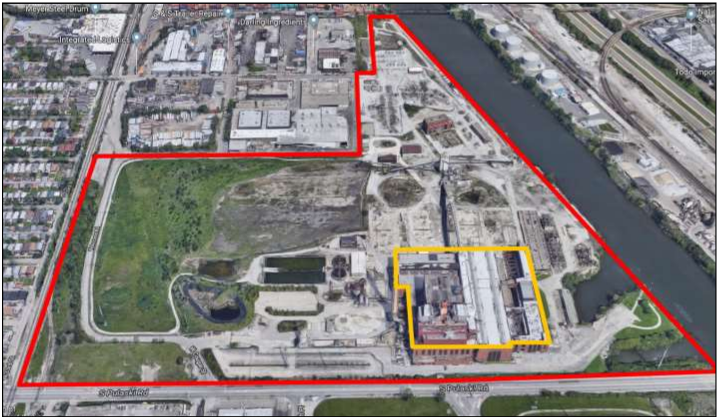
Historic Crawford Power Station outlined in yellow and extensive approximately 70 acre site outlined in red © Google Maps Aerials
